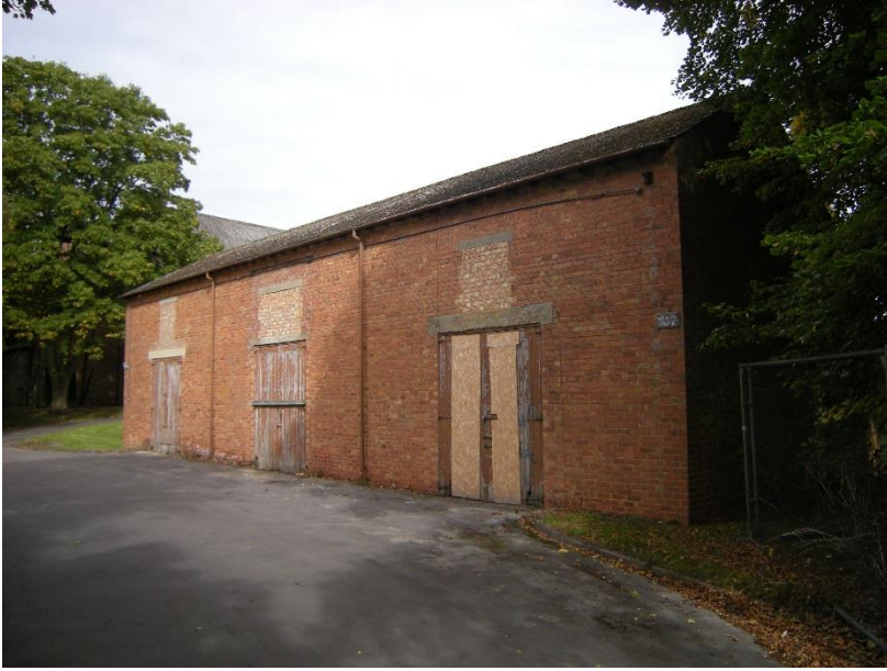
Fig 02 – Building 102 from South East
