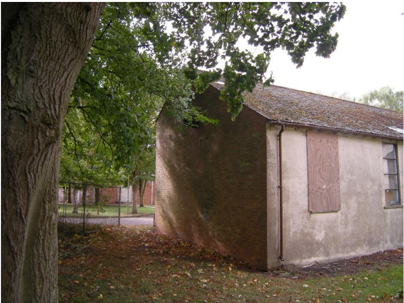
Fig 05 – Building 102 East Gable end
