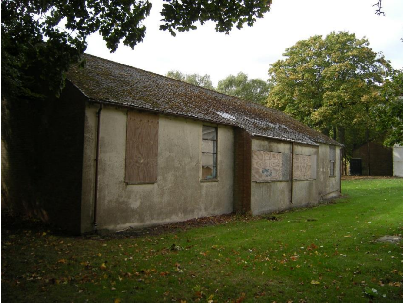
Fig 04 – Building 102 from North East
