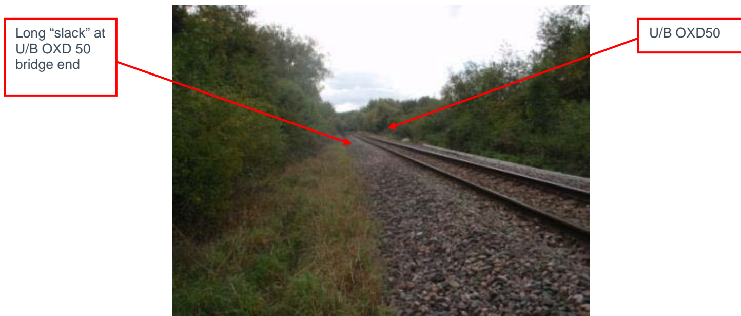
Photograph 2: OXD Line looking towards Oxford (Down Direction)
