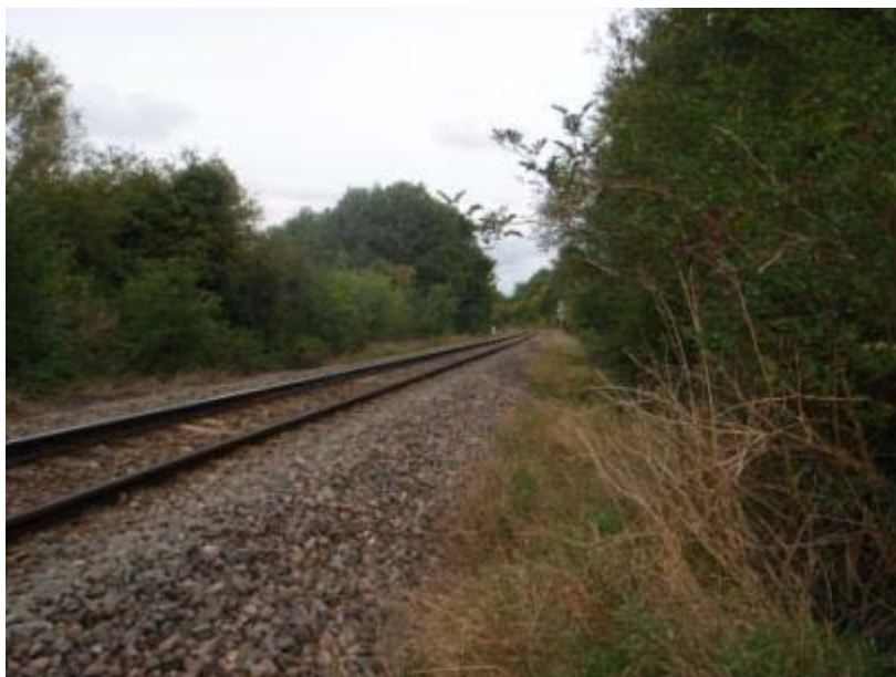
Photograph 1: OXD Line looking towards Islip (Up direction)
