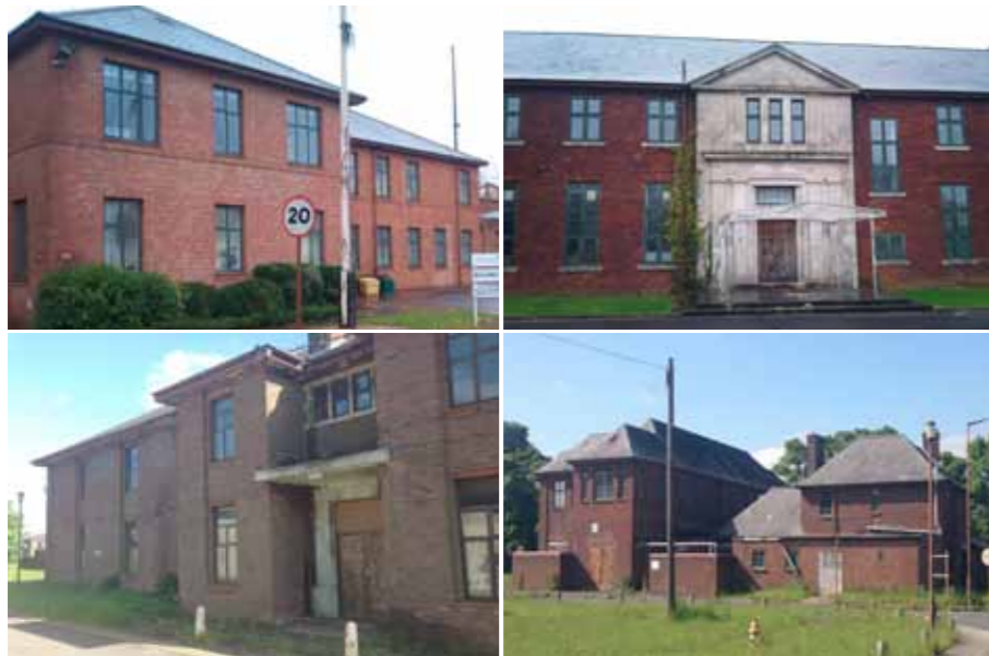
EXISTING FACILITIES AND BARRACKS BUILDINGS TO PROVIDE DESIGN PRECEDENT FOR THIS AREA
