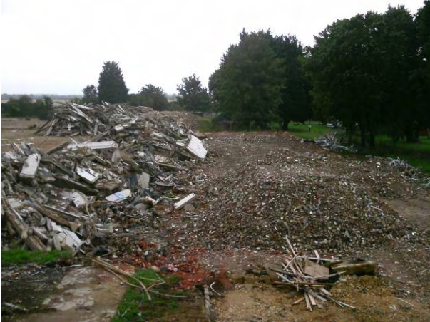
26.06.14 Demolition material awaiting processing from buildings 594 and 598
