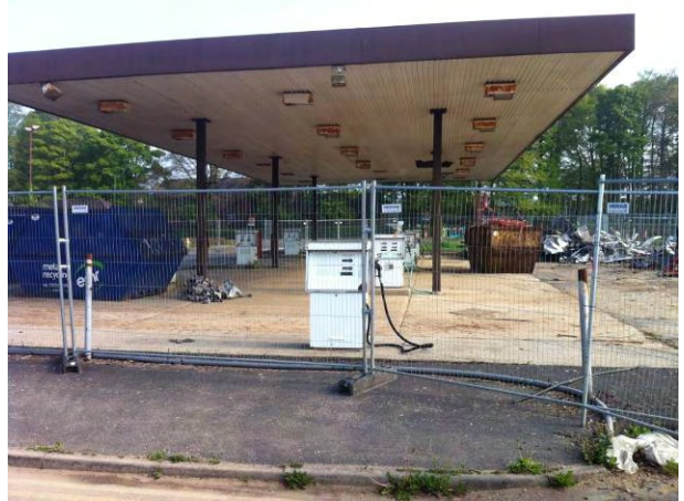
30.04.14 Petrol forecourt located in the north of D1B: Area 2 (building 493); location of UG-NSA-16-20
