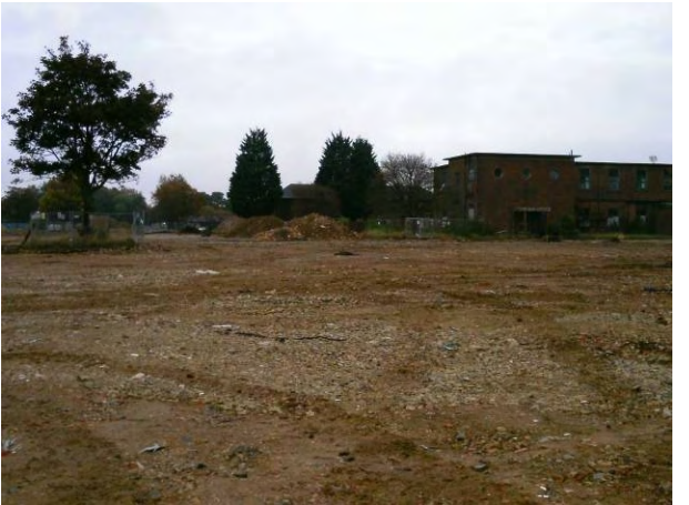
07.10.14 Temporary stockpiles of hydrocarbon waste generated from UST remediation temporarily stockpile (background)
