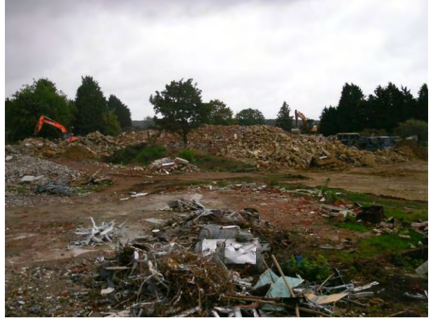
26.06.14 Processing of site won aggregates in the south of the site
