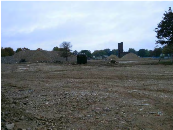
07.10.14 Northern view along the western side of the site, exposed natural strata following hard-standing strip
