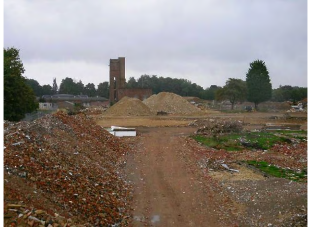
26.06.14 Northern view along the site's western boundary
