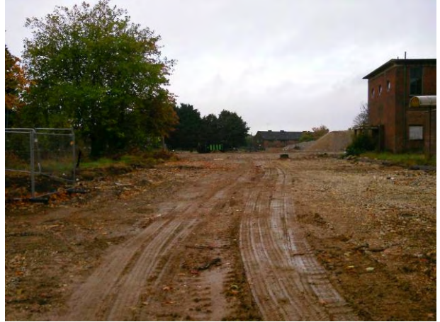
07.10.14 Western view across the southern face of retained building 488
