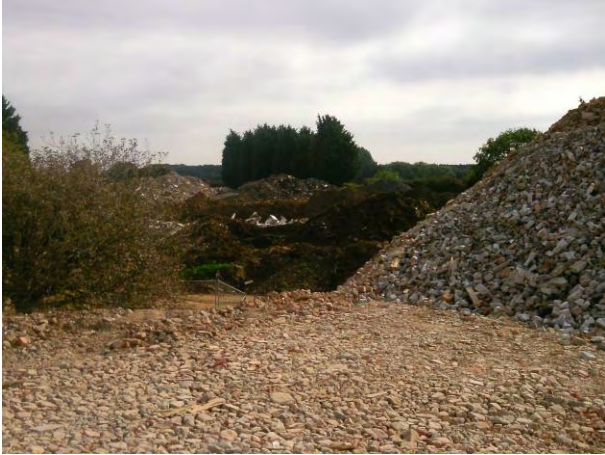
10.09.14 Eastern view along the south of the site, stockpile storage area
