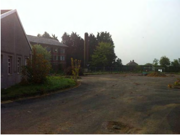
30.04.14 Chimney associated with boiler house (building 441); location of UG-NSA- 5-7
