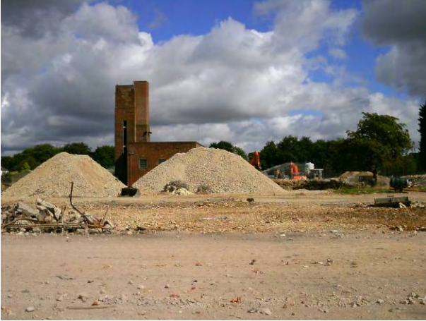
19.08.14 North-west corner of the site, boiler house (building 457) visible behind aggregate stockpile Agg-NW
