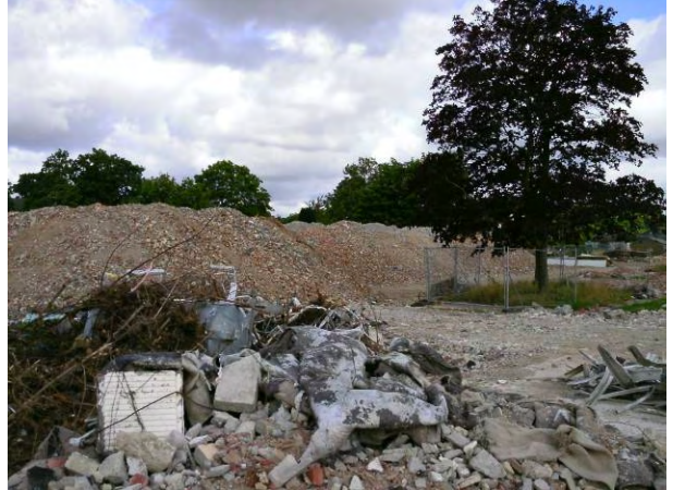
19.08.14 Site processed aggregate stockpile along the site's western boundary (Agg-W)
