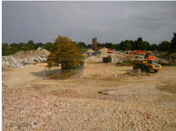
10.09.14 Northern view across the site with processing of hard-standing taking place
