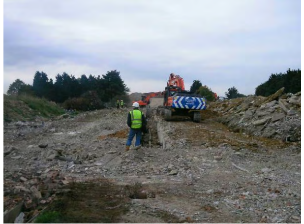
10.09.14 Breaking out of relict drains in the south-west of the site
