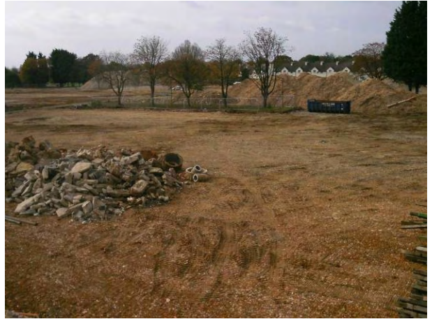
22.10.14 – Central view of the site, natural soils exposed following strip of hard-standing
