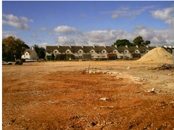
24.09.14 Remediation earthworks completed in the north-west corner
