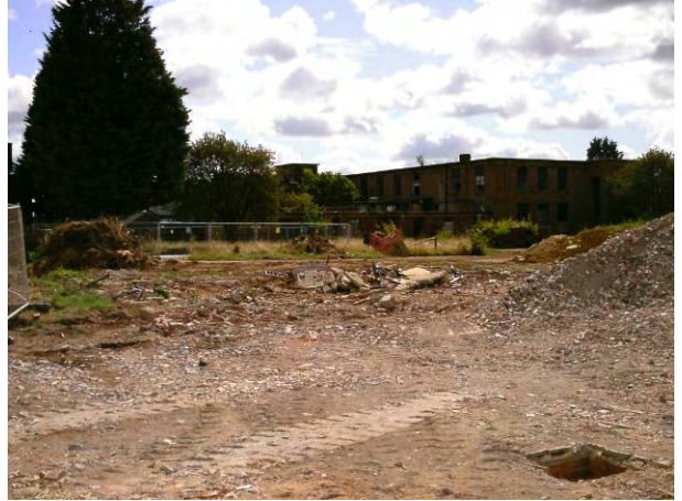
19.08.14 Centre of the site with building 498 that is to remain as part of the redevelopment
