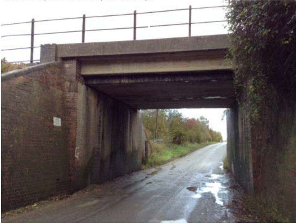
Photograph 15: Under Bridge 99, DCL 94m 77ch Western (Down cess) Elevation
