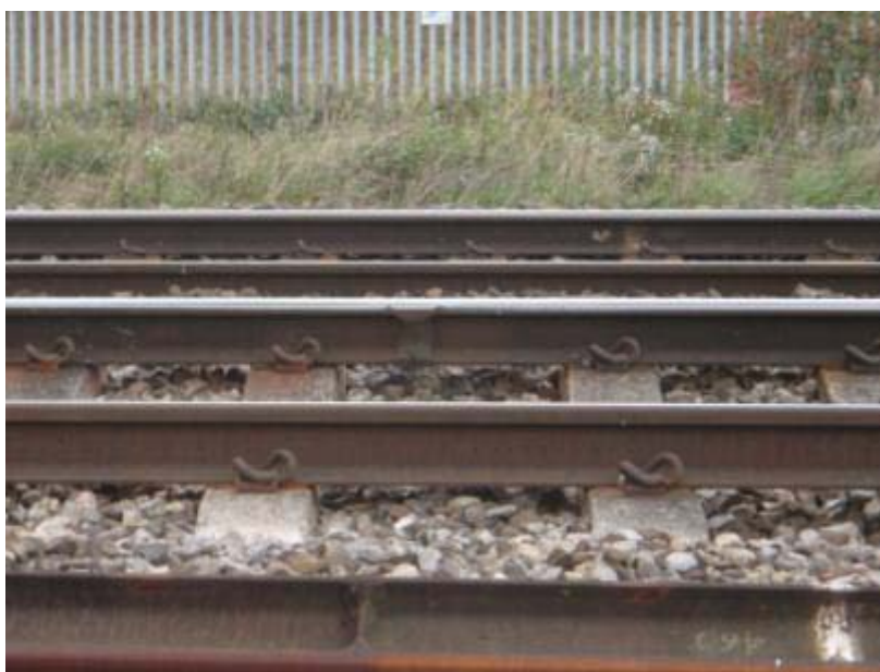
Photograph 11: DCL Line Up Main 6' rail 65m 501yards. L80 wide gap weld
