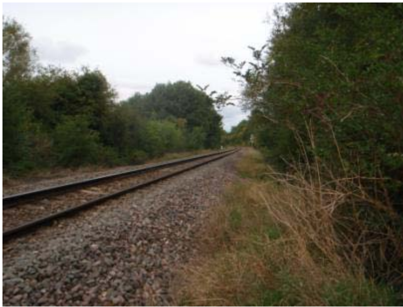
Photograph 1: OXD Line looking towards Islip (Up direction)
