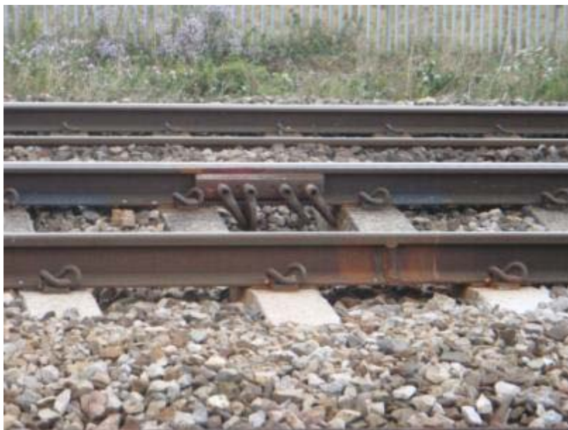
Photograph 10: DCL Line Up Main 6' rail 65m 515yards. Thermit Weld Emergency clamped
