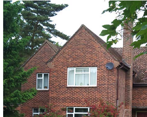
C4 GABLE FRONTED WITH CORBEL DETAILS
