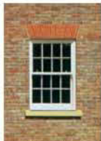
Example illustration - Flat gauged arch and stone window sill
