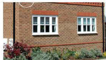
Example illustration - Projecting string course brickwork
