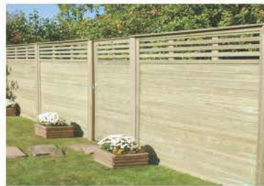
Timber fencing to garden facing access lanes
