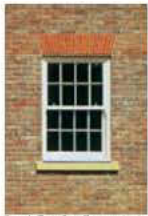
Example Illustration - Flat gugged arch and stone window
