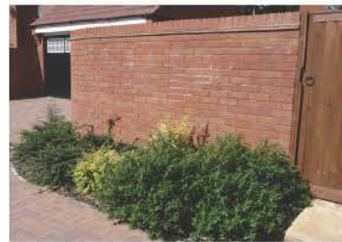
Brick wall to eastern end of courtyard
