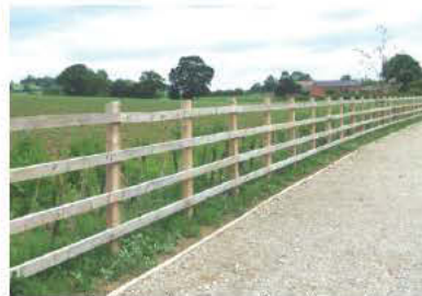
Post and rail fencing to southern boundary
