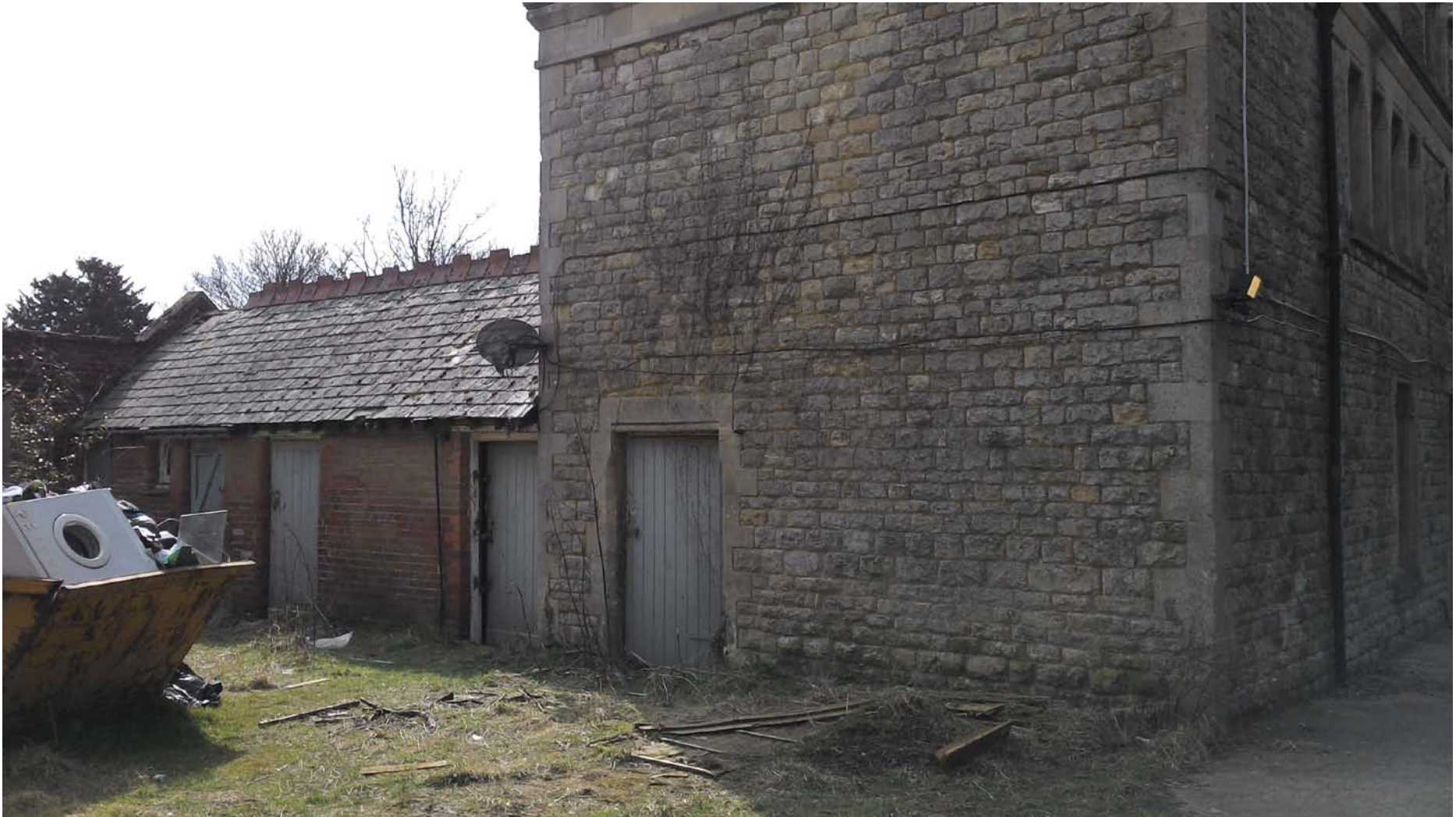
Northeast Elevation [please see Elevational Drawings included with the application for details of outbuilding conversion]
