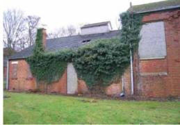
Building 82 - Holed roof, water damage, vegetation - Building of local importance
