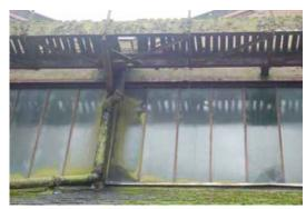
Building 137 - Failure of rainwater goods, water penetration - Grade II Listed
