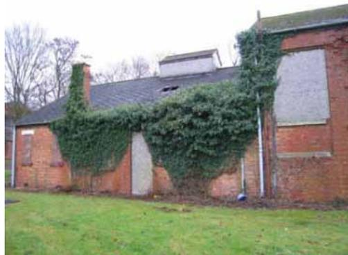
Building 82 - Holed roof, water damage, vegetation - Building of local importance
