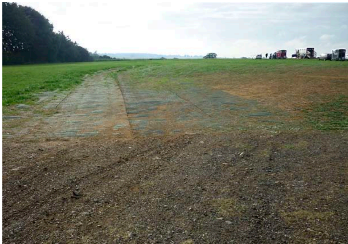
Ground reinforcement to reduce traffic wear on 28 Day Field.
