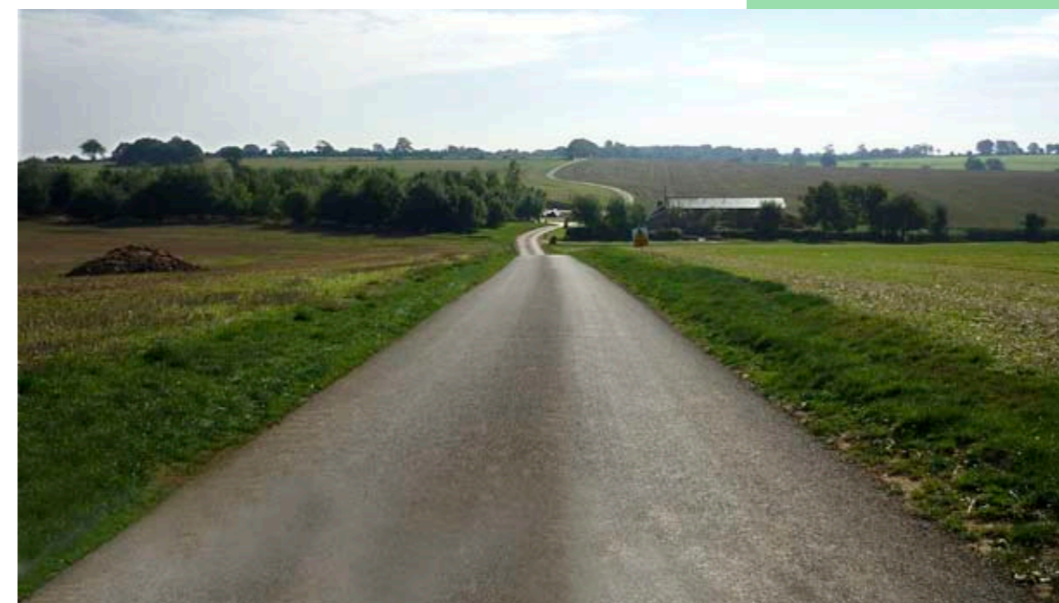
Grange Lane, 2.5m wide with one passing bay serving 2.15 kilometres of single track lane.
