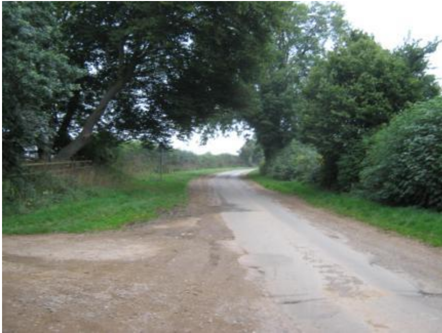
View of the damage in Grange Lane
