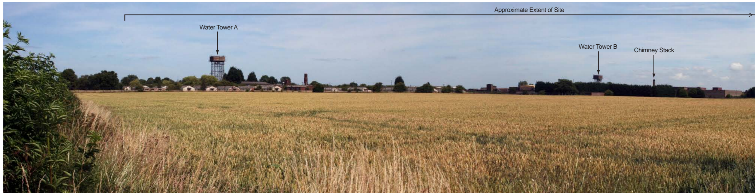
Photoviewpoint 10: View from Kirtlington Road looking east toward the site. The school and recreational sections of the RAF base are visible in the middle ground of the view although other sections tend to merge within the existing vegetation. The water towers act as prominent landmarks for the site.
