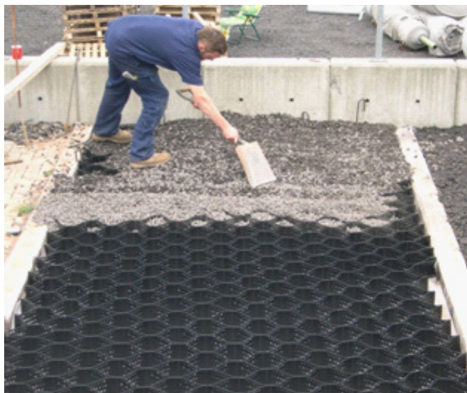
Figure 2 - CellWeb TRP® in construction.
