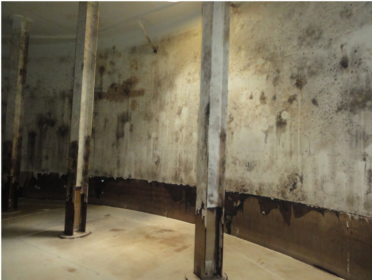
Photograph 250: POL 23B - Tank condition after clean and degas
