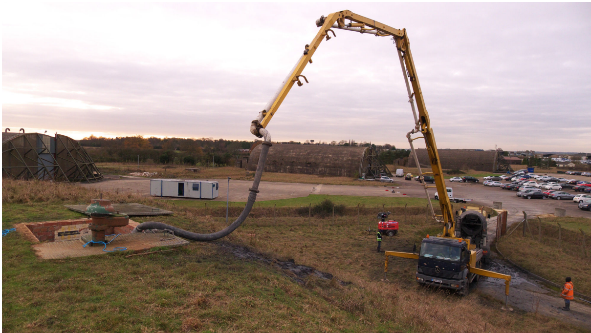
Photograph 388: Pump-over grout filling of Type 1 tank
