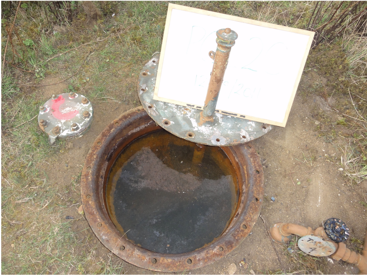
Photograph 13: POL 2C - Pre-condition photograph. Taken during tank sampling and inspection
