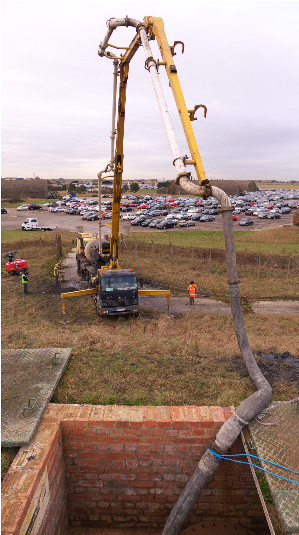
Photograph 389: Pump-over grout filling of Type 1 tank
