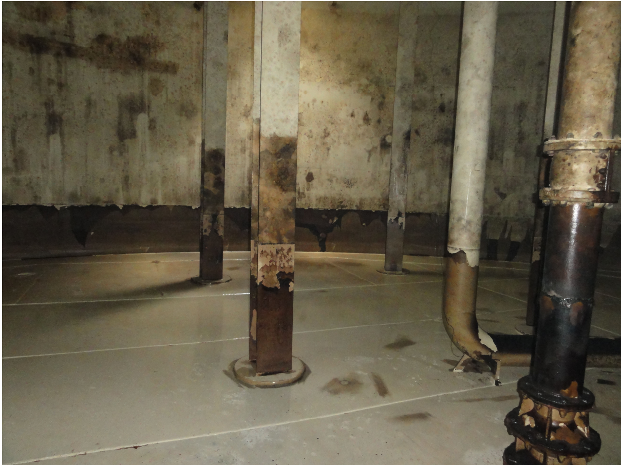
Photograph 246: POL 23B - Tank condition after clean and degas
