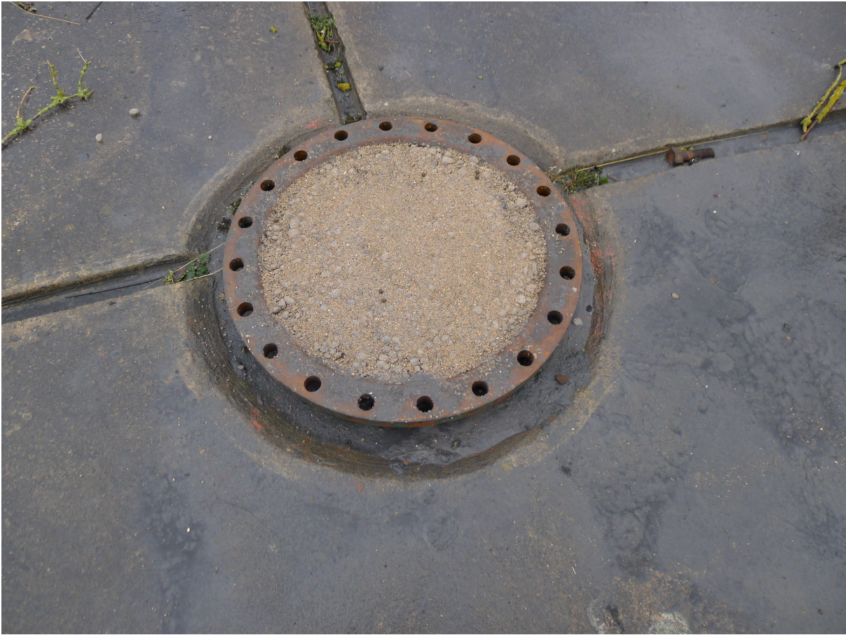
Photograph 54: POL 3B - Tank filled including concrete weathering cap
