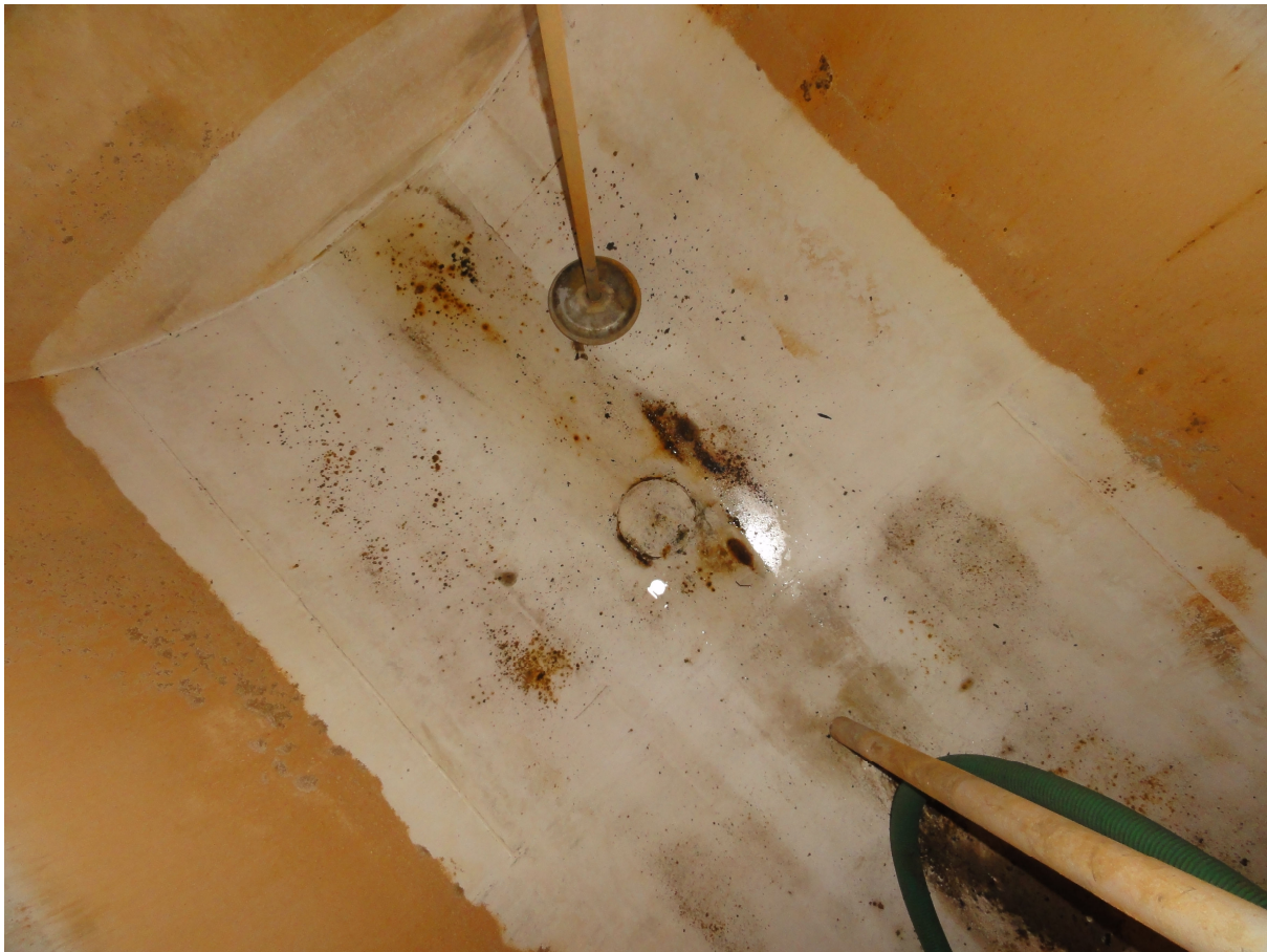
Photograph 277: POL 25C - Tank condition after clean and degas
