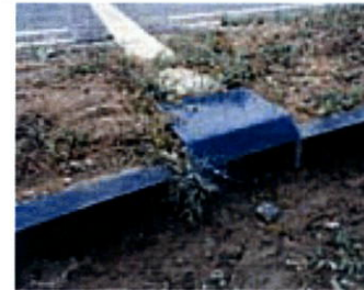
Typical example of amphibian tunnel
