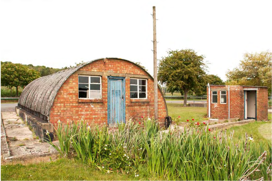
Fire Section D14, Turner's curved asbestos cement hut fire-pump garage and associated latrine block.
