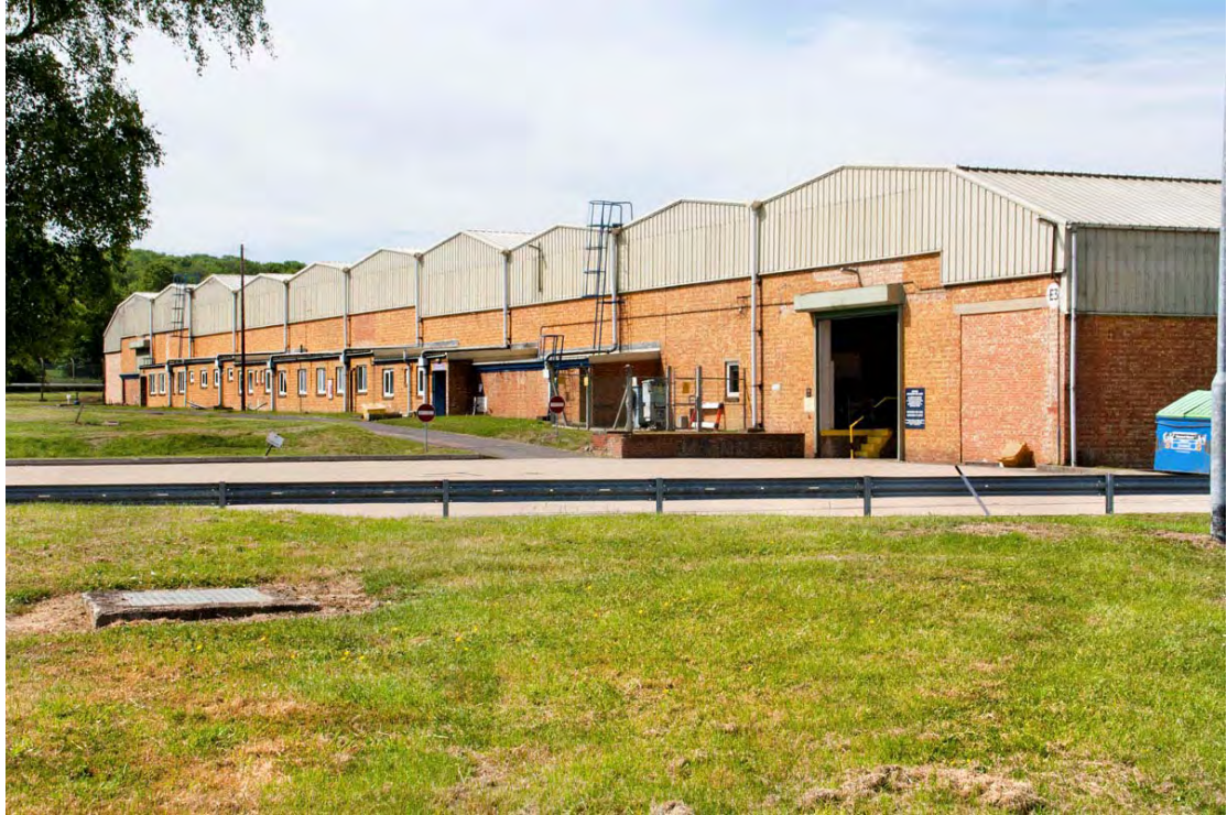
Storage Hangar E3, east elevation showing attached offices, ablutions, and air-raid shelters.
