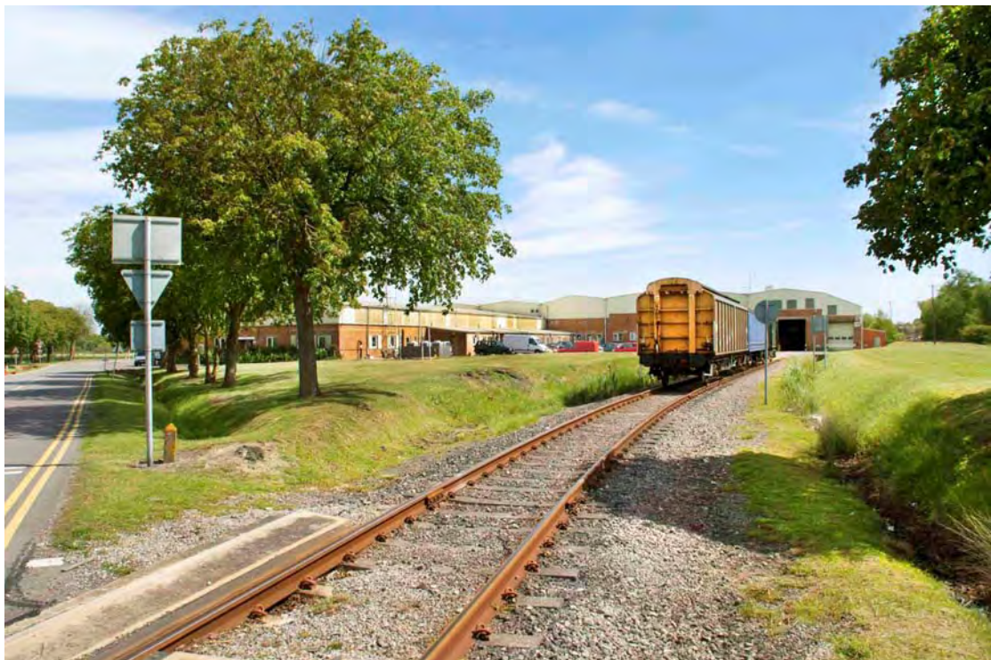
Storage Hangar E1, showing rail access and the attached western range.
