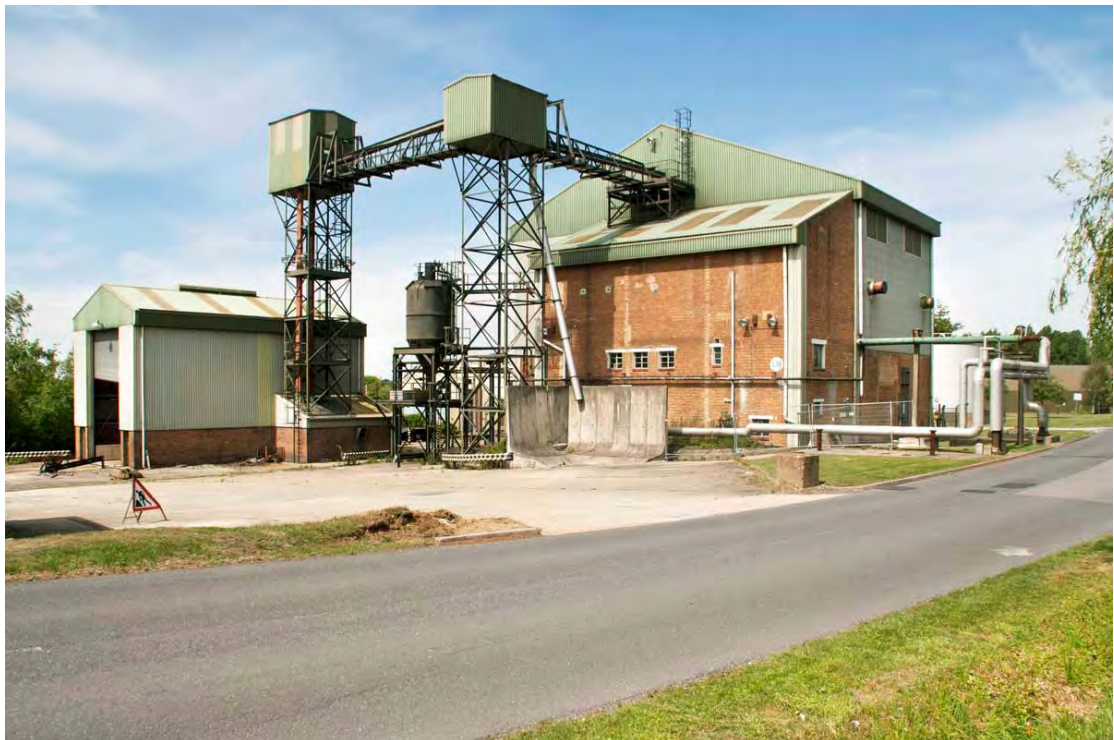
Boiler House E14 and associated coal and ash handling equipment
