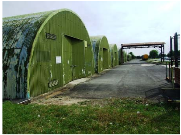
Plate 2: Buildings C30 and C31
