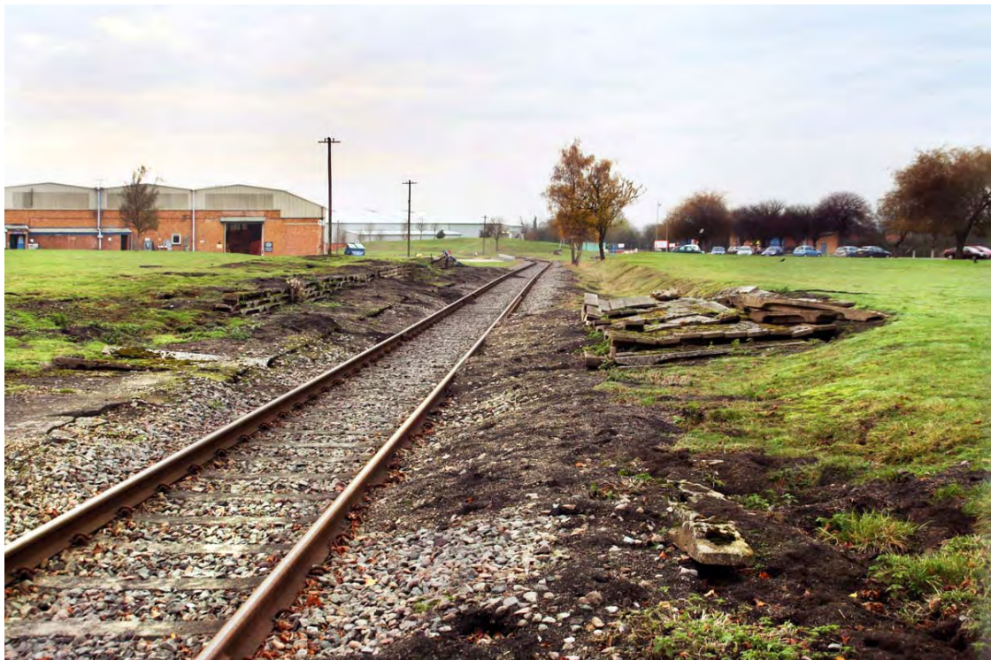
Westacott Platform, partially dismantled
