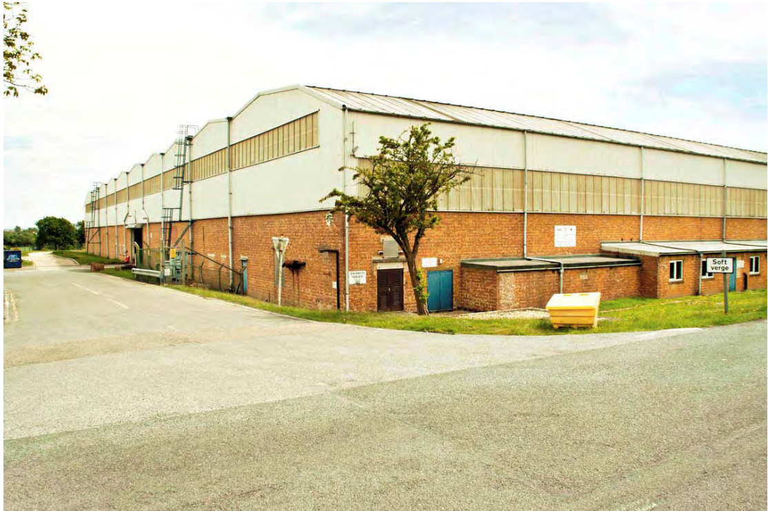
Storage Hangar D6, NB tall roof to allow the use of travelling cranes to lift heavy ordnance
