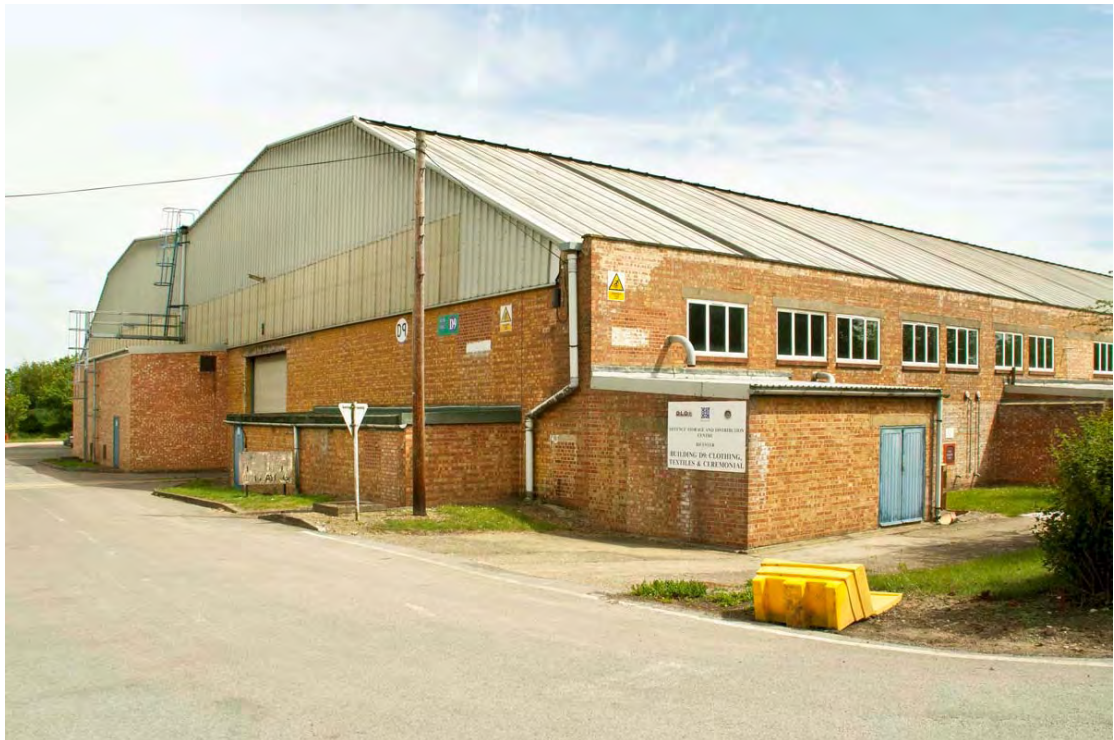
Storage Hangar D9, north elevation, NB tall roof line, rail access, and attached air-raid shelter
