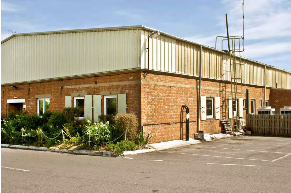
Storage Hangar E1, west range integral air-raid shelter, NB concrete roof line & blast shutters
