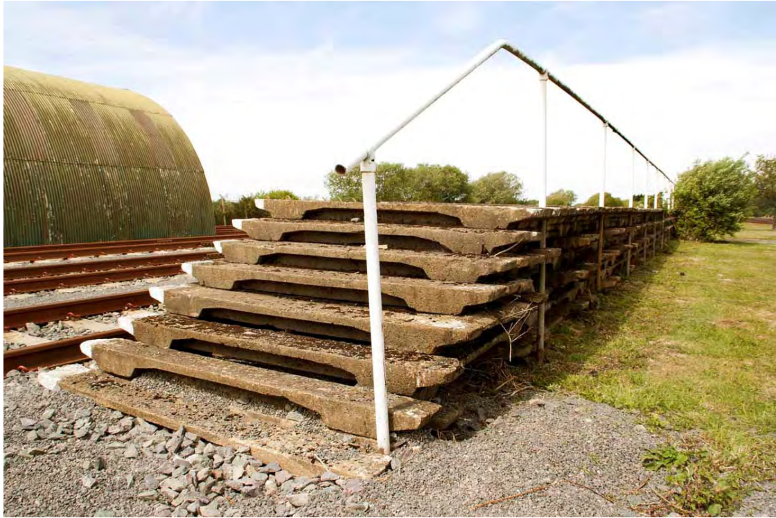
Graven Hill Platform built of up-turned concrete sleepers
