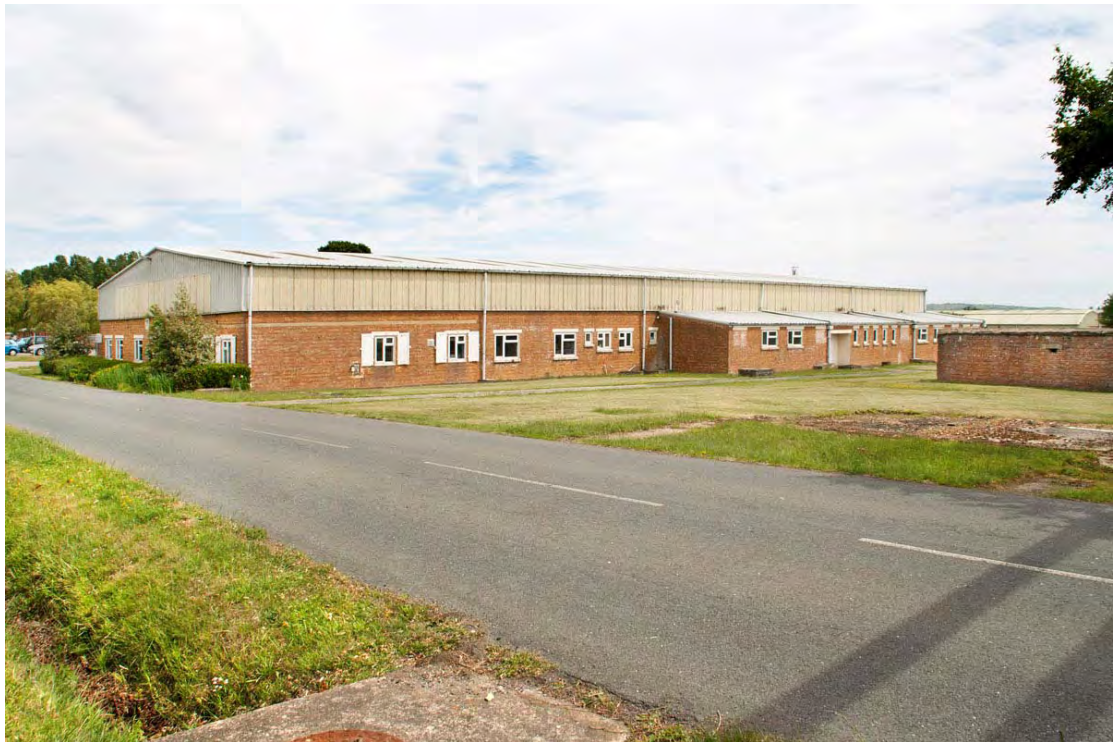
Training Block D3, NB concrete roof line of the integral air-raid shelter & steel blast shutters
