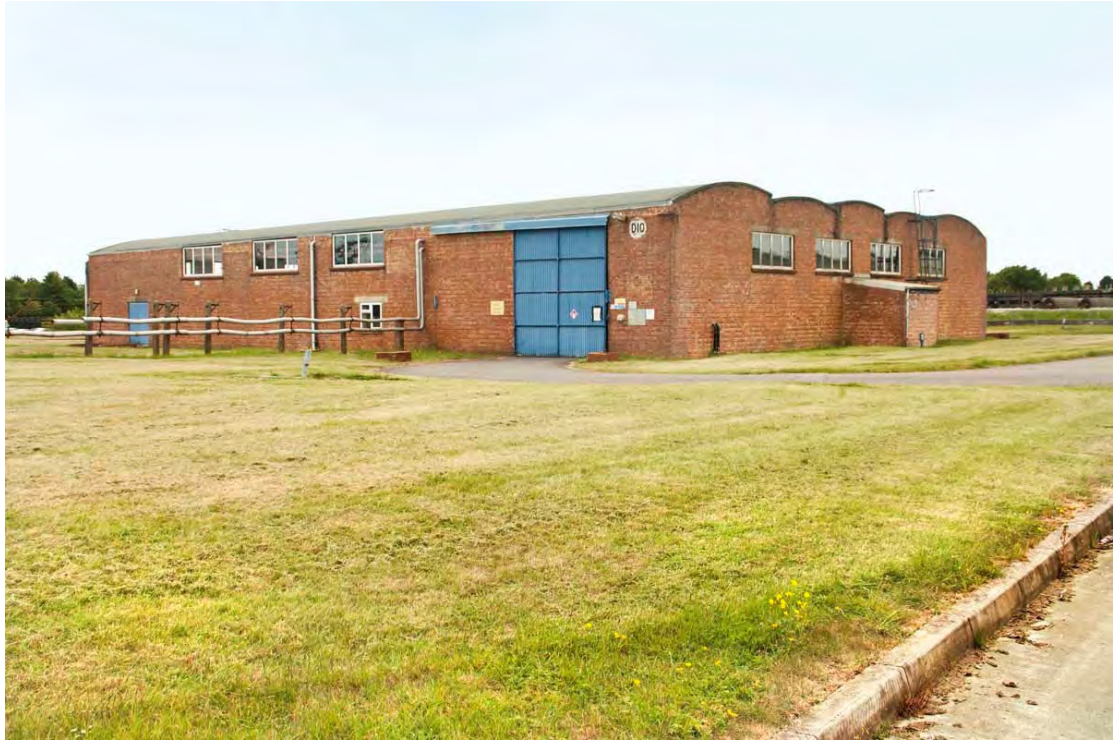
Storage Shed D10, NB high-set windows and reinforced concrete shell roof
