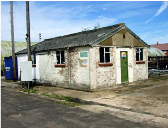
Plate 3: Break Hut at Buildings C30 and C31
