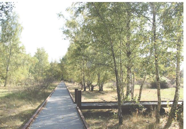
**ABOVE** The elevated walkway at Südgelände Nature Park is made from an anti-slip metal grille deck that spans between 2 former site rail lines.
