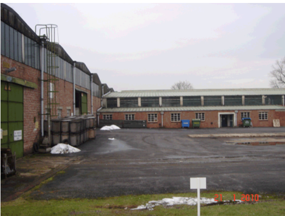
Plate 17: Warehouse A1 and Mechanical Handling Equipment Training Annex
