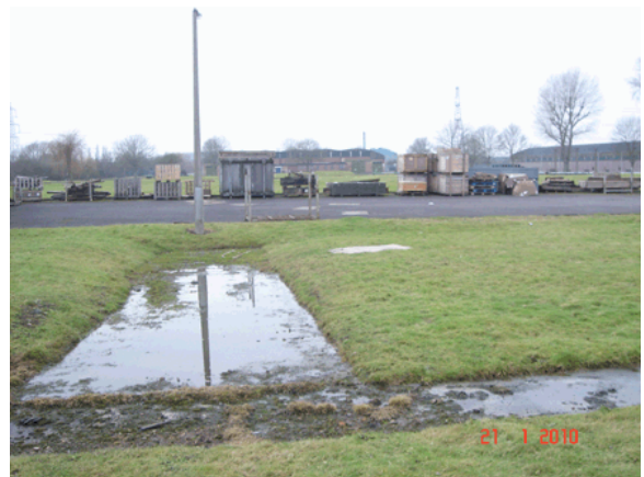
Plate 18: Hardstanding area located to the West of A1
