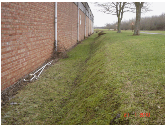
Plate 21: A4 Viewed along Southern Side
