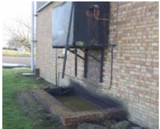
Plate 10: Stained Bunding on Wall Mounted Fuel Tank at Building D2
