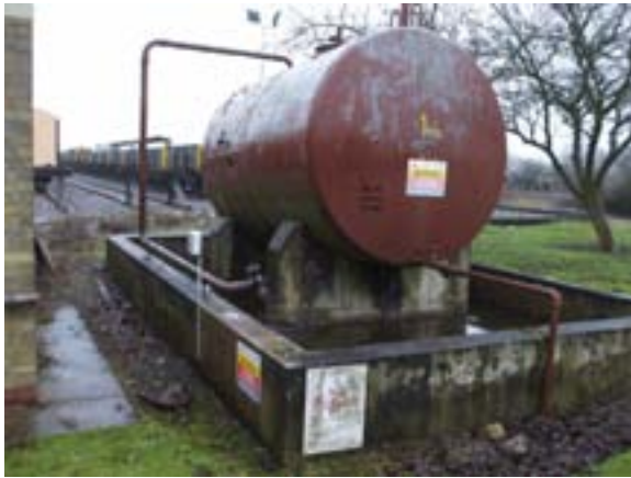
Plate 7: Loco Shed Above Ground Fuel Tank
