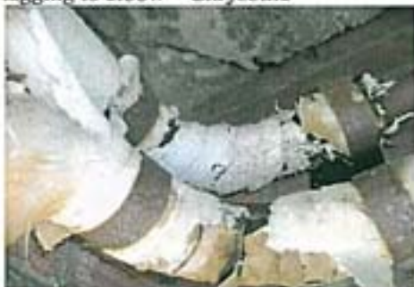
Photo 11 – EX02 Porch – Sample 7: Pipe lagging to elbow – Chrysotile
