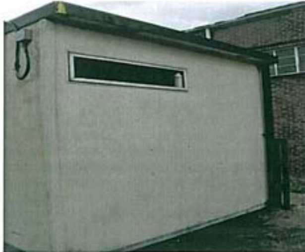
Photo 1 – External EX01 Main, Sample 1; Textured coating to external walls – No asbestos detected.
