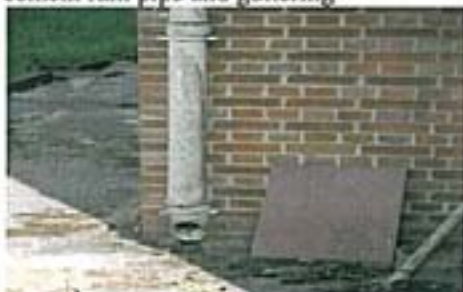
Photo 9 – External EX01 – Strongly Presumed cement rain pipe and guttering
