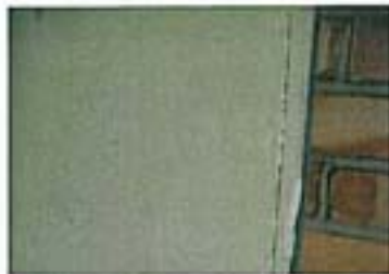
Photo 3 – 1.23 Store Room – Sample 2: Insulation panel to door x2 – Chrysotile
