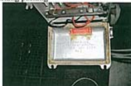
Photo 22 – 2.01 Roof Void – Sample 11: Rope (in switch box x4) also used as backing packing
