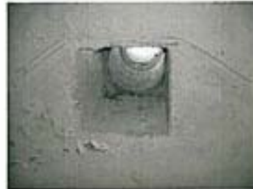
Photo 2 – 1.23 Store Room – Strongly Presumed asbestos to cement sleeve through ceiling to roof
