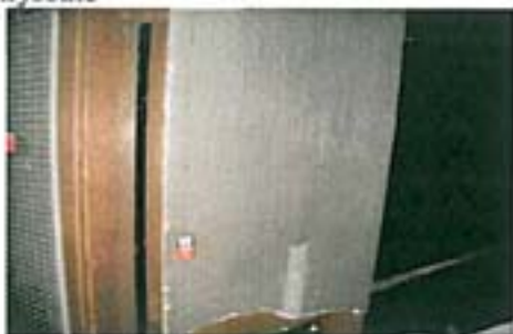
Photo 19 – 2.01 Roof Void – Sample 10: Insulation panel and debris to door – Chrysotile
