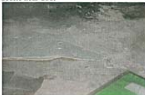
Photo 7 – G30 under stage – Strongly Presumed Asbestos insulating board panel and debris near door
