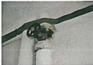
Photo 5 – G18 Lobby/foyer – Sample 4: Gasket to pipes (x8) - Chrysotile
