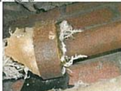
Photo 12 – EX02 Porch – Strongly Presumed asbestos to rope (wrapped around pipe lagging)
