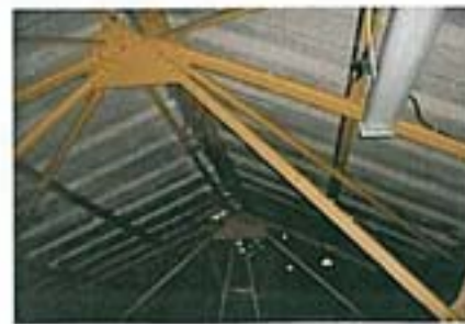
Photo 18 – 2.01 Roof Void – Sample 9: Cement sheeting to roof – Chrysotile
