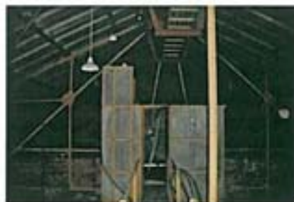
Photo 20 – 2.01 Roof Void – As Sample 10: Durasteel panels – Chrysotile
