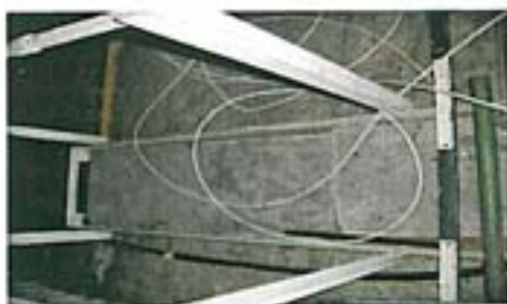
Photo 25 – 2.01 Roof Void – As Sample 9: Cement panel below walkway – Chrysotile
