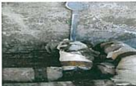
Photo 15 – EX03 Porch – As Sample 7: Pipe lagging to elbow – Chrysotile
