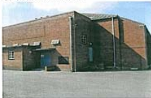
Photo 17 – EX01 – Strongly Presumed asbestos to cement facia
