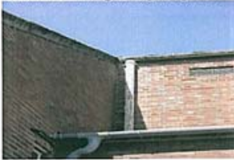
Photo 13 – EX01 – Strongly Presumed asbestos to cement guttering at high level
