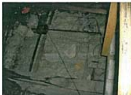
Photo 24 – 2.01 Roof Void – As Sample 9: Cement debris – Chrysotile
