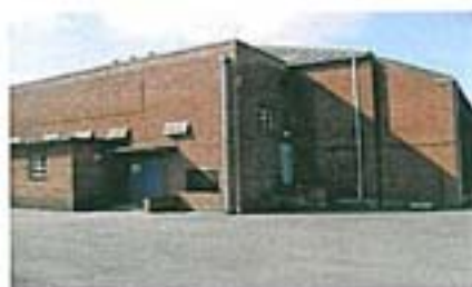
Photo 27 – EX01 External – Strongly Presumed cement facia to roof
