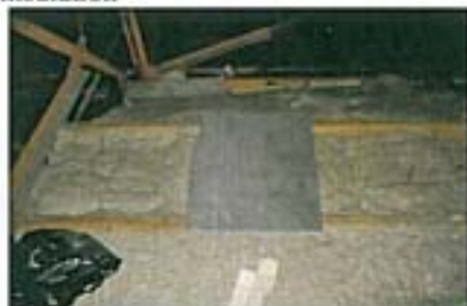
Photo 21 – 2.01 Roof Void – Strongly Presumed asbestos to Durasteel panel on top of 2m insulation
