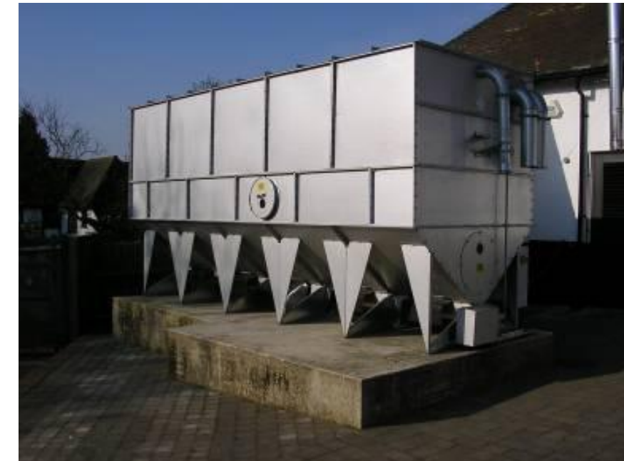
Figure 4.9: Example of biomass fuel storage: External pellet silo
