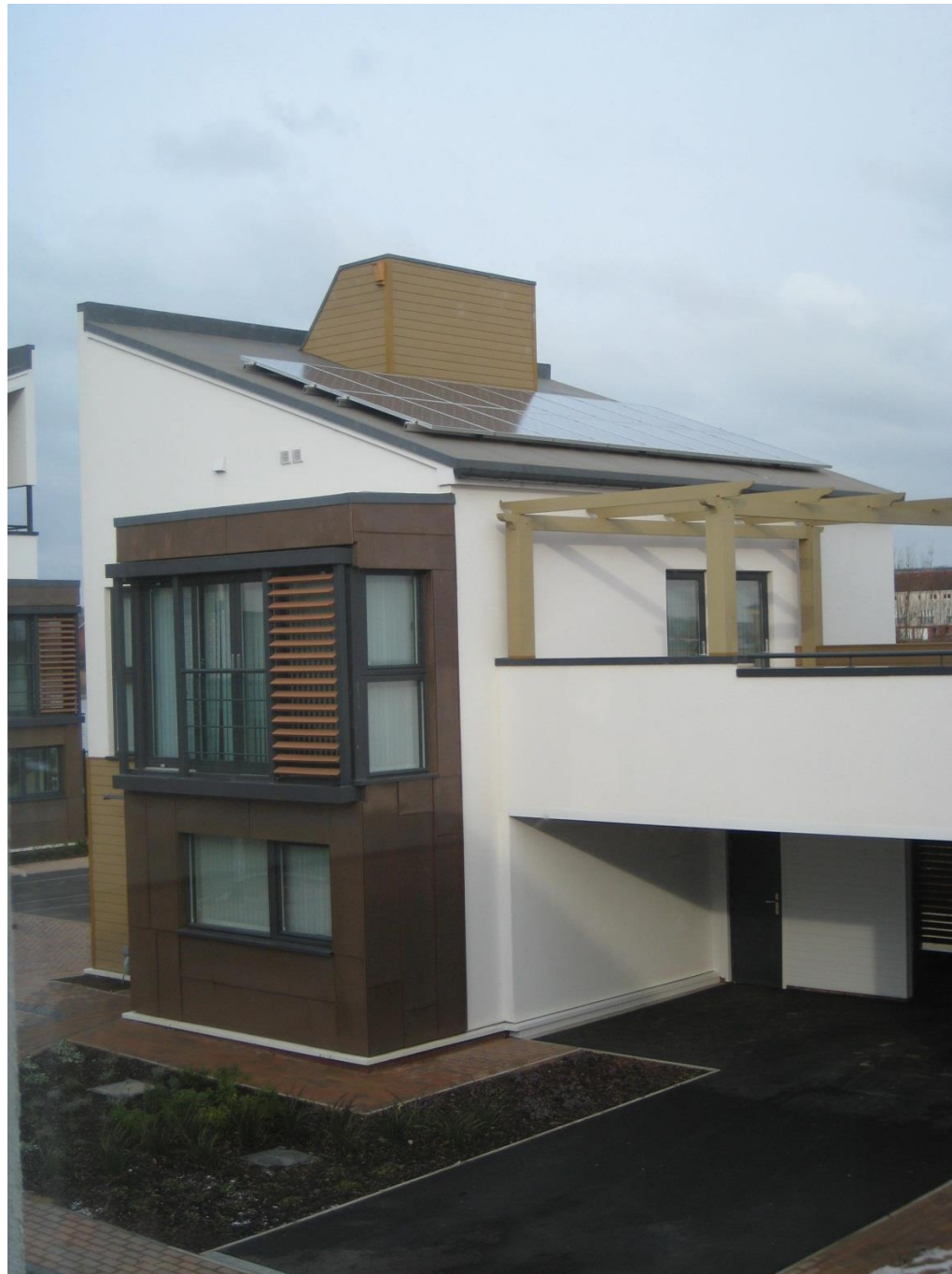
Figure 3.1: Code for Sustainable Homes Level 5 compliant dwelling in Newport, Wales, demonstrating the great amount of photovoltaics required to meet the standard. The development also includes a district energy system with CHP and biomass boilers
