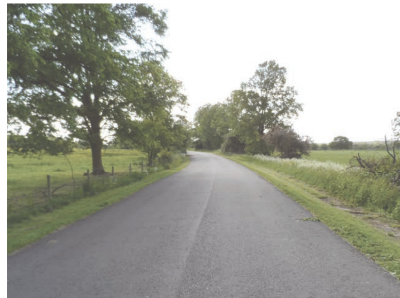
ABOVE Existing ‘rural lane’ at Graven Hill showing the proposed, simplistic highway design of a single, shared macadam surface with grass verges either side.
