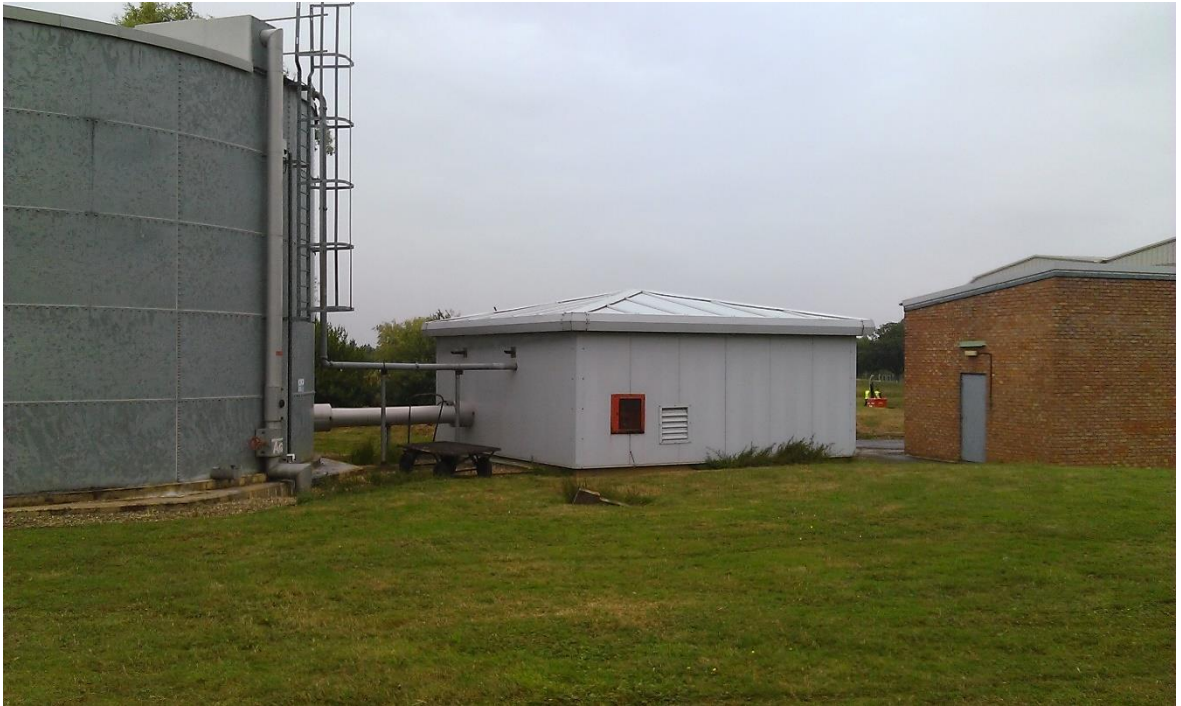
Existing water tank and diesel water pump house. Building E3 is immediately to the right of and behind the brick garage building on the RHS of the photo, which is also to be retained.
