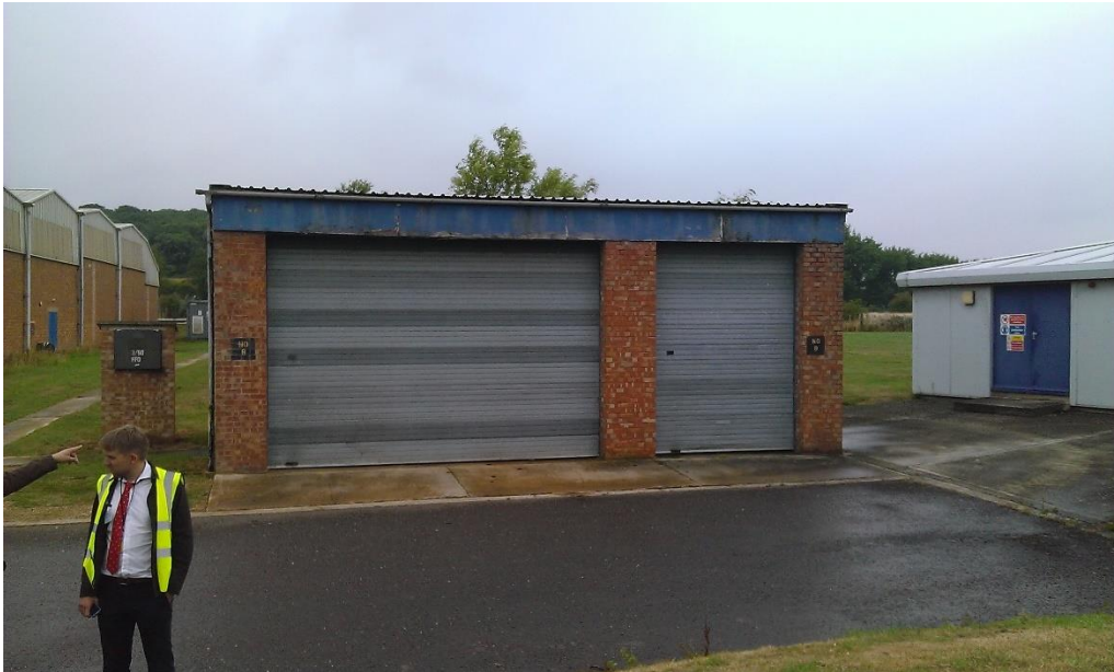
Building E3 on LHS. Brick garage building to be retained. Existing water tank diesel pump house on RHS to be retained.
