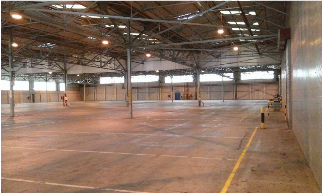
Typical photo of MOD Building E3 – Internal
