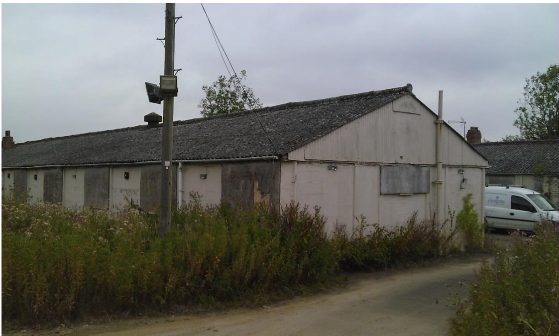
Typical photo of Rodney House Social Club Out Buildings
