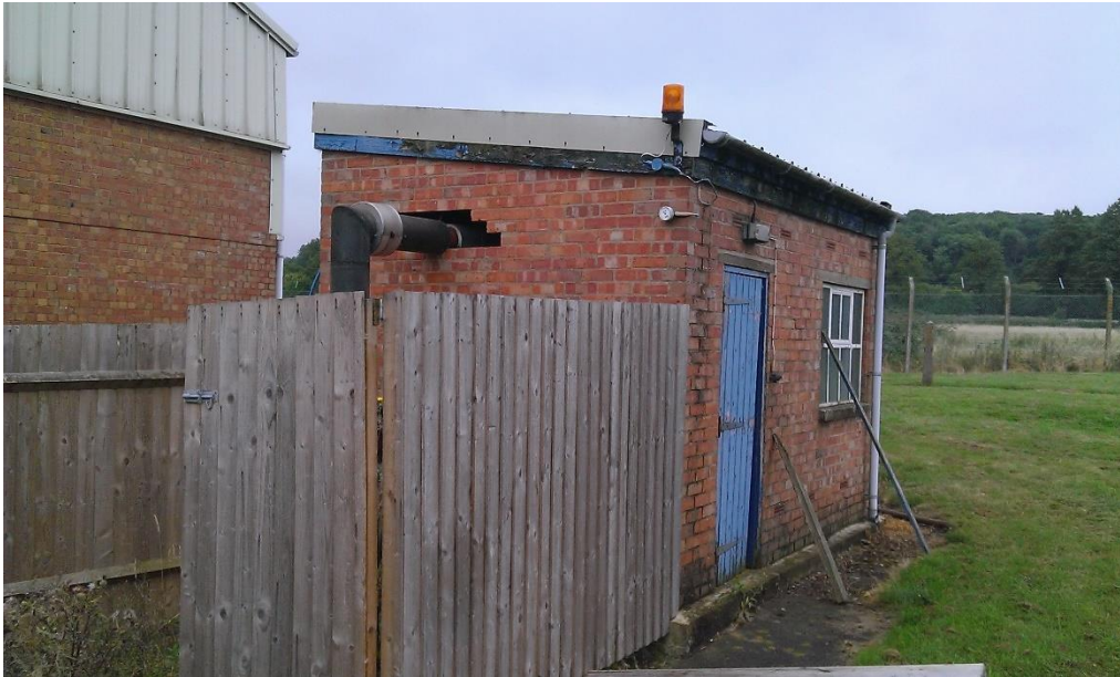
Former brick diesel Generator Building to be demolished. Building E3 on LHS.
