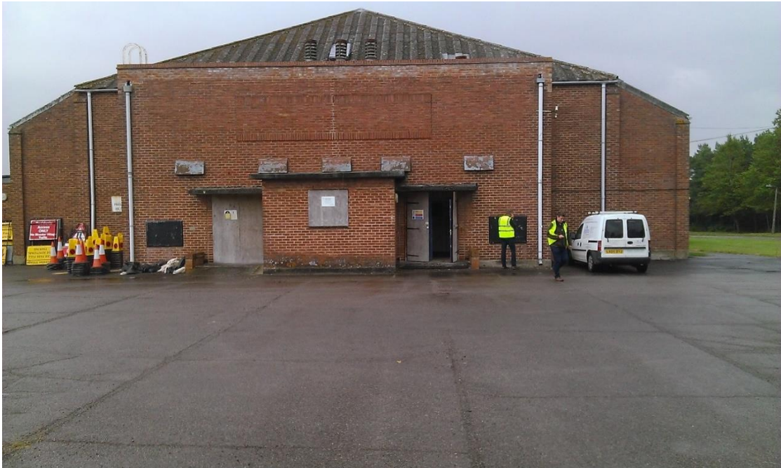
Typical photo of Former Garrison Theatre – End Elevation - Includes a basement
