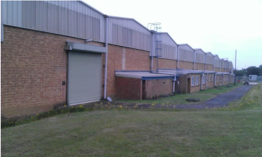
Typical photo of MOD Building E3 – External
