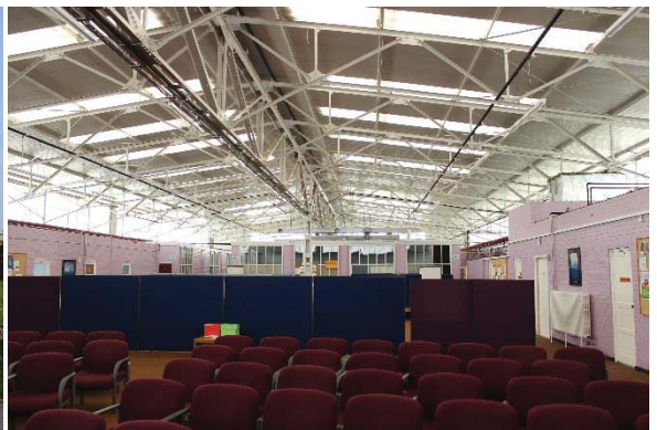
Figure 36: Interior view of Building D3
