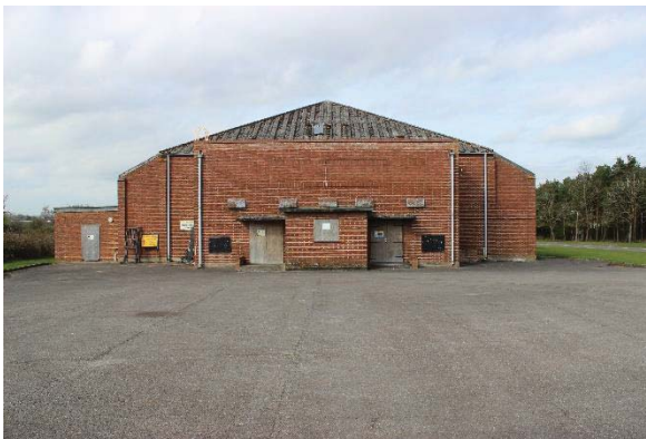
Figure 25: Front (south) elevation
