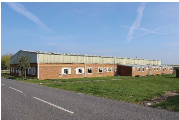
Figure 35 : View of Building D3 from north west
