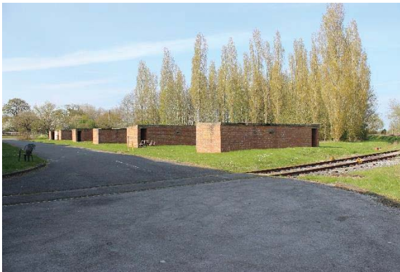
Figure 27 : Air raid shelters adjacent to Building D2
