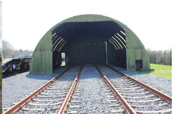
Figure 16: Romney hut (Building D98)
