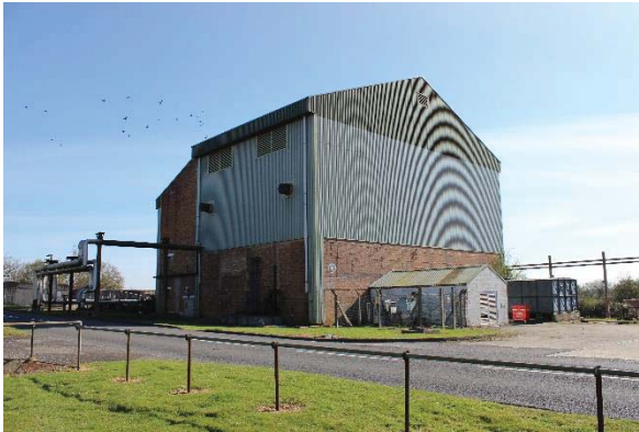
Figure 33 : View of boiler house from north
