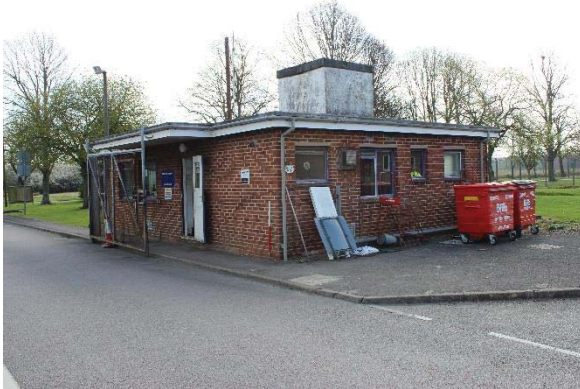
Figure 37: Guard post at E Site entrance
