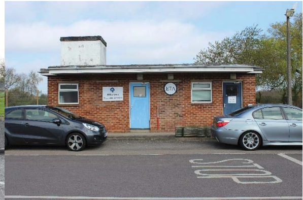
Figure 38: Guard post at E Site entrance
