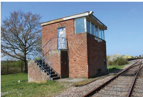
Figure 23: D Site Signal Box
