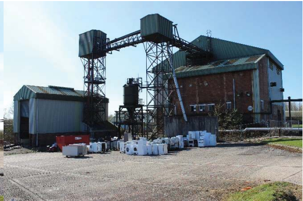
Figure 34: View of boiler house from south east
