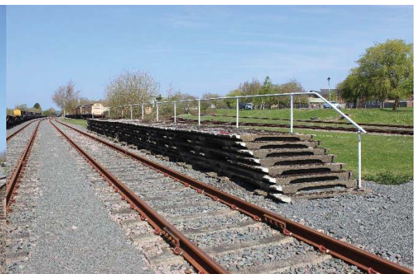
Figure 24: Platform made of sleepers (D Site)
