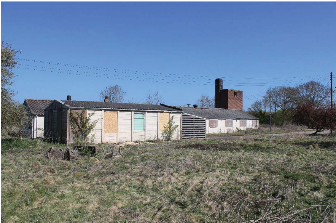
Figure 14: View of Rodney House from south-west
