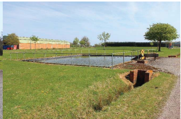
Figure 32: Pond adjacent to Building D4
