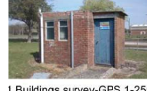
Level 1 Buildings survey-GPS 1-255
