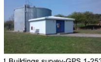
Level 1 Buildings survey-GPS 1-253
