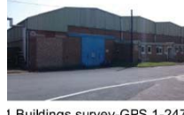
Level 1 Buildings survey-GPS 1-247
