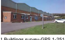
Level 1 Buildings survey-GPS 1-251
