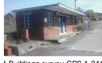
Level 1 Buildings survey-GPS 1-241
