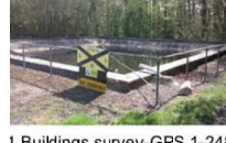
Level 1 Buildings survey-GPS 1-248
