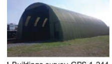
Level 1 Buildings survey-GPS 1-244
