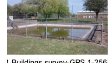
Level 1 Buildings survey-GPS 1-256
