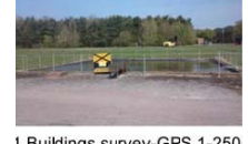
Level 1 Buildings survey-GPS 1-250
