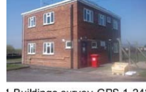
Level 1 Buildings survey-GPS 1-242
