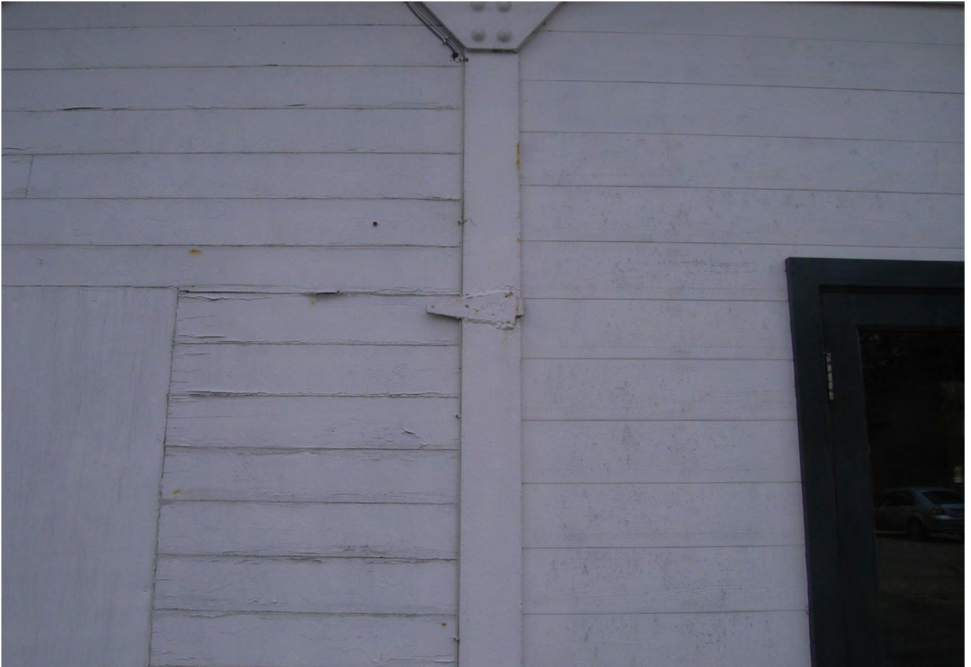
Plate 115.7 An original hinge surviving on a column
