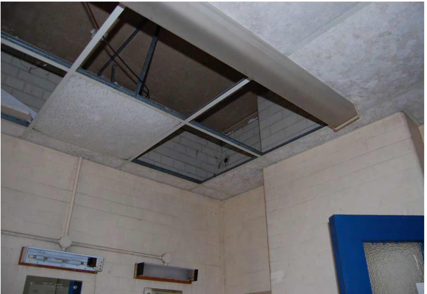
Plate 485.9 The glazed brickwork in the ablutions, visible above suspended ceiling
