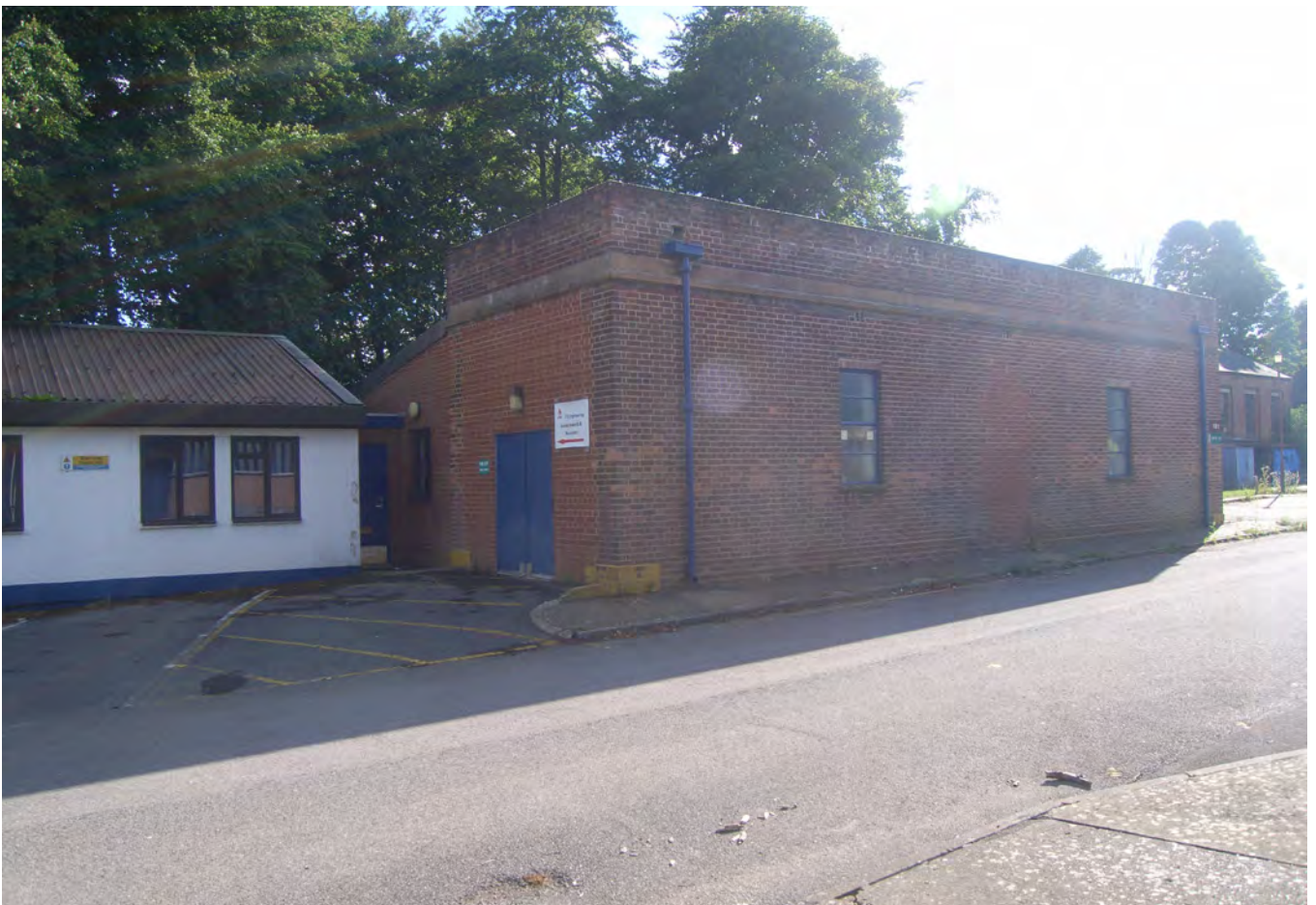
101.2/14 Maintenance Shop, showing brick infill to south and west elevations
