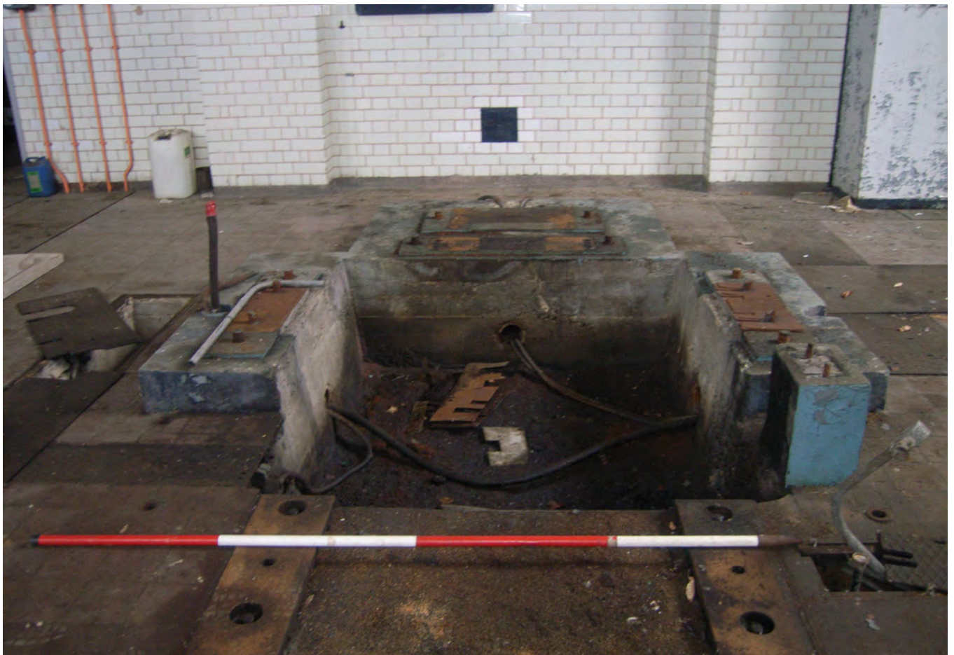
Plate 114.12 The support structure for the former machinery
