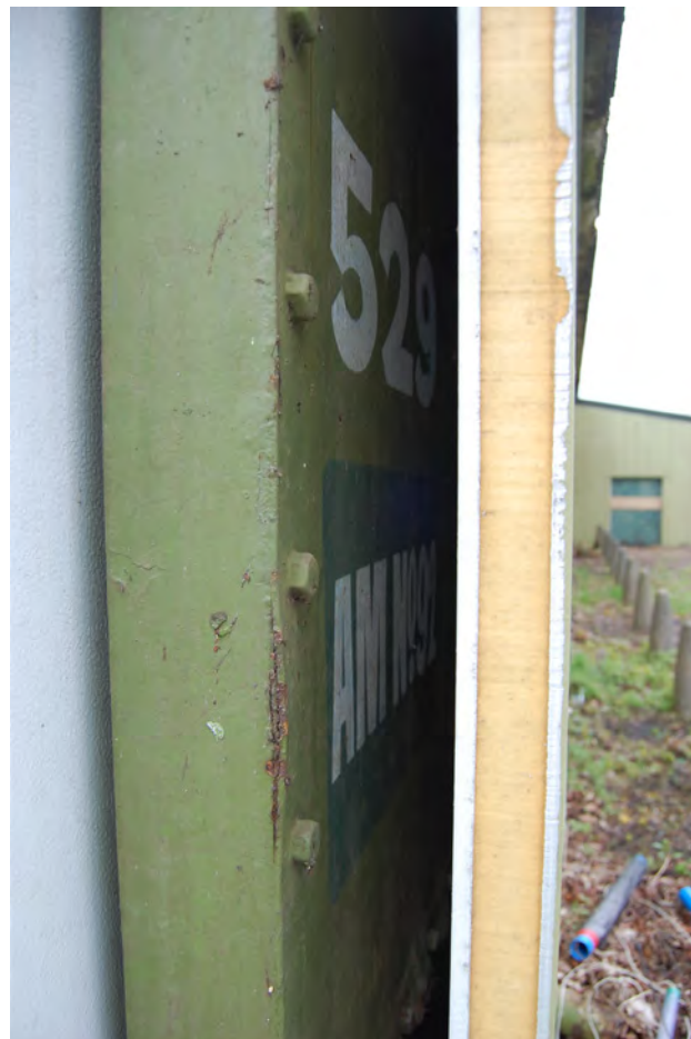
Plate 529.10 Primary metal cladding encased behind 1980s panels
