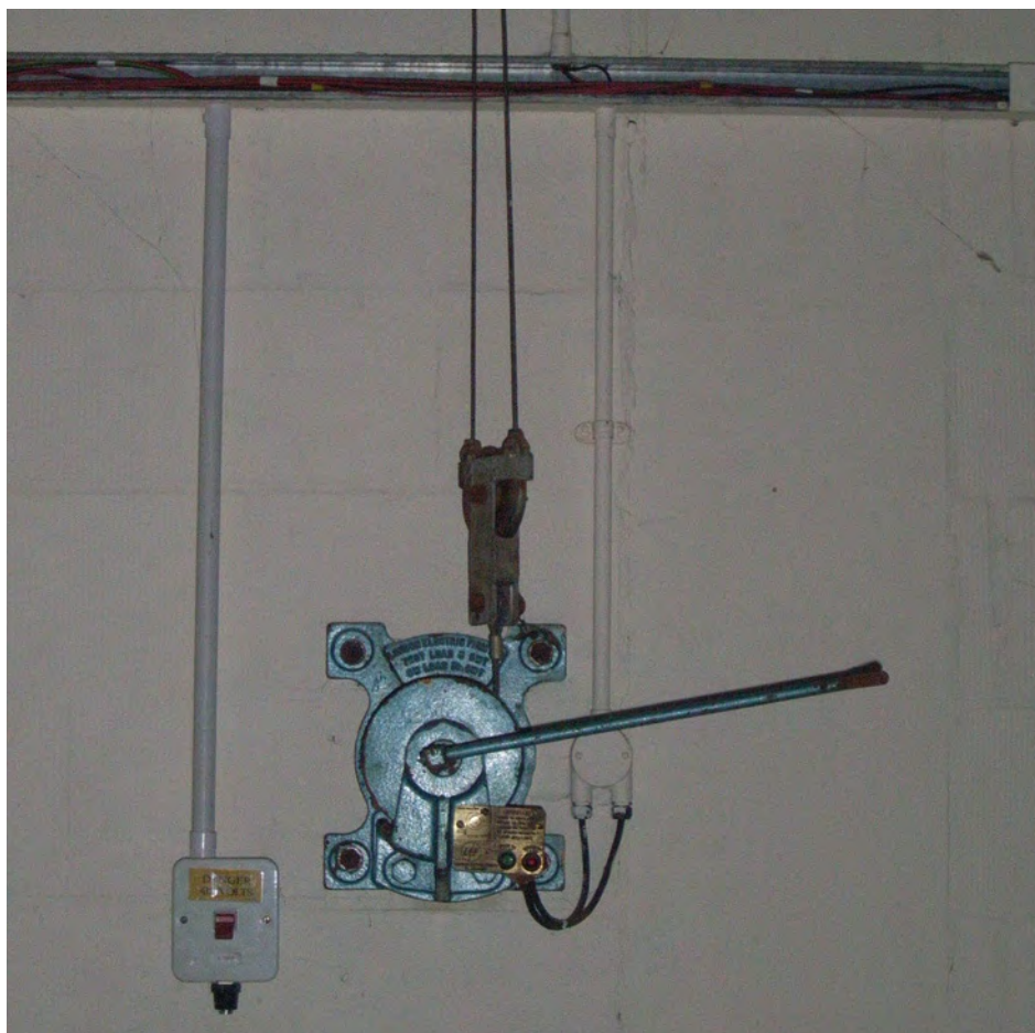
Plate 293.6 Detail of lighting pulley control within flight simulator room
