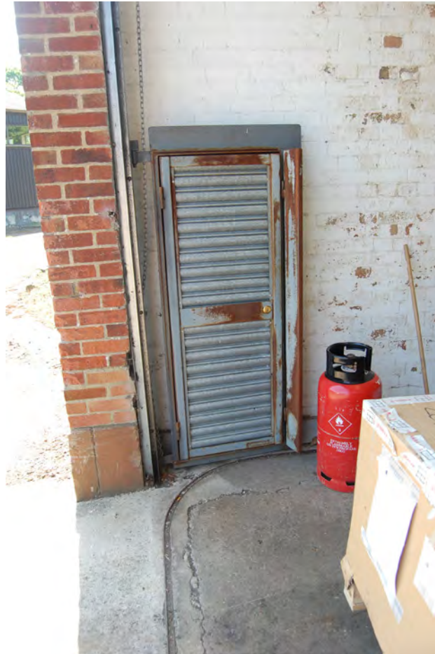
Plate 119.3 Personnel door for the roller shutter and the rail for the former door
