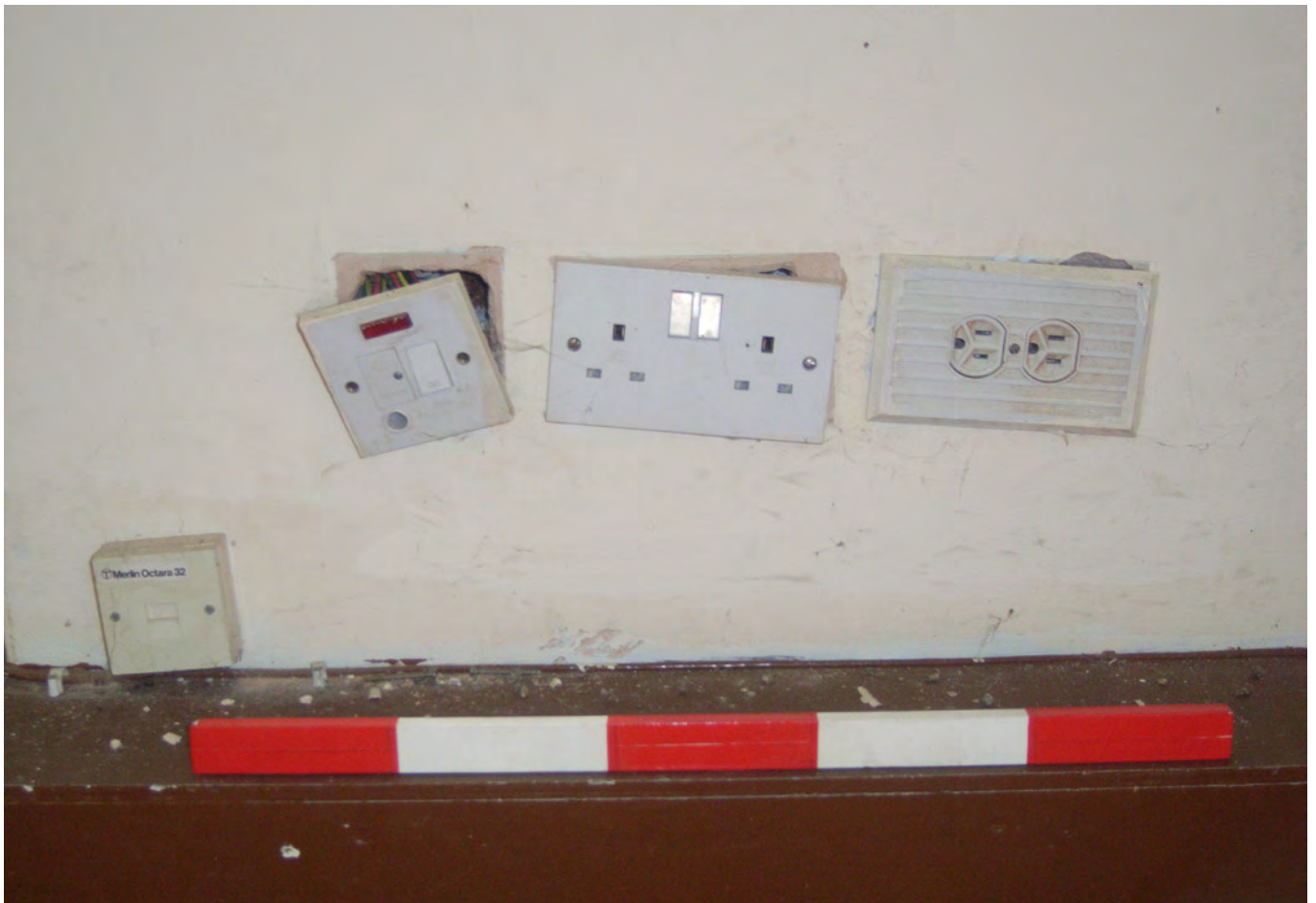
Plate 488.13 An example of the American and British power sockets
