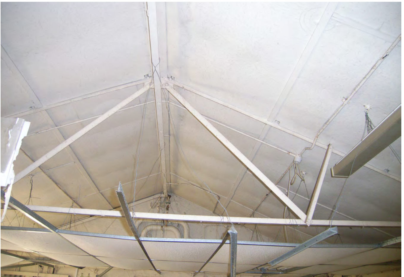
Plate 804-815.12 Roof trusses
