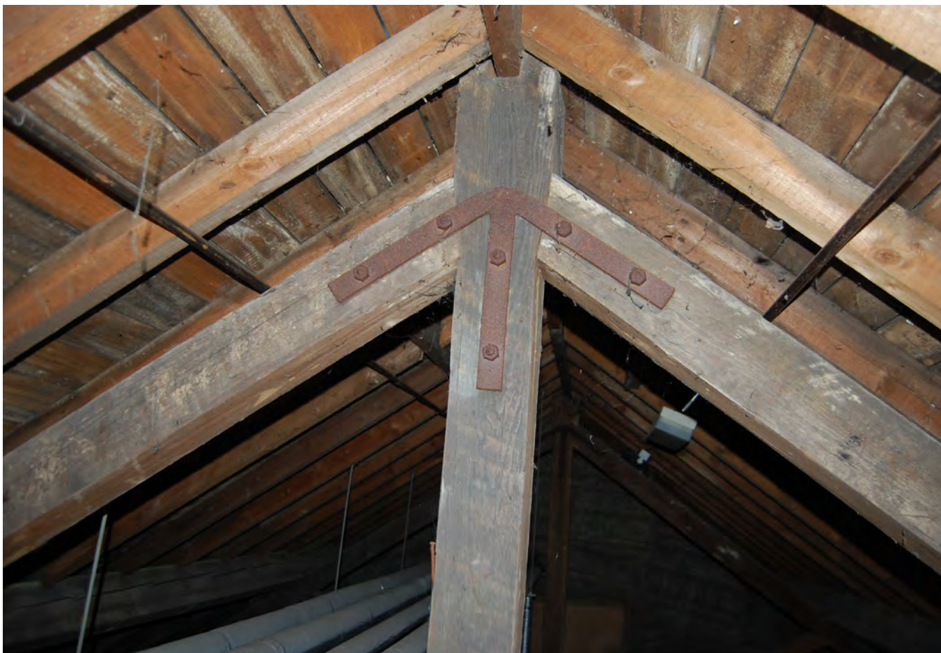
Plate 480.15 Truss apex detail
