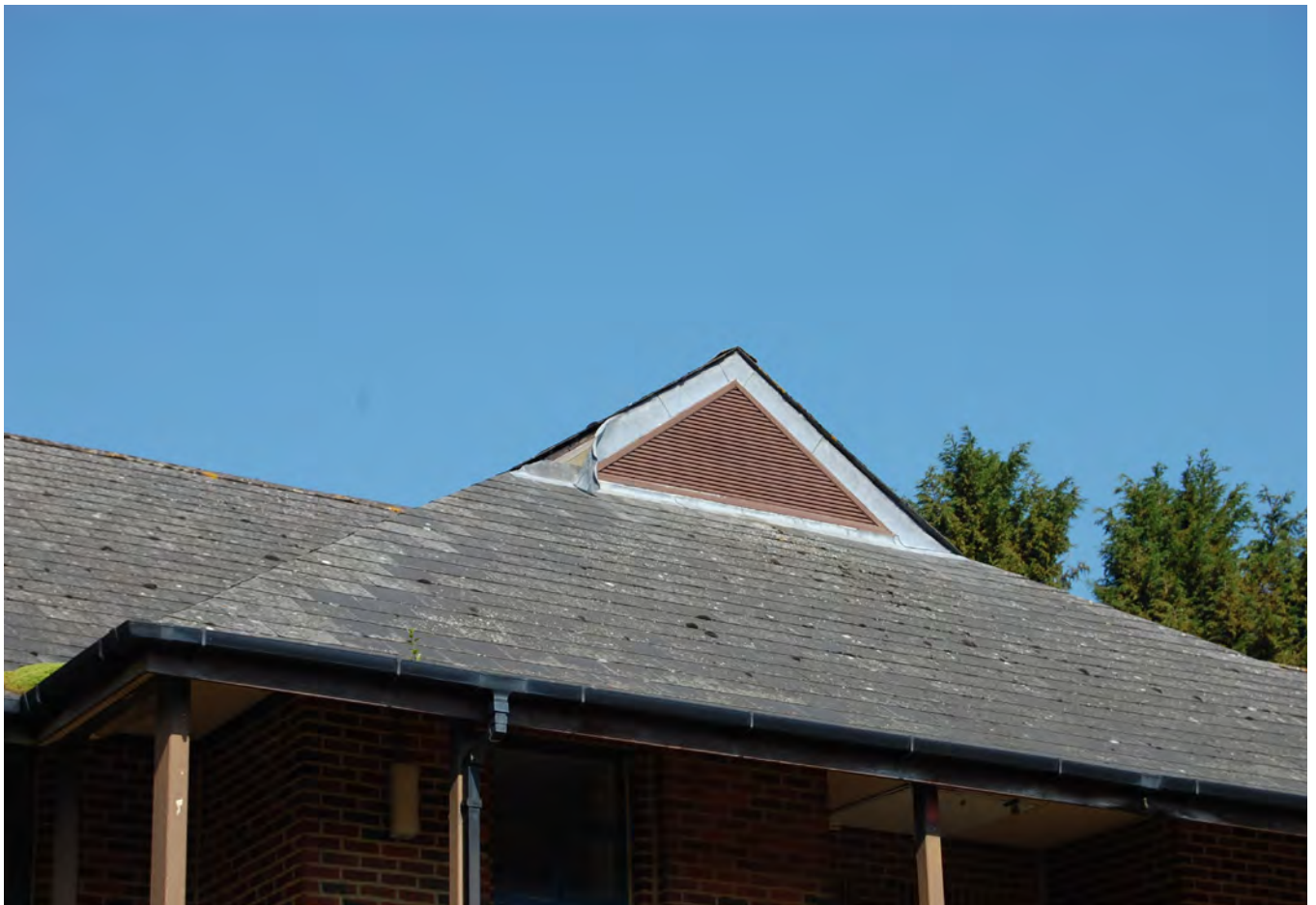
Plate 466.5 Gablet in roof added in 1980s alterations
