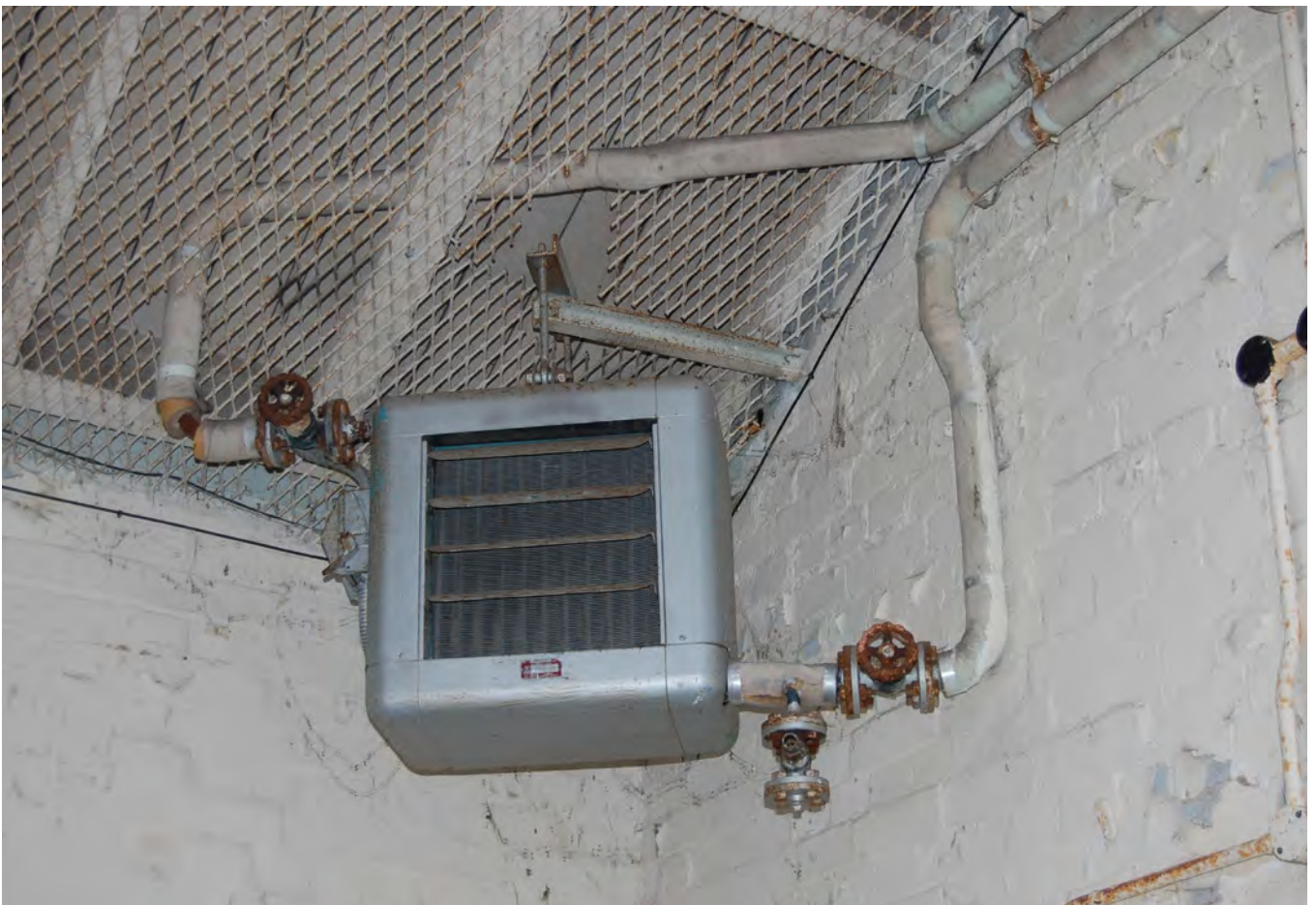
Plate 146.12 Space heater in the Lubricant Store
