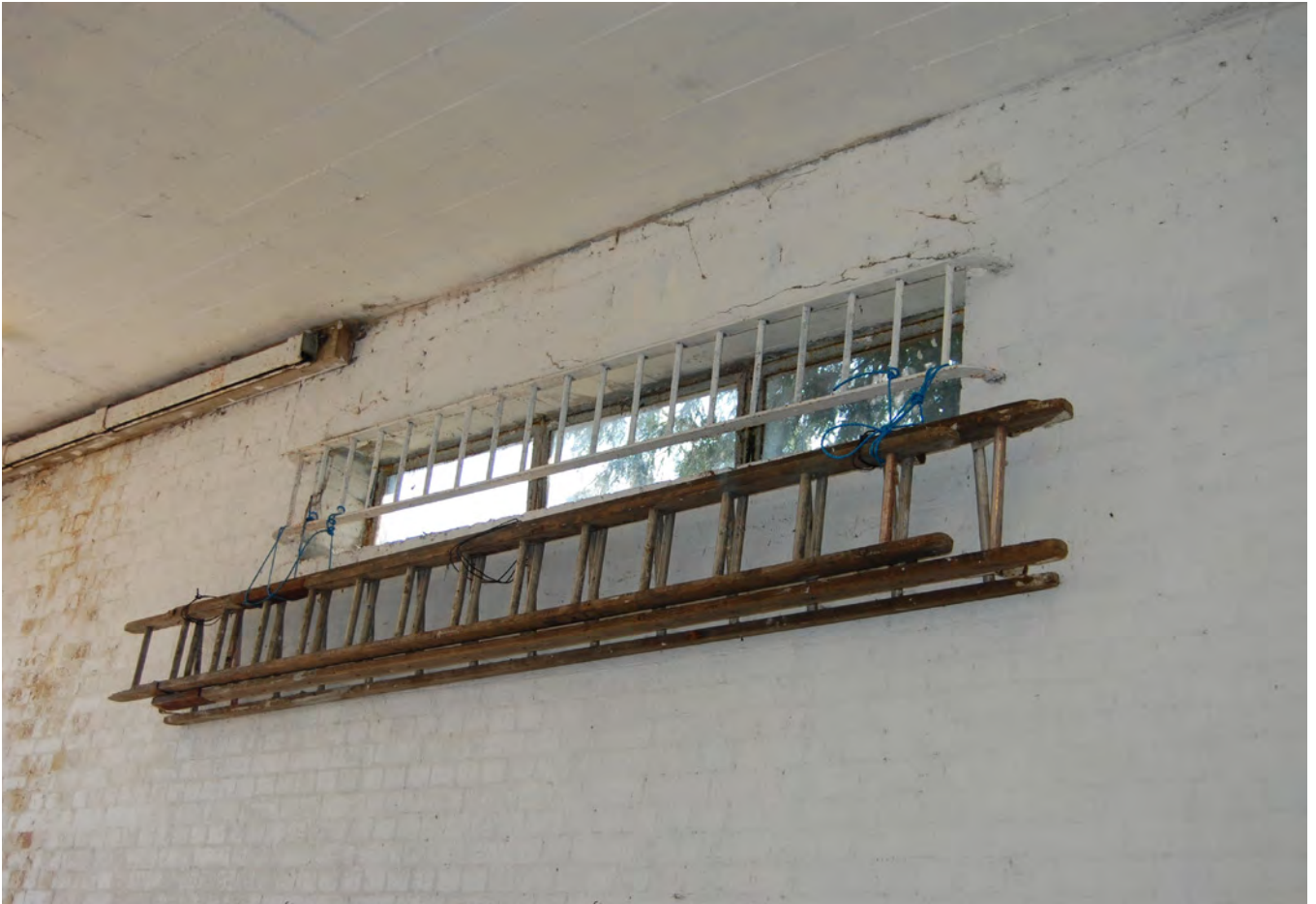
Plate 119. 7 A high level window, barred internally
