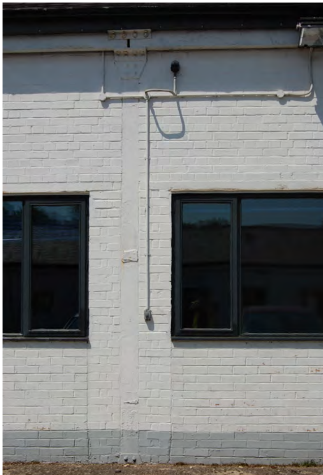
Plate 117.3 Original hinges surviving on a column
