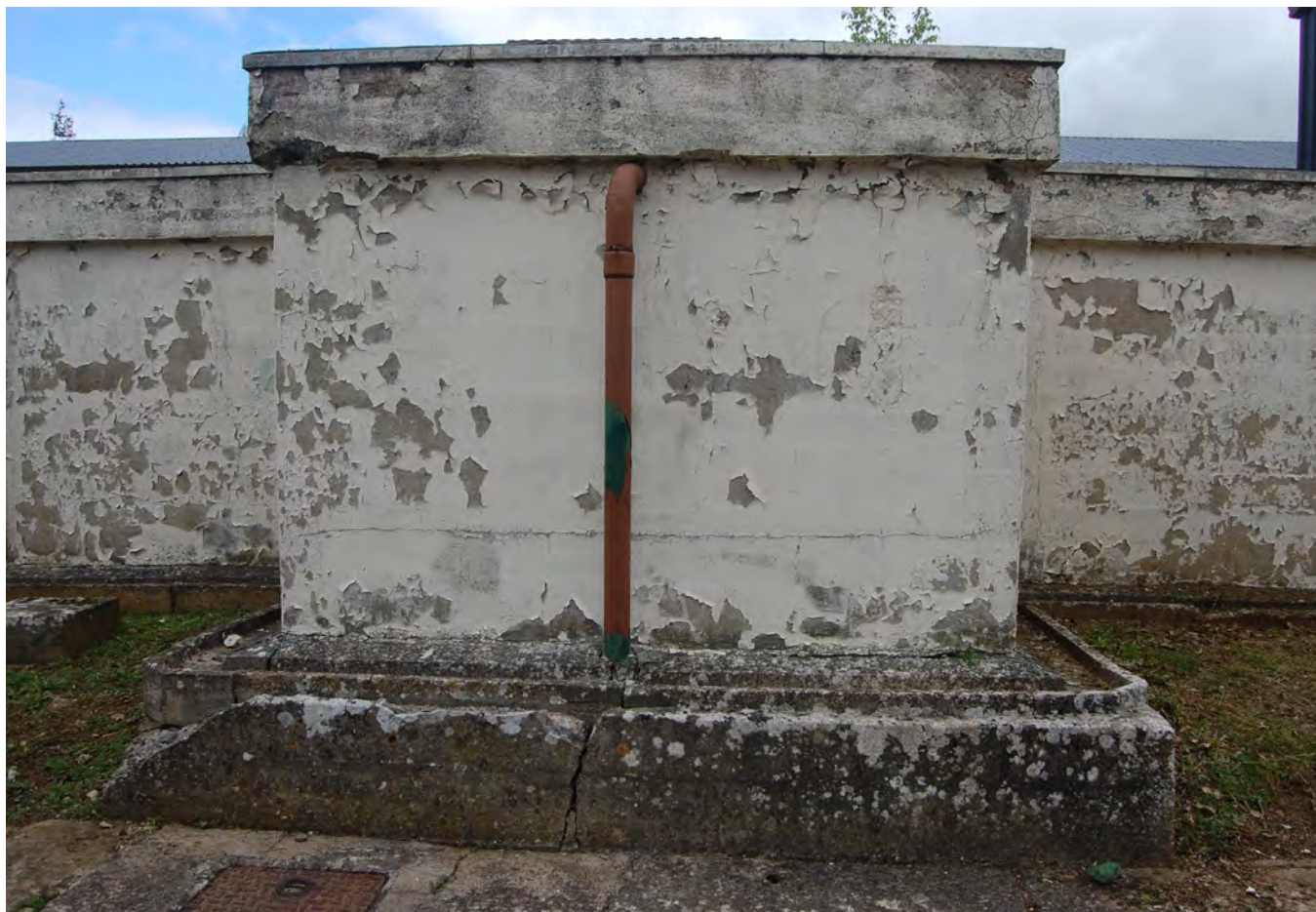
Plate 107.3 Base of water tank showing projection and channel running around the footprint
