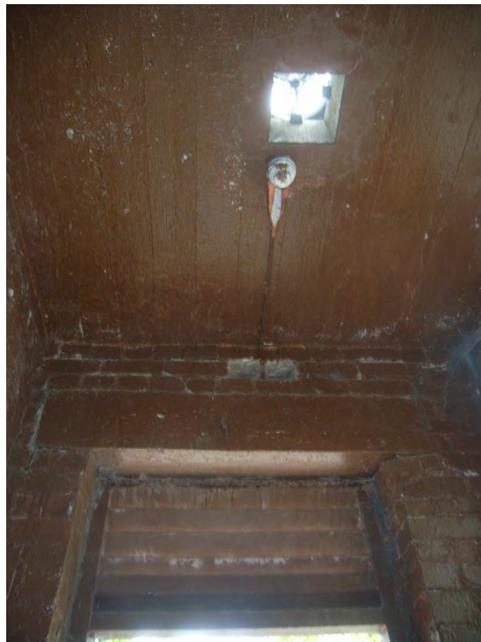
Plate 145.2 Example of the ventilation louvres above the doors and concrete roof
