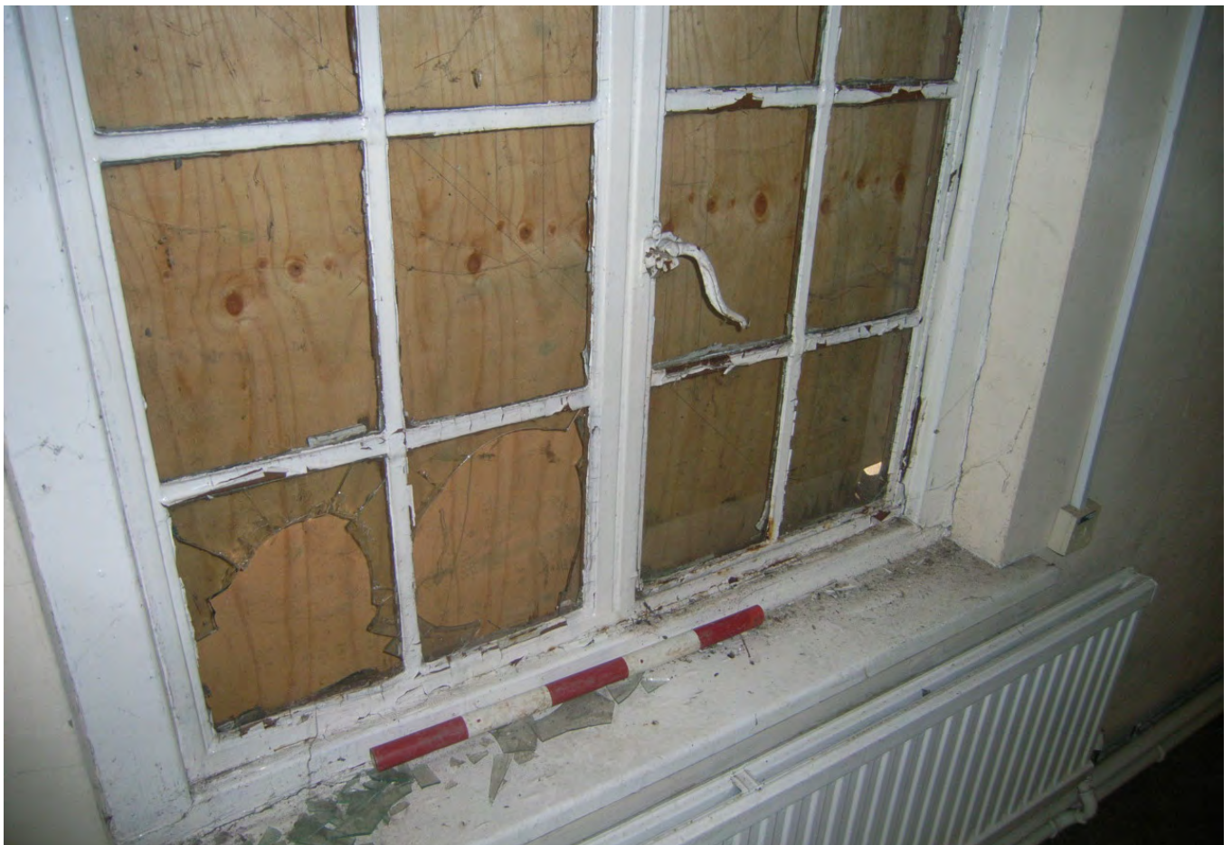
Plate 459.14 Typical primary crittall type window
