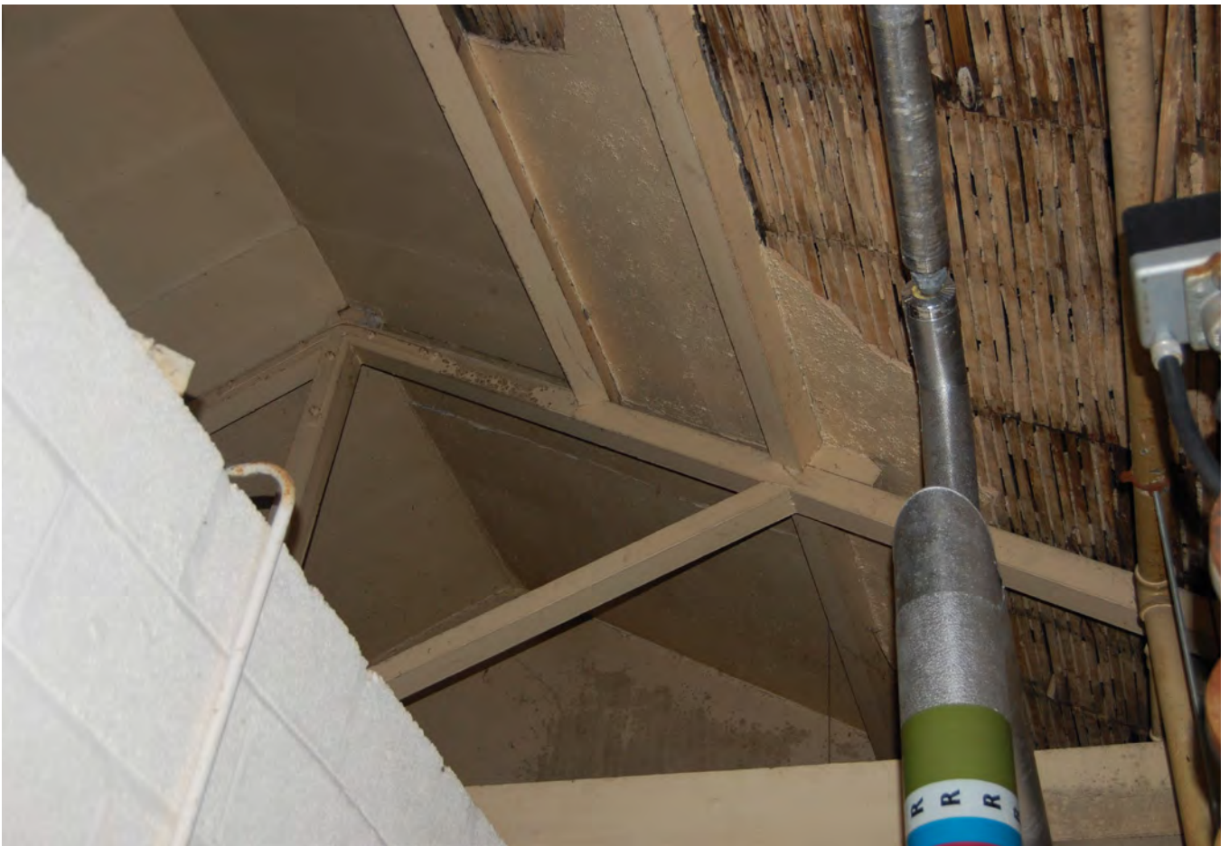
Plate 474.15 The roof truss and original ceiling above the calorifier and supply store
