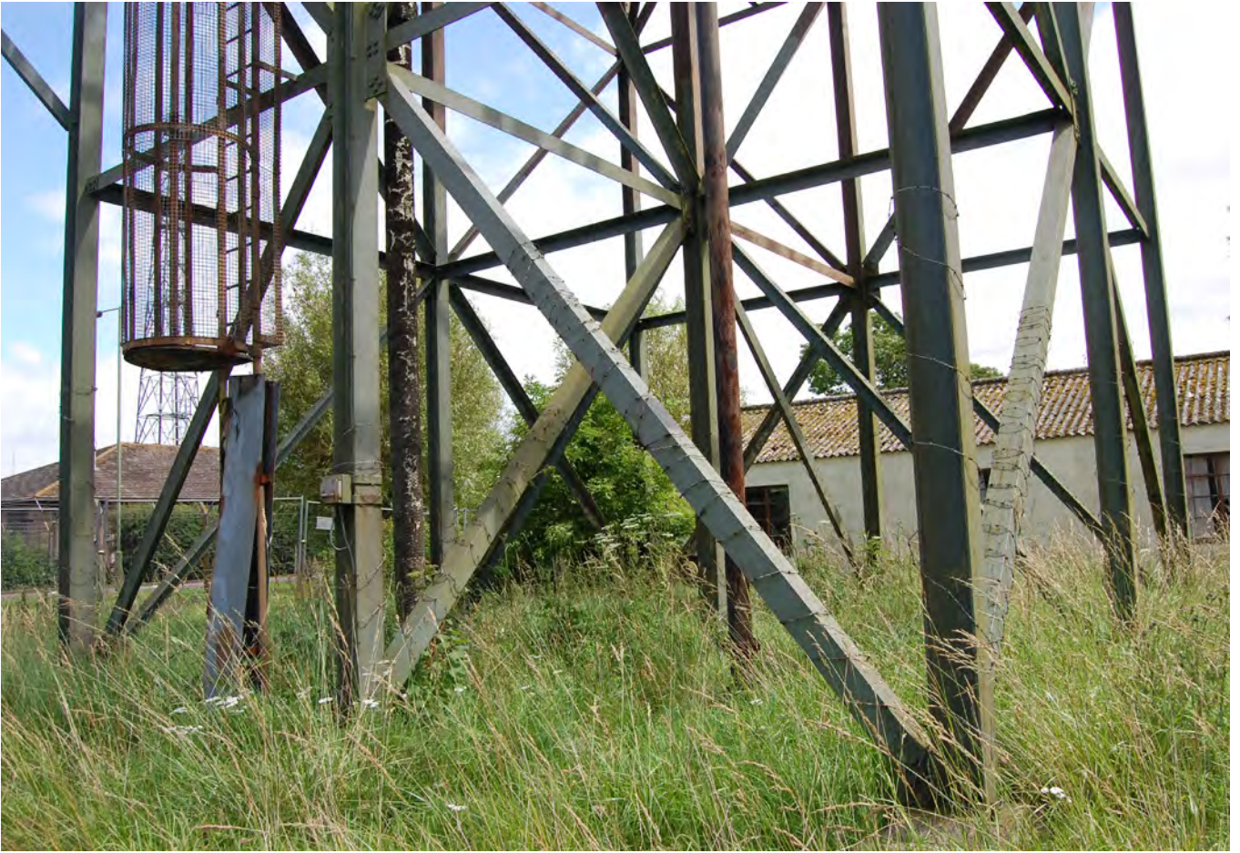
Plate UH74.5 Base of tower, with concrete pads just visible
