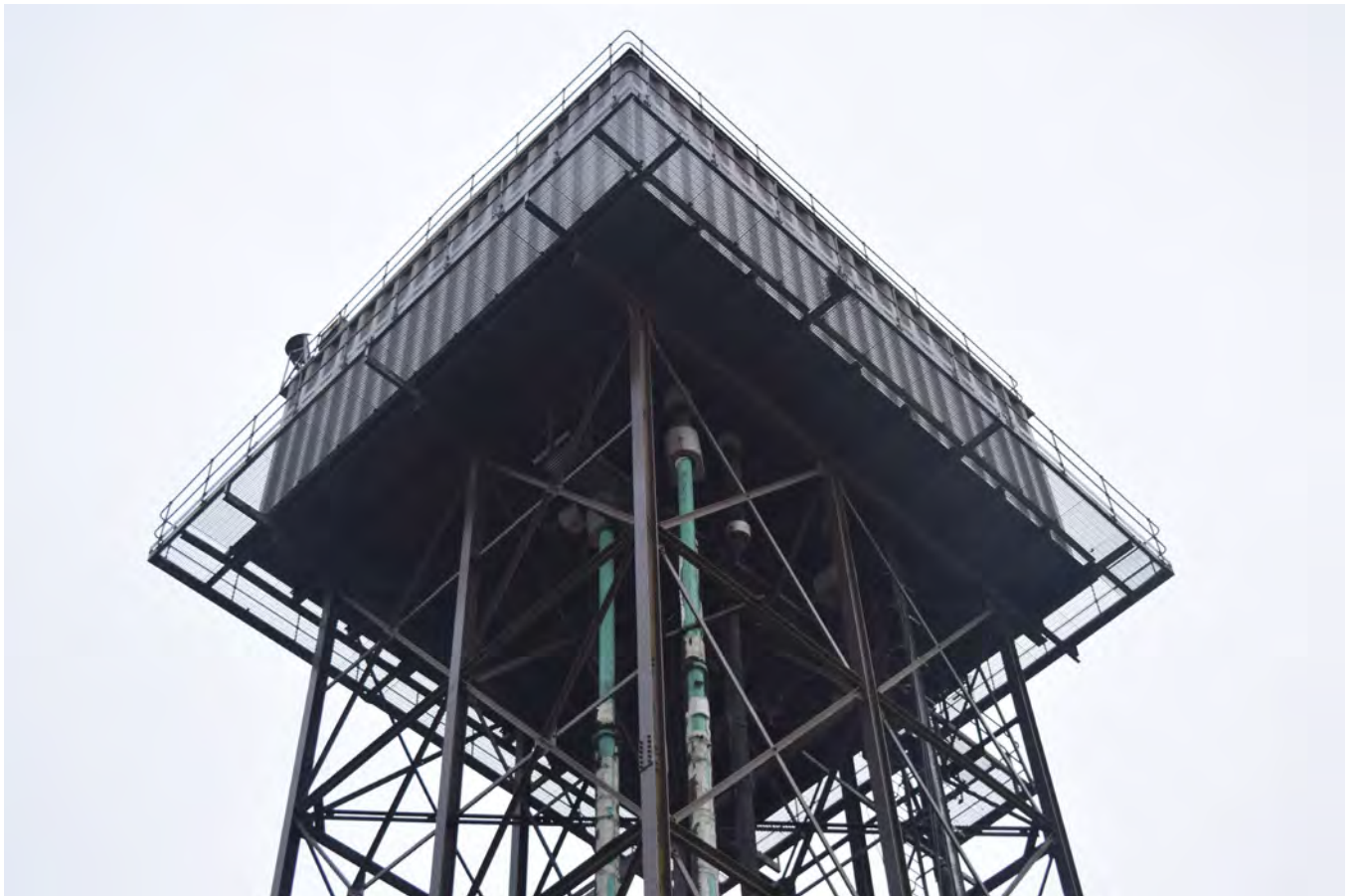
Plate 291.10 Water pipes with lagging
