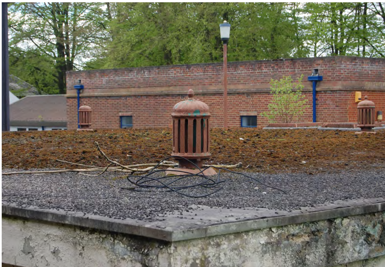
Plate 107.4 Top of tank showing cowels
