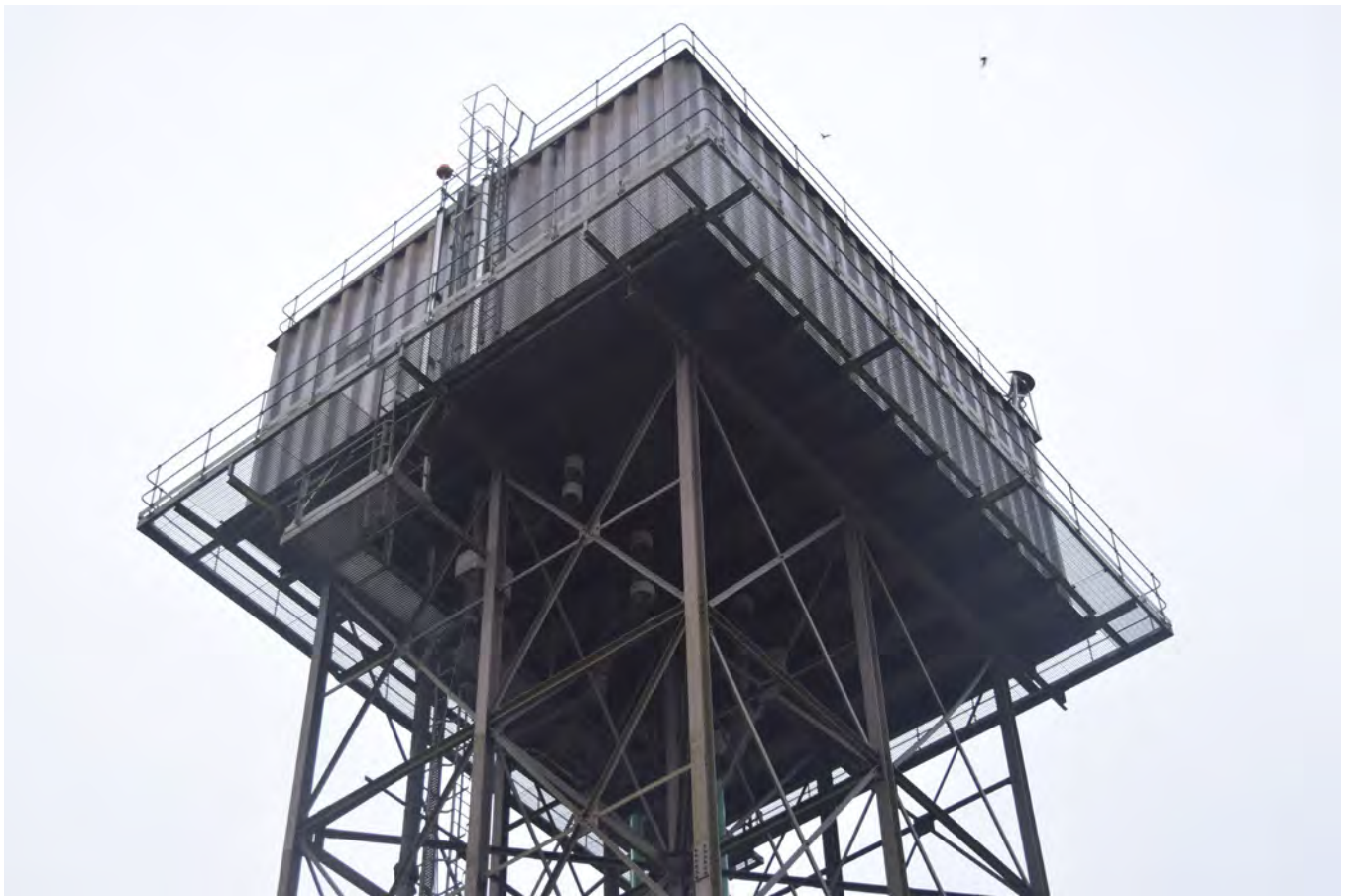
Plate 291.7 Platforms and ladders leading up to the water tank
