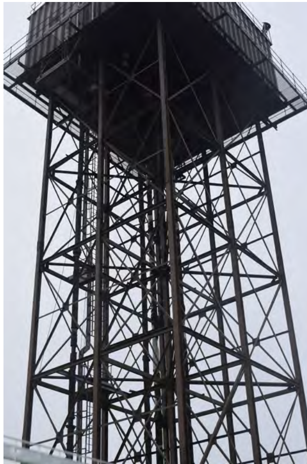
Plate 291.3 Metal frame supporting the water tank
