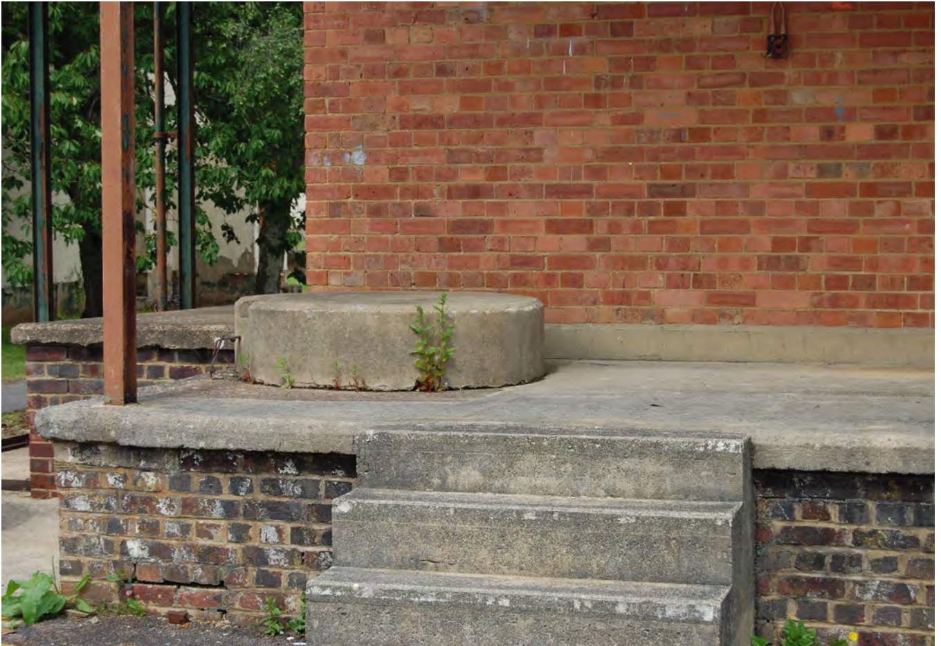
Plate 146.7 Concrete capping to the western corner of the Lubricant Store
