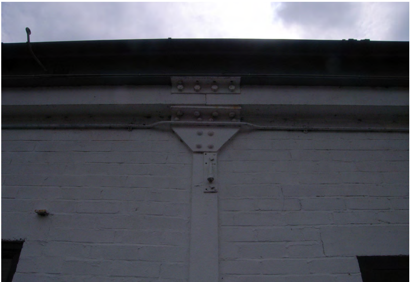
Plate 115.6 An original hinge surviving on a column
