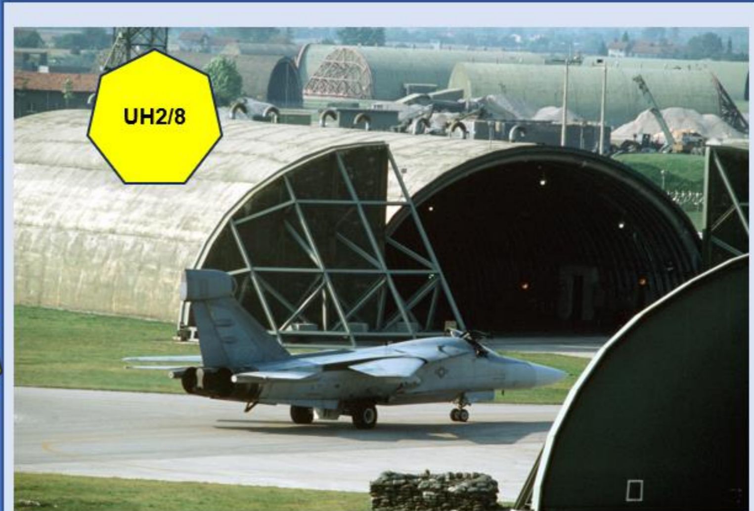
Building 383 was the headquarters of the 42 nd Electronic Combat Squadron. It had an unprotected 'soft' side for everyday use. This 'hard' side was used during alerts. It can withstand a direct hit from a 600 lb (227 kg) bomb. It has a controlled environment. Access was via an Entry Control Point with an armed guard.
