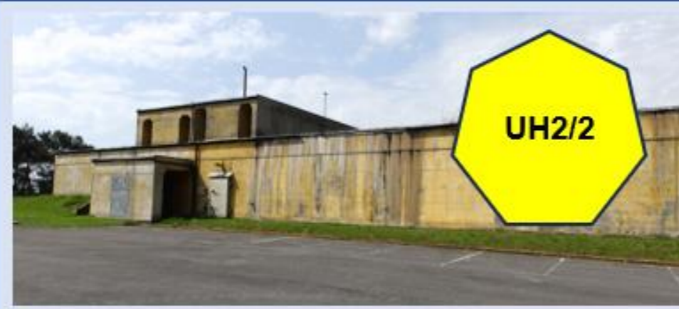
Building 383 was the headquarters of the 42 nd Electronic Combat Squadron. It had an unprotected 'soft' side for everyday use. This 'hard' side was used during alerts. It can withstand a direct hit from a 600 lb (227 kg) bomb. It has a controlled environment. Access was via an Entry Control Point with an armed guard.
