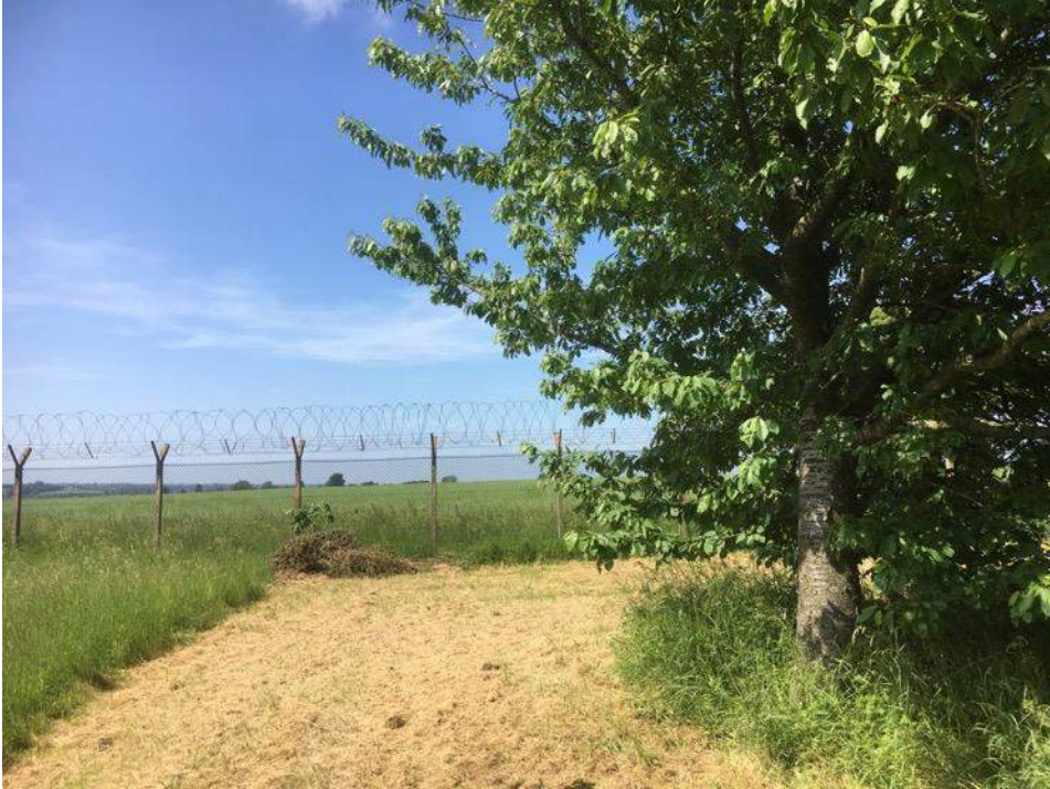
Photoview 2: View looking north towards the existing chain-link perimeter fence with the western edge of G1023 to right of frame.
