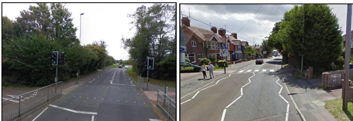
Bucknell Road has footways along both sides of the carriageway, varying in width between 1.2 and 2.0 metres, which is substandard in places. The footways do generally benefit from a good horizontal alignment, street lighting, appropriate crossing infrastructure and a well maintained surface condition.
