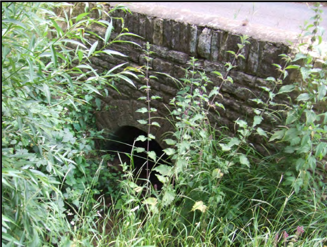
Plate 3: Stone-faced drainage culvert crossing beneath Bucknell Road at a location some 500m NW of the junction (roundabout) with the A4095 (Lord's Lane)
