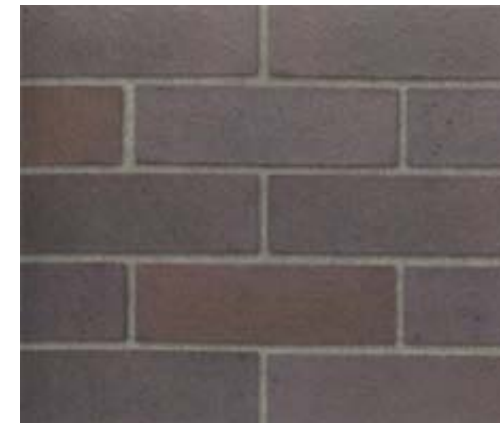
FIG.86 Blue brick, Dragface, Stretcher bond
