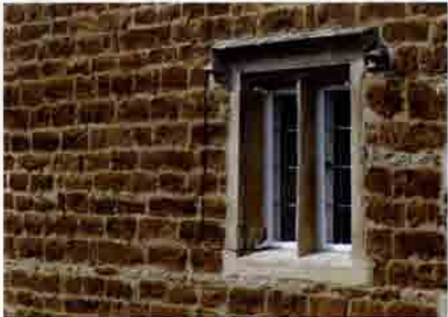
Timber casement window with carved limestone reveal
