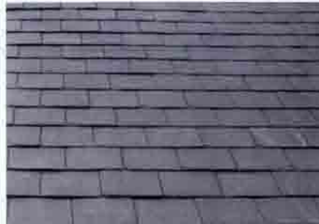
Welsh slate roof
