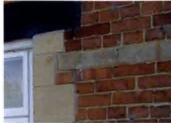
Brick with Limestone Ashlar Dressings
