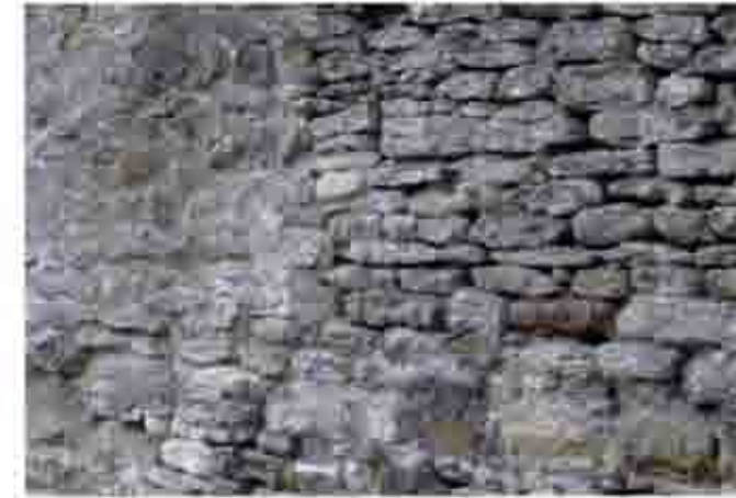
Rubble Limestone of a boundary wall
