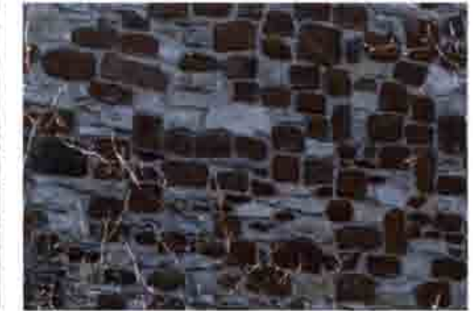
Random mix of ironstone and limestone blocks
