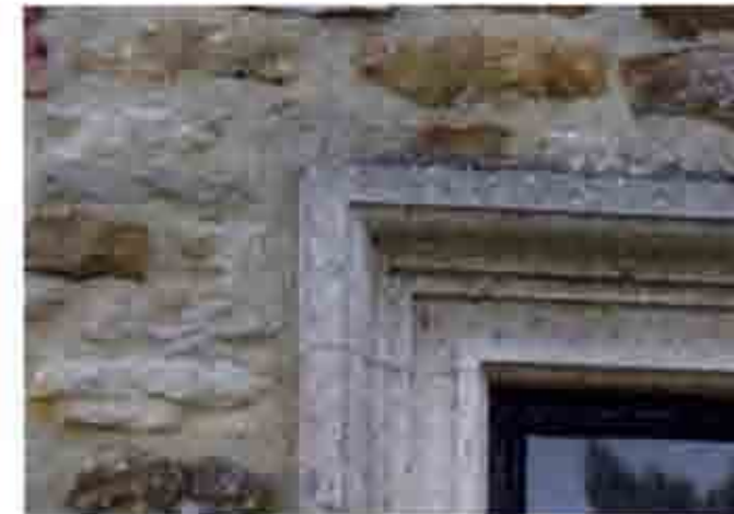
Coarse Limestone stone with Limestone Ashlar Window Reveal
