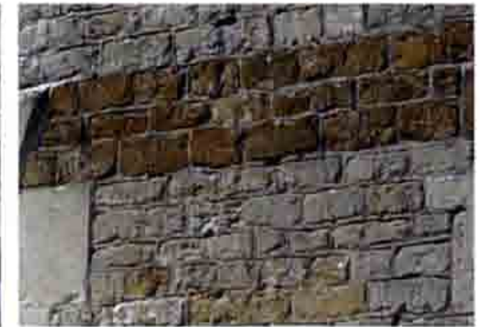
Limestone Blocks with Ironstone Banding
