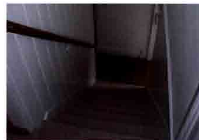
Steep staircase connecting ground and first floor
