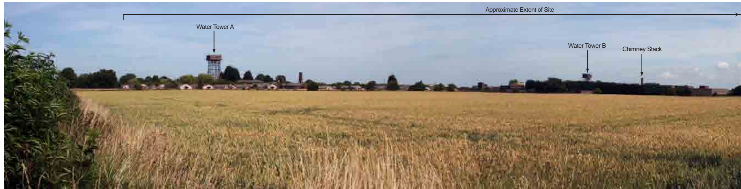
Photoviewpoint 10: View from Kirtlington Road looking east toward the site. The school and recreational sections of the RAF base are visible in the middle ground of the view although other sections tend to merge within the existing vegetation. The water towers act as prominent landmarks for the site.
