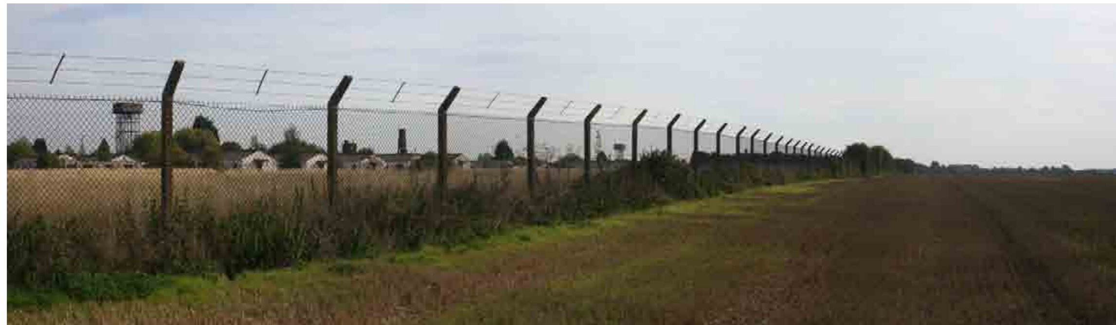
Photoviewpoint 18: View from the footpath at the junction with Kirtlington Road looking east toward the Site. The domineering concrete post and wire mesh fence forms an abrupt and intimidating boundary to the Site whilst the recreational area can also be clearly seen. Other residential areas within the Site are less conspicuous. Views further into the Site are not possible.
