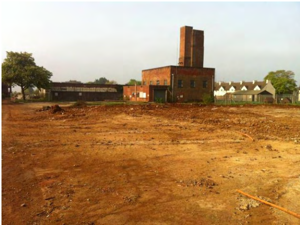
30.04.14 Southern view of building 467 (boiler house); location of UG-NSA 1-3
