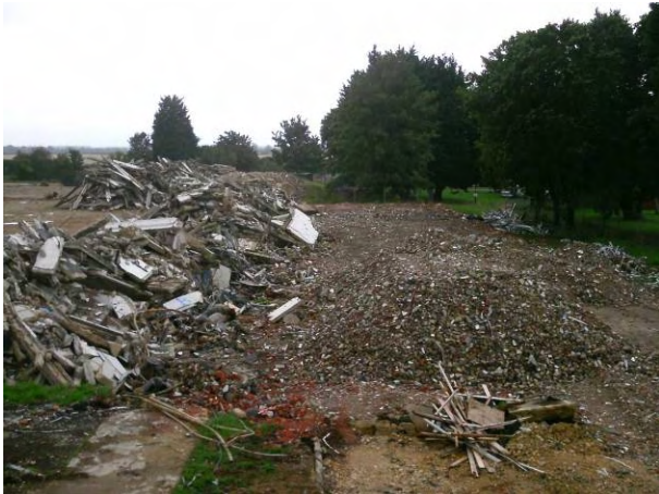
26.06.14 Demolition material awaiting processing from buildings 594 and 598
