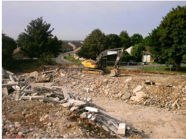
10.09.14 Removal of foundations/obstructions associated with building 598
