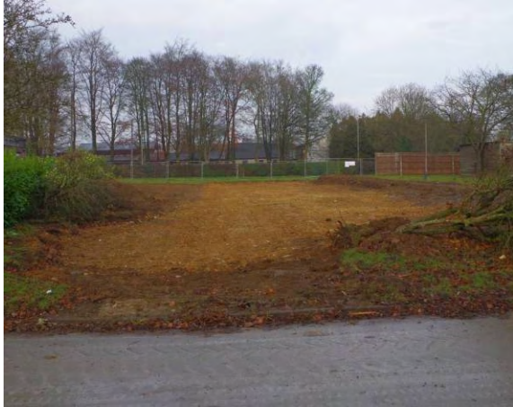
05.12.13 Earthworks complete in location of former building 459
