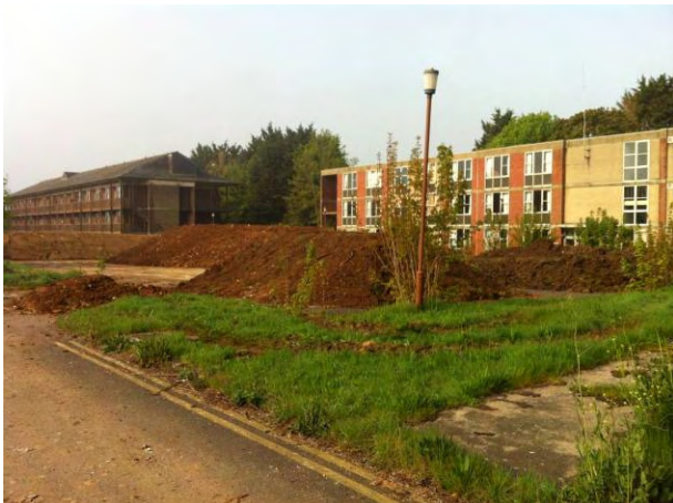
30.04.14 South-west corner of the site, barracks buildings 594 (right) and 598 (left) visible
