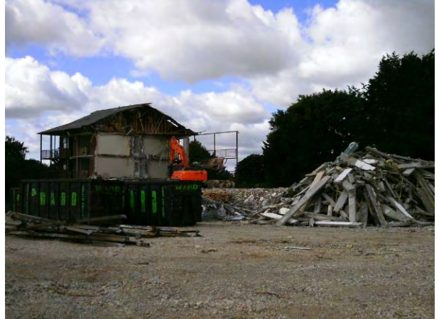
19.08.14 Demolition of former barracks (building 598) taking place in the south-west corner
