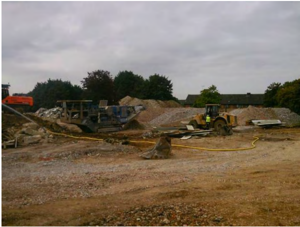
10.09.14 Processing site won aggregate (Agg-W); dust suppression in use
