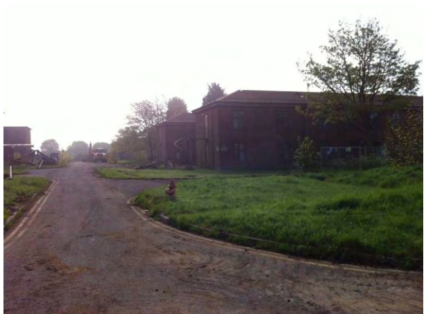
30.04.14 Southern view of the site prior to demolition
