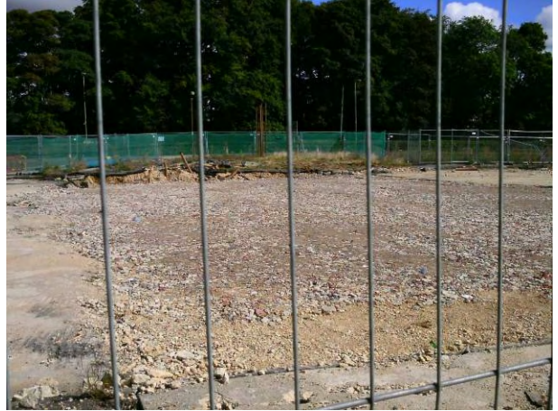
19.08.14 Backfilled area following remediation of UG-NSA- 16-20
