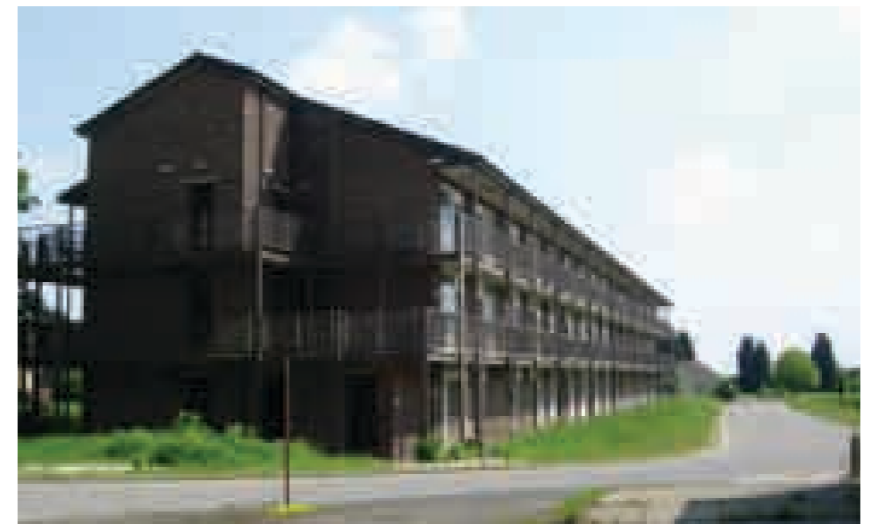
Barracks (RAF Domestic and Residential Section)
