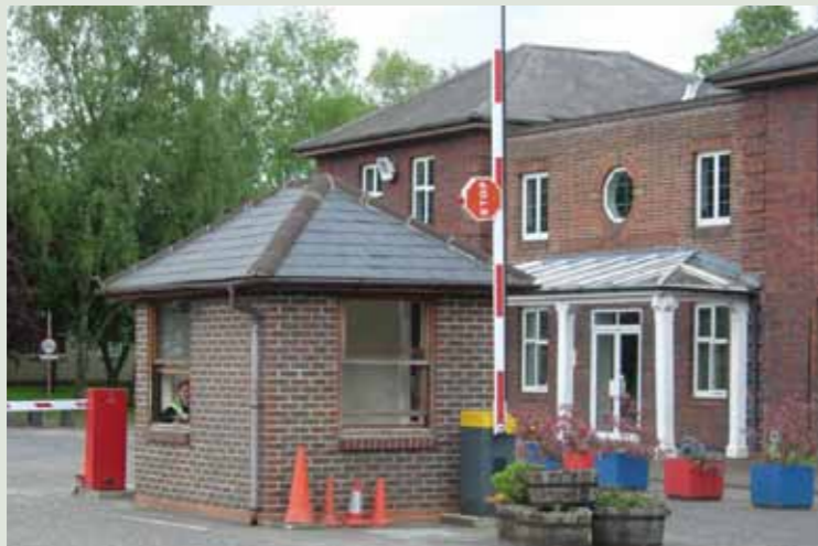
BRICK AND SLATE ROOFING
