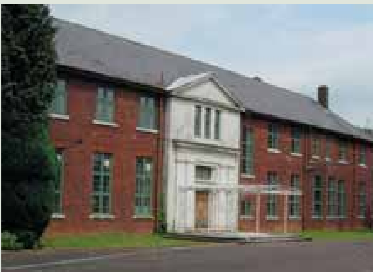
RED BRICK, SLATE ROOF FEATURE RENDERED GABLE
