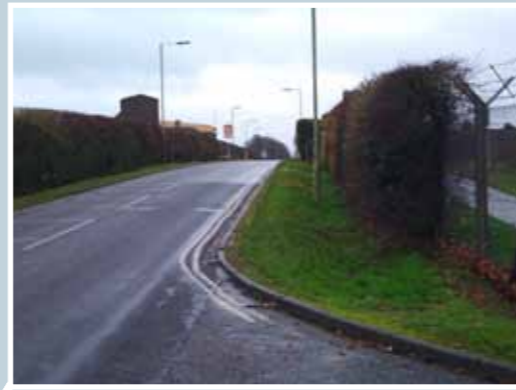
EXISTING HEDGEROW SCREENS SECURE FENCING TO NORTH OF CAMP ROAD.
