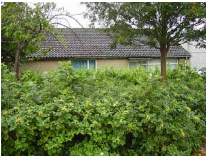
BUILDING 650 TO BE RETAINED
