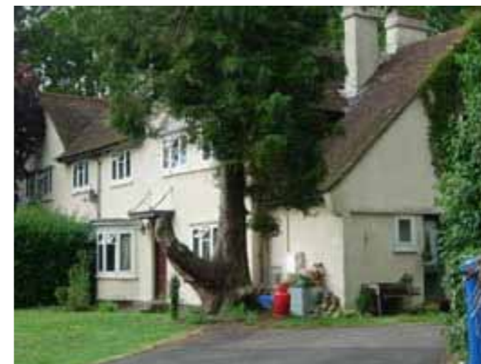
BUILDING 1 TO BE RETAINED
