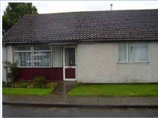
EXISTING BUNGALOWS DOMINATE THE MIDDLE OF THE SOUTHERN AREA.
