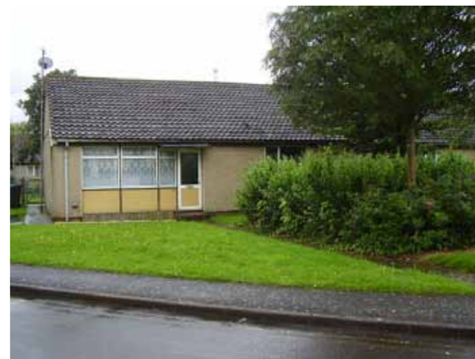
BUILDING 650 TO BE RETAINED
