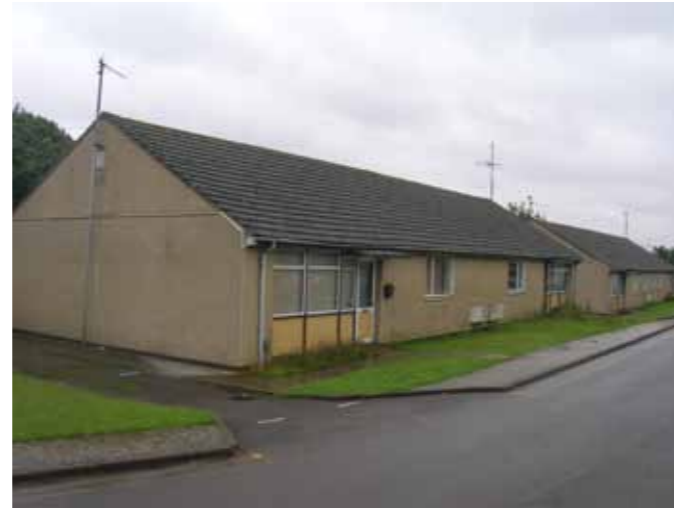
BUILDING 716 TO BE RETAINED
