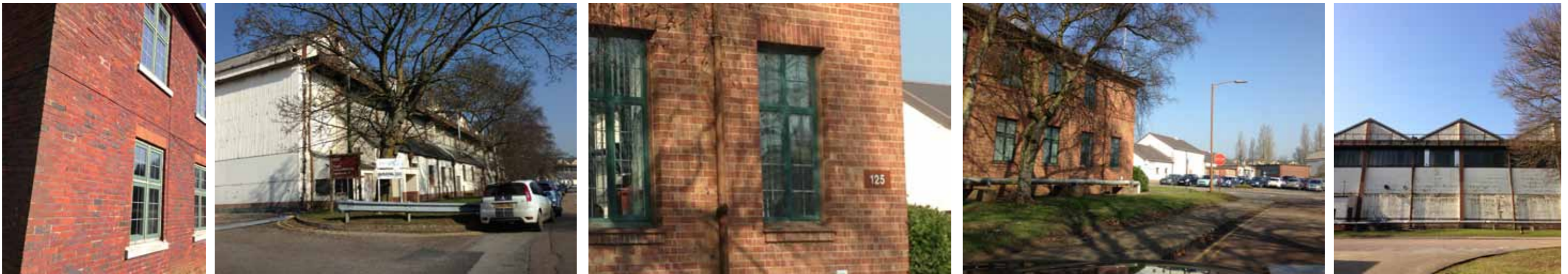
EXISTING TRIDENT AREA BUILDINGS
