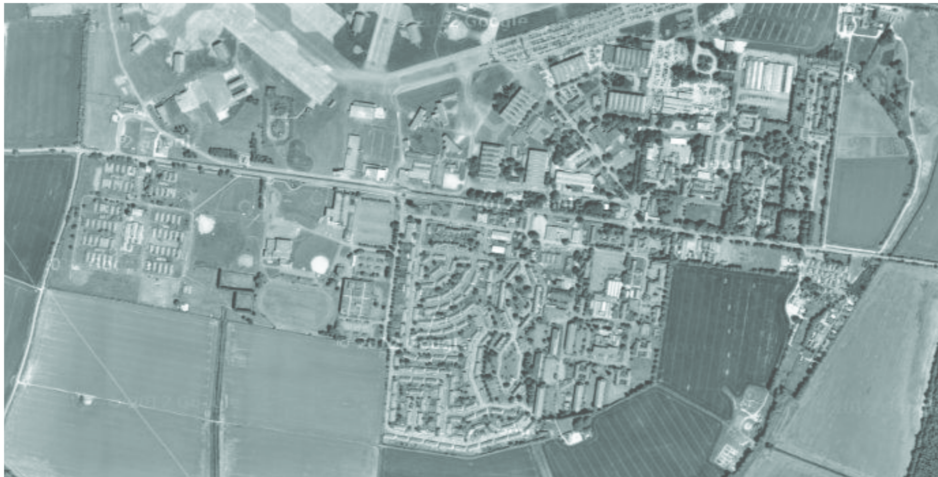
AERIAL PHOTOGRAPH OF SITE
