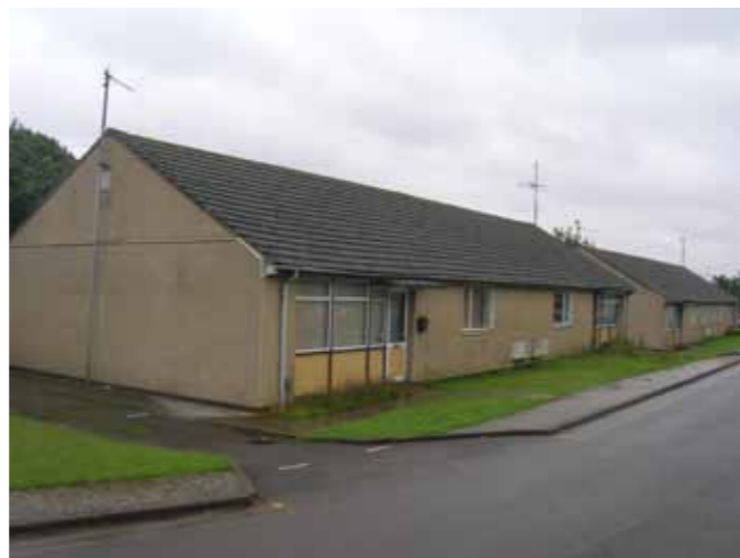
BUILDING 716 TO BE RETAINED
