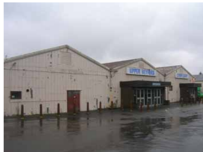
BUILDINGS 32 & 34 TO BE REMOVED
