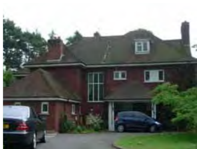
BUILDING 2 TO BE RETAINED
