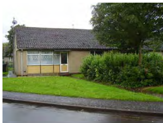
BUILDING 650 TO BE RETAINED
