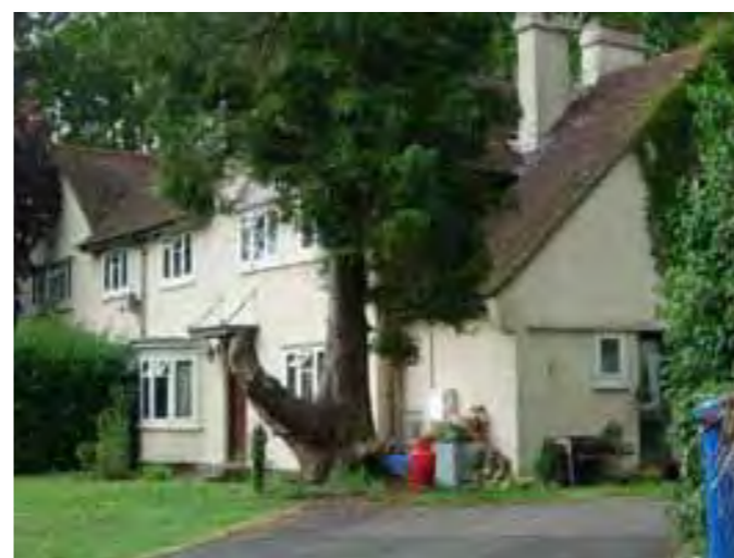
BUILDING 1 TO BE RETAINED
