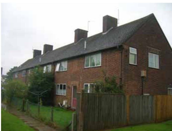
BUILDING 533 TO BE RETAINED
