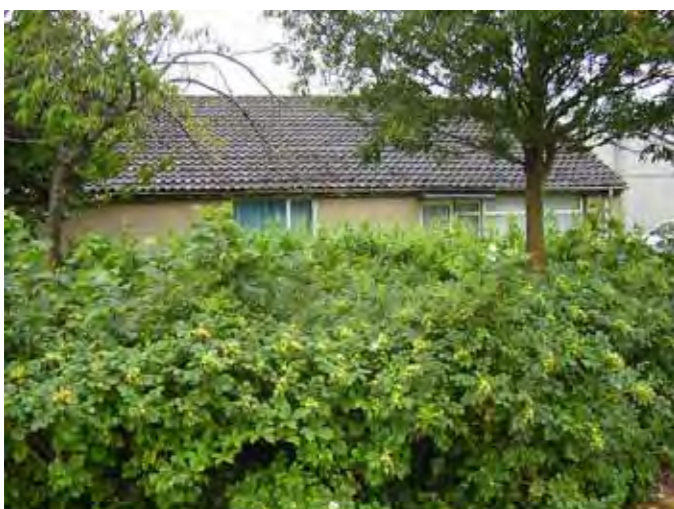
BUILDING 650 TO BE RETAINED
