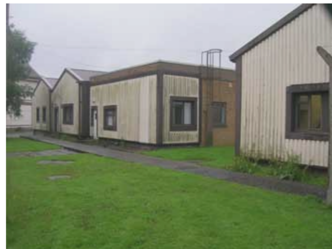
BUILDING 123 TO BE REMOVED
