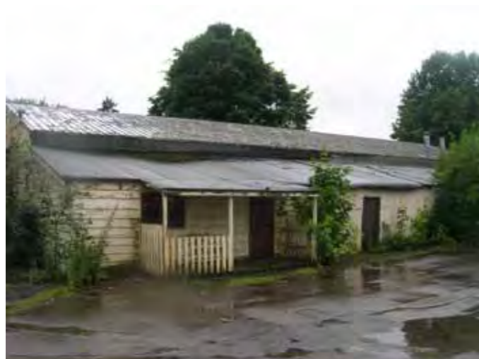
BUILDING 313 TO BE REMOVED
