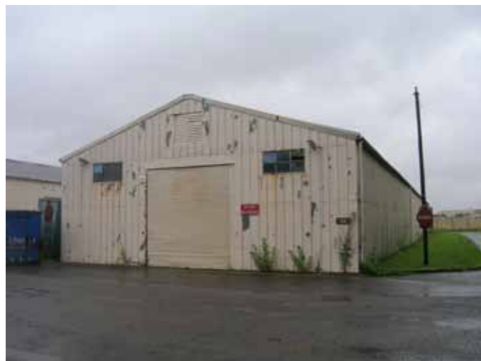
BUILDING 35 TO BE REMOVED
