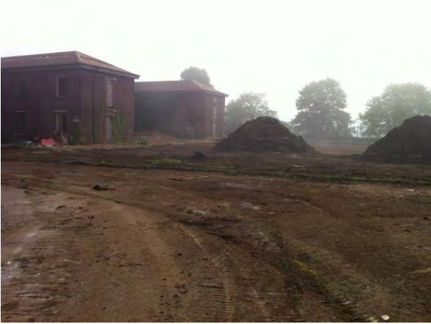
30.04.14 Strip of area of soft-landscaping prior to demolition works taking place
