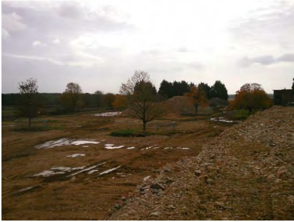
22.10.14 Southern view from the top of D1B-Agg-NE stockpile
