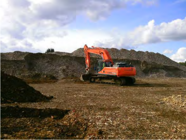
07.10.14 Stockpile of approximately 4000m 3 aggregate (Agg-D1b-NE)
