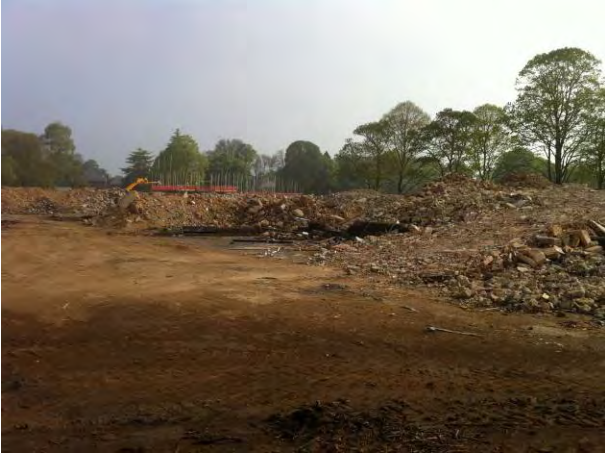
30.04.14 Buildings demolished in the north, awaiting processing of recovered aggregates/hard-standing
