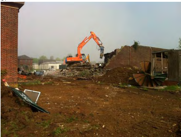
30.04.14 Demolition of building 443 (Store) taking place
