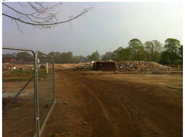
30.04.14 Northern view with Building 476 (sub-station remaining)
