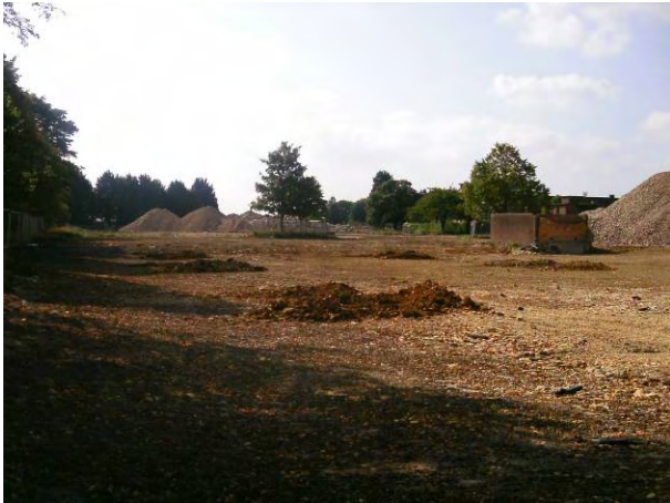
10.09.14 Southern view of the site showing the location of D1B-SS6 re-sampling entries
