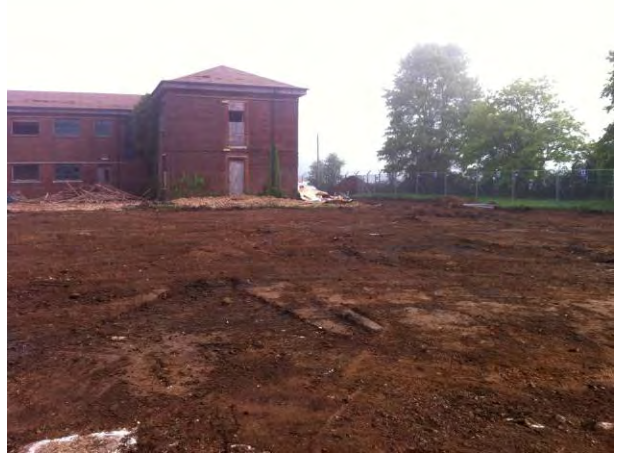
30.04.14 Southern area of the Phase D1B: Area 1
