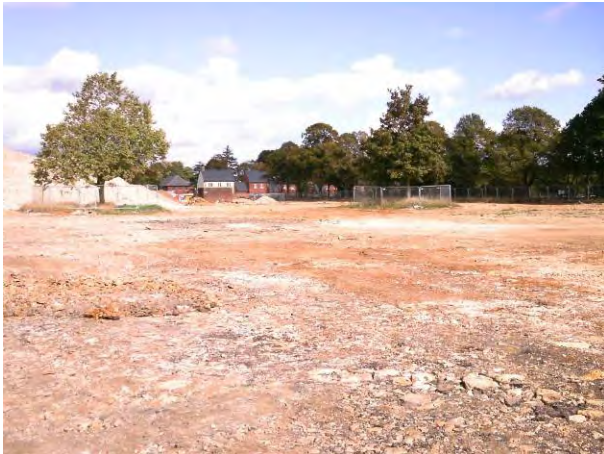
24.09.14 North-east view of the Phase 1B: Area 1
