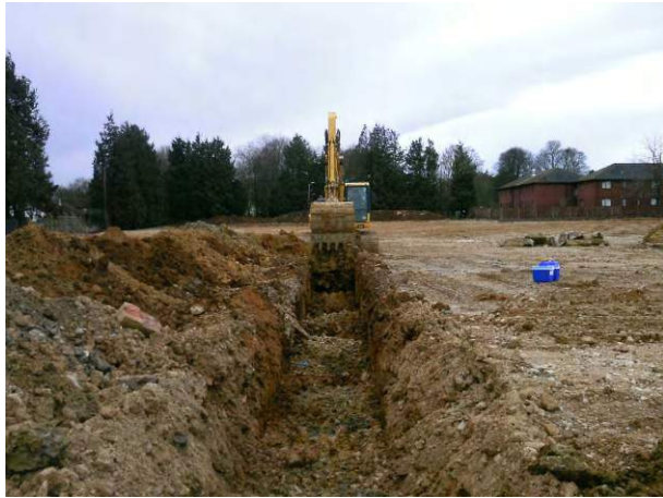
23.02.15 Excavation of trench (north to south) in north-east of Phase D2
