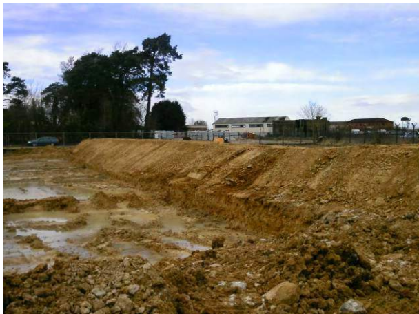
23.02.15 Clean overburden batoned in order to reduce water percolation during removal
