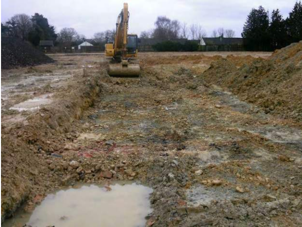
16.02.15 Exposed contaminated soils awaiting removal
