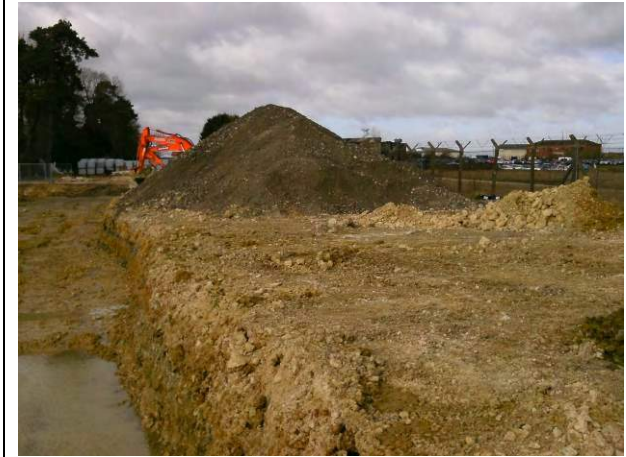
04.03.15 – Remaining area awaiting hydrocarbon removal
