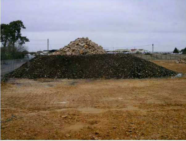
13.01.15 Stockpile of site won "tarmac" stripped from former car park areas
