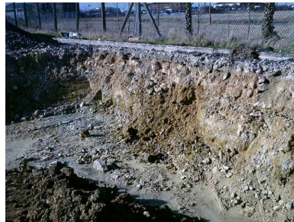
10.03.15 – Hydrocarbon contamination removed down to solid bedrock
