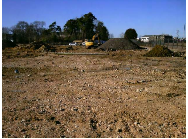
17.02.15 Natural strata exposed at site surface following removal of hard-standing
