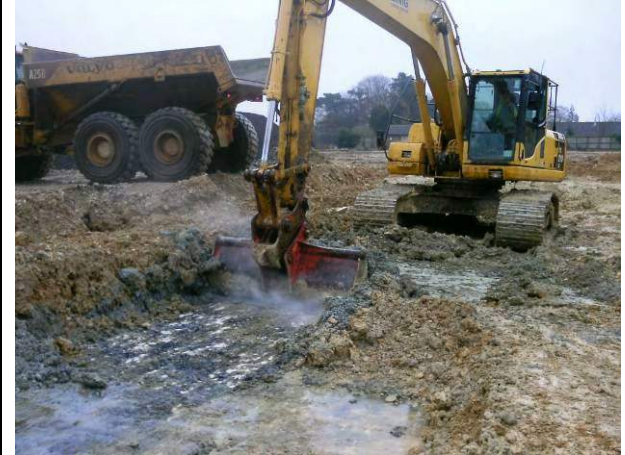
16.02.15 Removal of impacted soils to treatment/storage area
