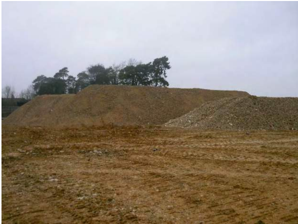
16.02.15 Aggregate stockpile (Agg-1) located in the west of the site
