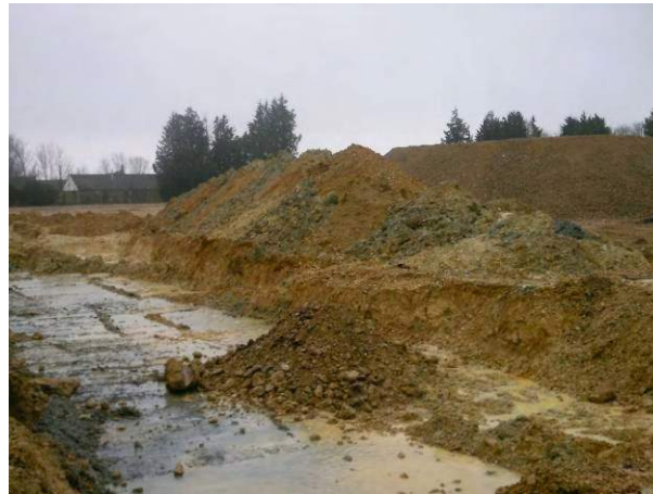
16.02.15 Clean soils side cast pending replacement following contamination removal
