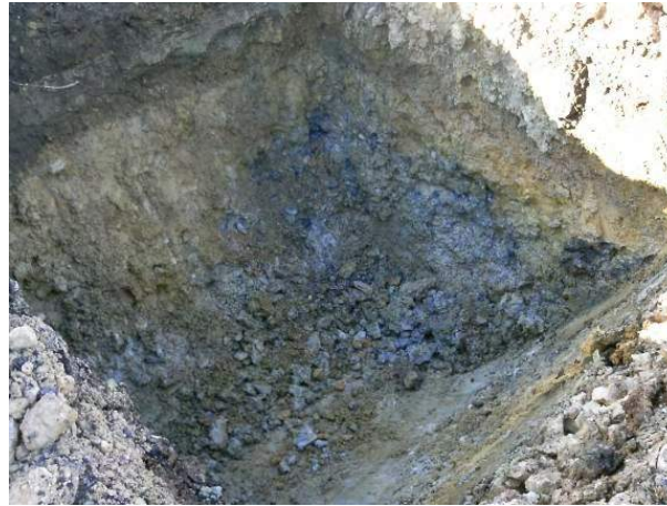
17.02.15 Grey/Silver impacted soil at base of trial-pit confirms hydrocarbon impacted soil present
