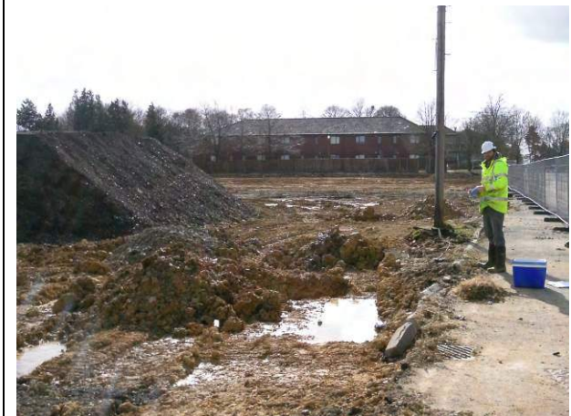
04.03.15 – Collection of validation samples along the western boundary following removal
