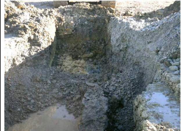
19.01.15 Extent of URL HS1 removal confirmed and validation sample collected from north and southern extent
