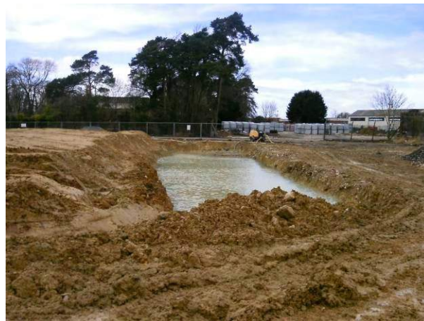
23.02.15 Adjacent remediation cell requiring pumping following ingress of groundwater
