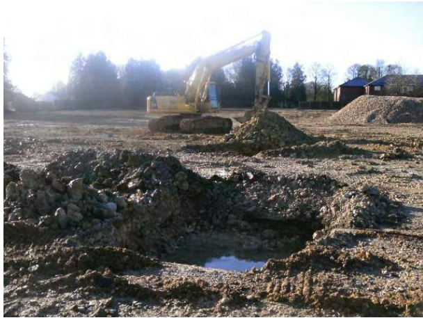
17.02.15 Excavation of trial-pits to delineate the extent of hydrocarbon impacted soils
