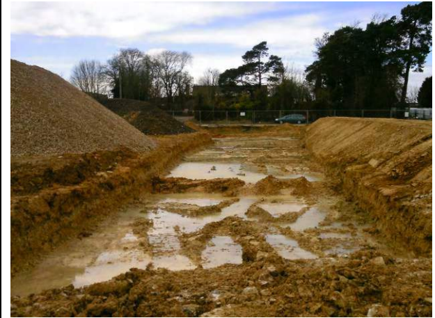
23.02.15 Side cast over burden to expose soils ~0.5m above bedrock to allow SGP screen with PID
