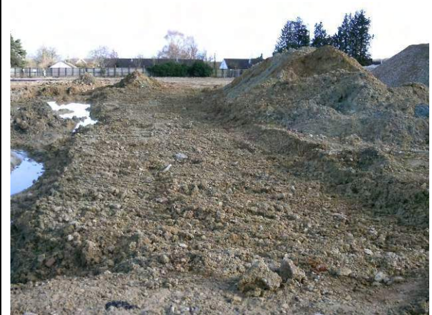
17.02.15 Backfill of excavation area with clean uncontaminated soil
