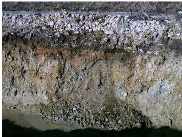
10.03.15 – Excavation sidewall available for inspection and collection of validation samples
