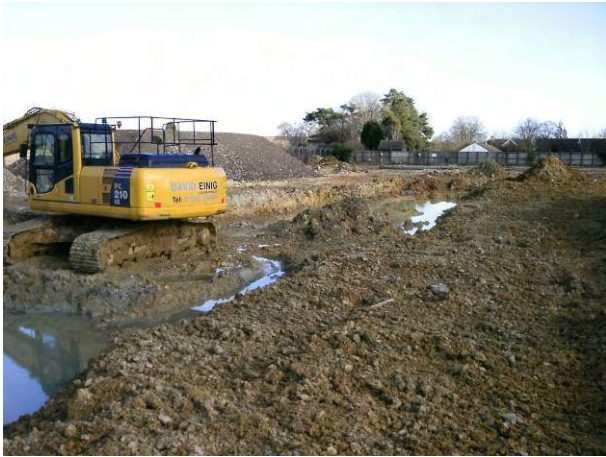
17.02.15 Excavation of hydrocarbon impacted soils in the north-east of the site
