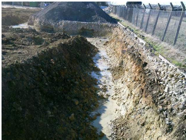
10.03.15 – Removal of contamination up to northern boundary
