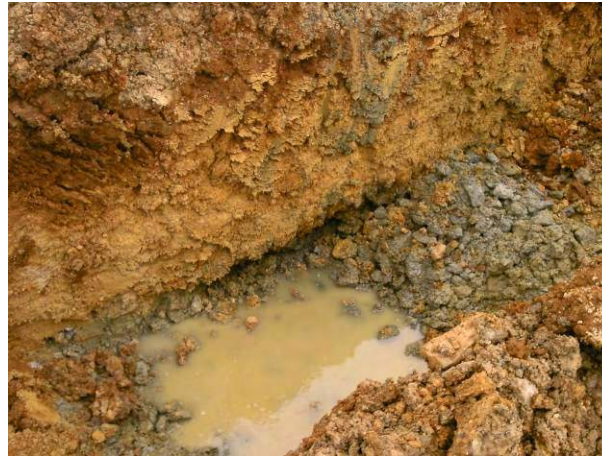
23.02.15 Grey hydrocarbon impacted soils encountered (150ppm)
