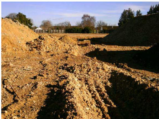
17.02.15 Trench from western boundary into site centre
