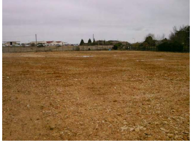
13.01.15 Centre of the site, natural soils of weathered limestone bedrock visible
