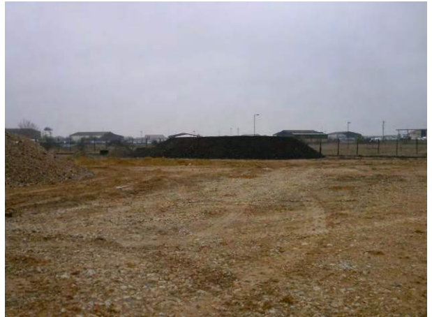
16.02.15 Stockpile of site won tarmac located in the north-west
