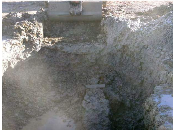
19.01.15 Continuation of trench 1 (north to south) until granular infill no longer encountered and natural strata remains
