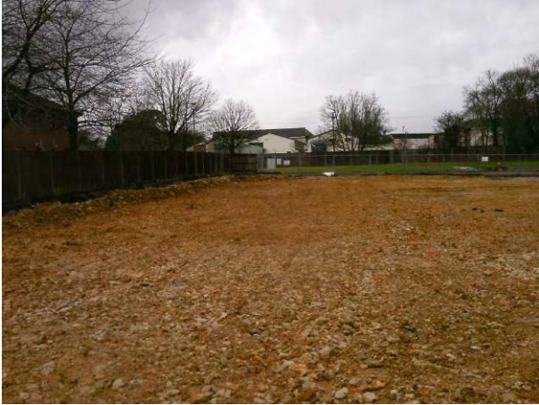
13.01.15 Western view along the site's southern boundary
