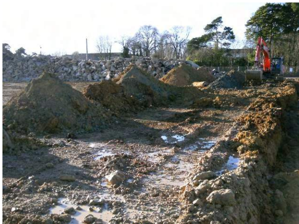
19.01.15 Arisings screened with a PID, maximum reading of 100ppm
