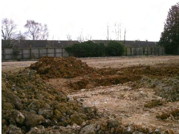
04.03.15 – Excavation of trial-pits to delineate extent of contamination in the north-west
