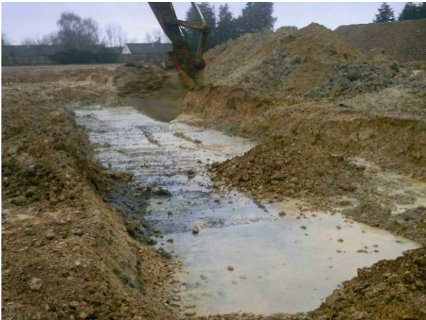
16.02.15 Clean soils side cast, contaminated soil removed down to bedrock
