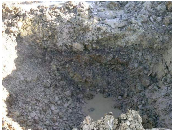
19.01.15 Trench 2 excavated (east to west)
