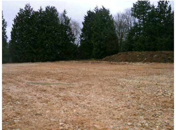
13.01.15 South-east corner of the site, soil mound (background) denotes area not remediated due to trees
