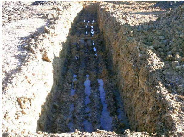
19.01.15 Trench 3 excavated to confirm presence of hydrocarbon contamination
