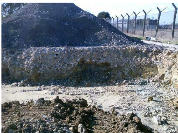
10.03.15 – Lateral extent of excavation
