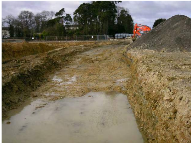
04.03.15 – Contamination removed from remediation cell down to bedrock, validation samples collected
