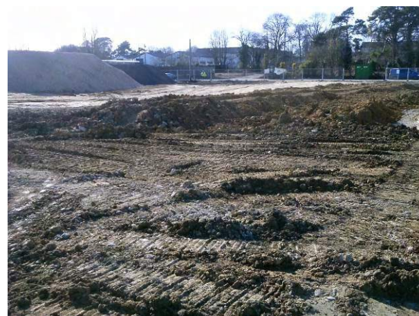
10.03.15 – Clean overburden replaced in adjacent remedial cell
