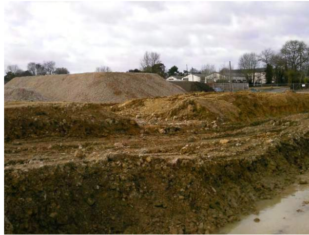
04.03.15 – Clean overburden side cast from remediation cell during contamination removal
