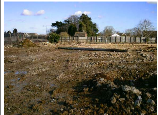
17.02.15 Trial-pits within north-east corner of the site
