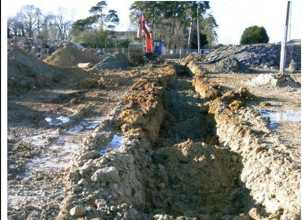
19.01.15 Trench 3 extended (east to west) to delineate extent of contamination
