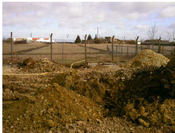
04.03.15 - Excavation of trial-pits to delineate extent of contamination in the north
