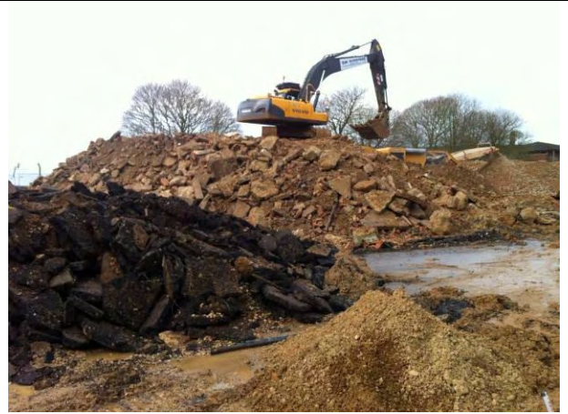
28. 17.01.14 – Site generated recycled aggregate
