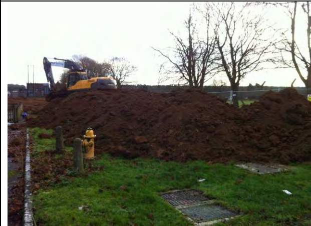
5. 18.12.13 – Phase 1A site generated topsoil
