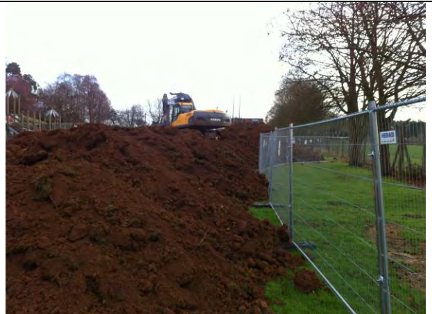
6. 18.12.13 – Phase 1A site generated topsoil
