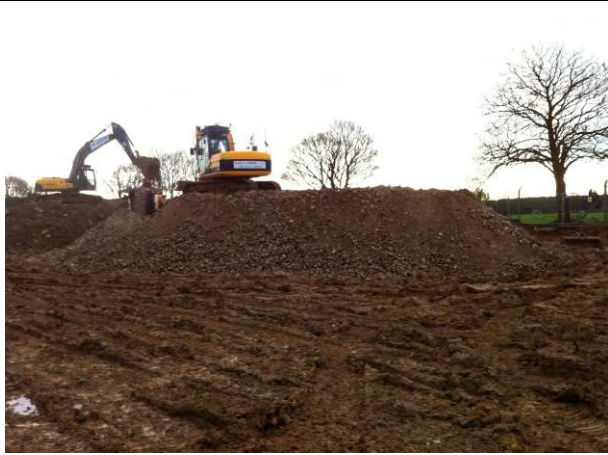
27. 17.01.14 – Site generated recycled aggregate
