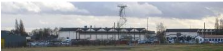
Type A Hanger and observation tower
