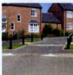
Fig.69. Raised pedestrian crossing.
