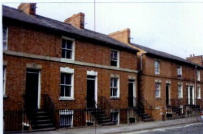
Fig. 12: Typical stringcourse features on workers cottage.
