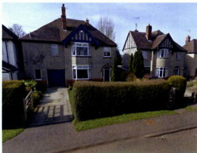
Fig. 19: Post Second World War detached house with bay windows, timber gables and hip roofs
