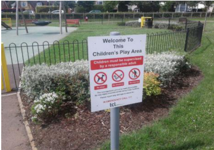
Finding: Sign loose
