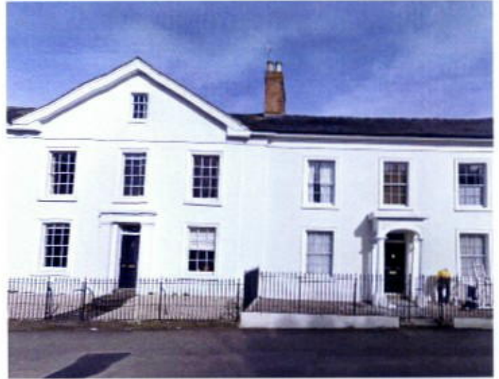
Fig. 18: Simple proportioned houses with stucco 'render' and vertically balanced sash windows, typical classical architecture features.
