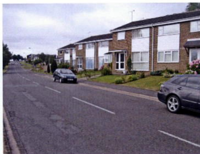
Fig 24: White fascia board is a key feature of properties on Cherwell Heights
