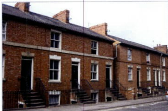
Fig. 12: Typical stringcourse features on workers cottage.
