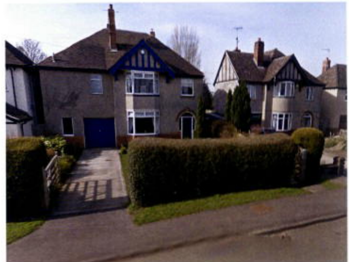
Fig. 19: Post Second World War detached house with bay windows, timber gables and hip roofs
