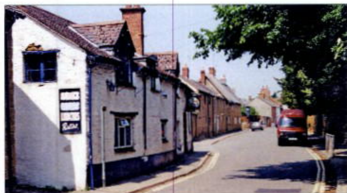
Fig 31: A small amount of the buildings are whitewashed, which is in contrast to the local vernacular of honey coloured ironstone.
