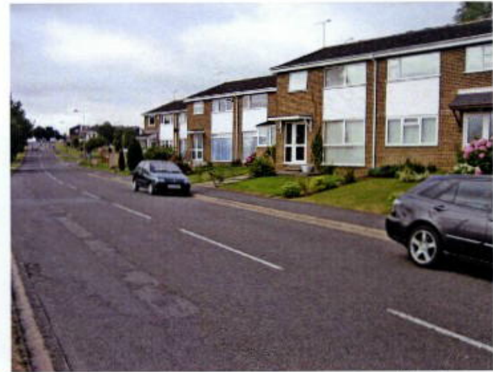
Fig. 24: White fascia board is a key feature of properties on Cherwell Heights
