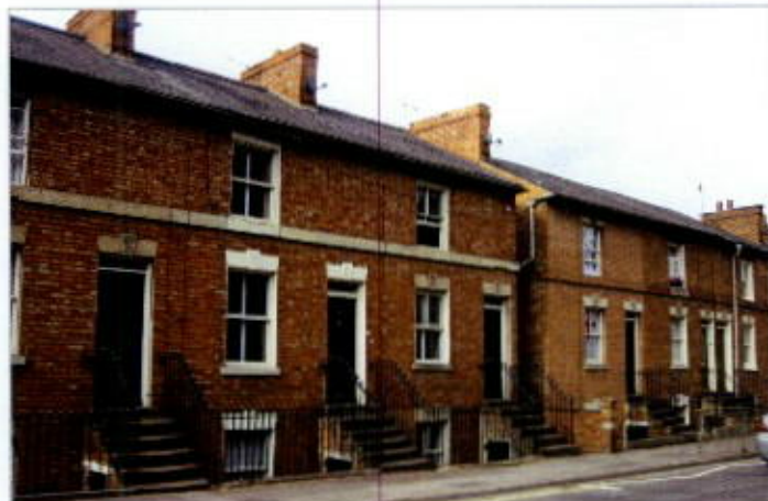
Fig 12: Typical stringcourse features on workers cottage.
