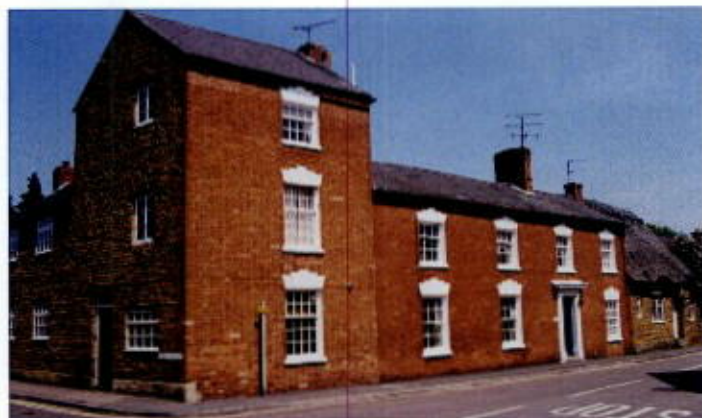
Fig 29: There are a diverse range of storey heights within Bodicote, with the higher storeys at the corner of the blocks. The range of materials used on the corner building adds interest to the streetscape
