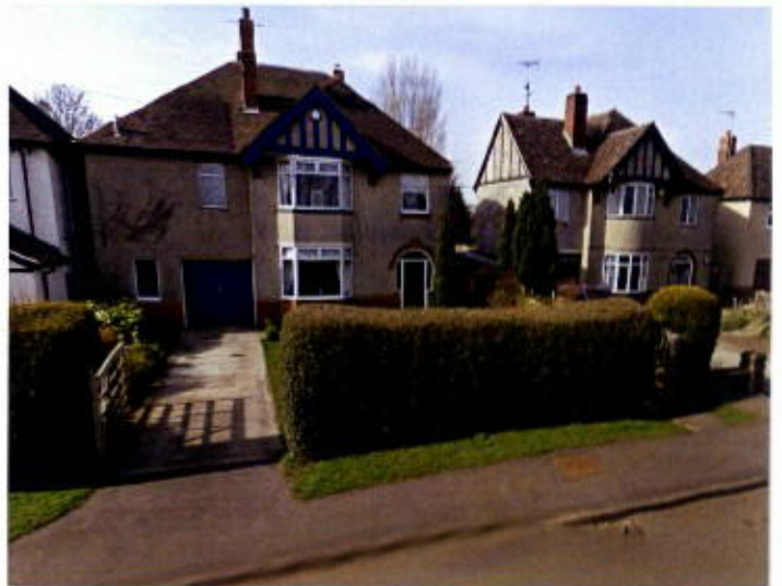
Fig. 19: Post Second World War detached house with bay windows, timber gables and hip roofs
