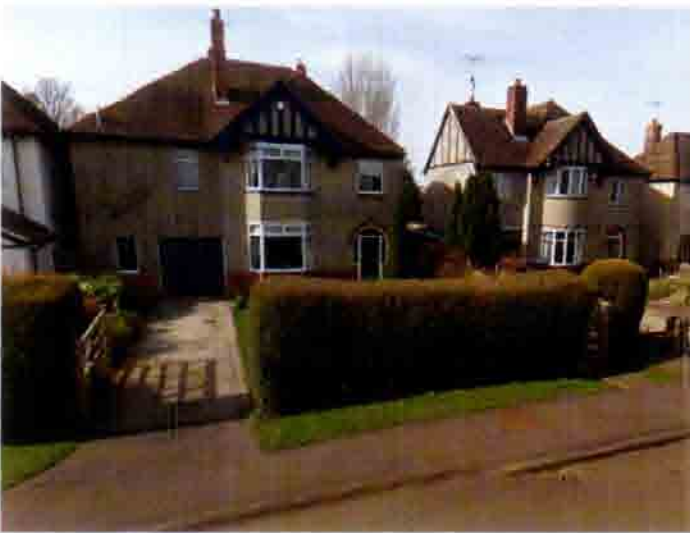
Fig. 20: Post Second World War detached house with bay windows, timber gables and hip roofs
