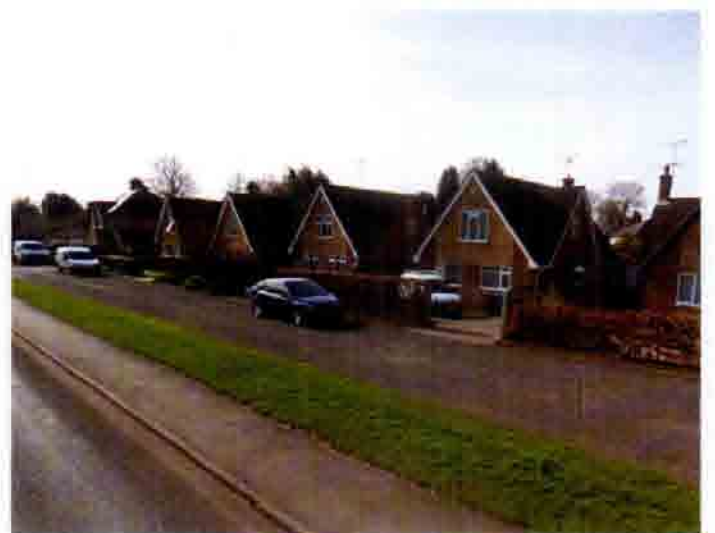
Fig.23 1960-70's suburban detached houses of one and a half storey in height and a variety of pale orange and ochre bricks.
