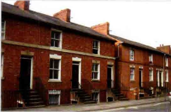
Fig.12: Typical stringcourse features on workers cottage.
