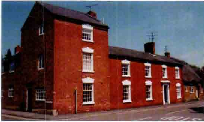
Fig.28: There are a diverse range of storey heights within Bodicote, with the higher storeys at the corner of the blocks. The range of materials used on the corner building adds interest to the streetscape.
