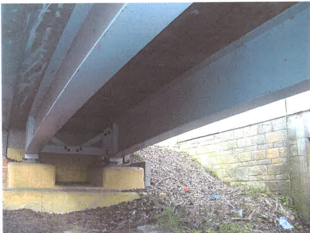
Photograph 2: Underside of Footbridge on downstream side of Charbridge Lane Bridge
