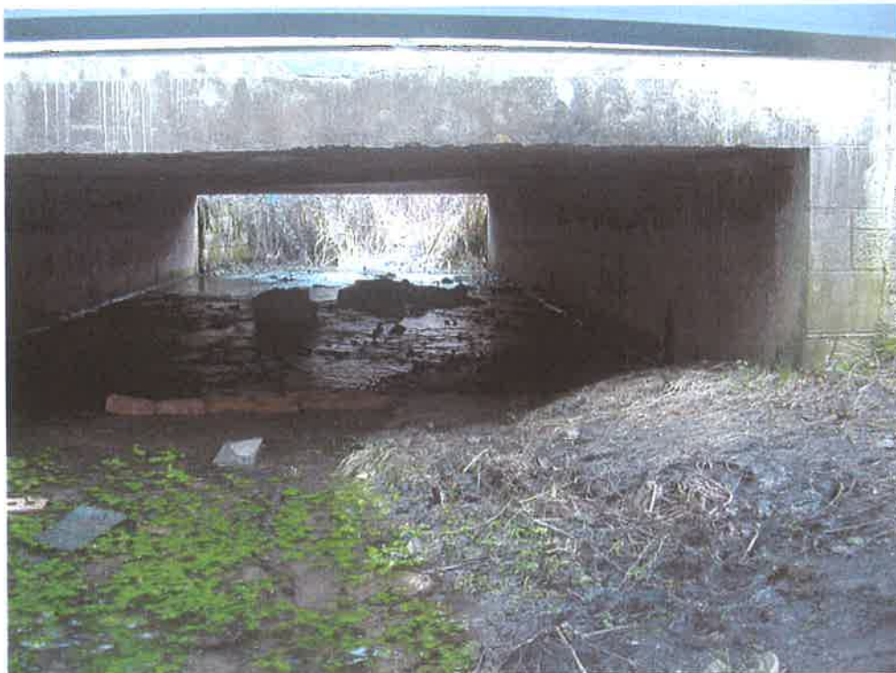
Photograph 4: Culvert under Charbridge Lane
