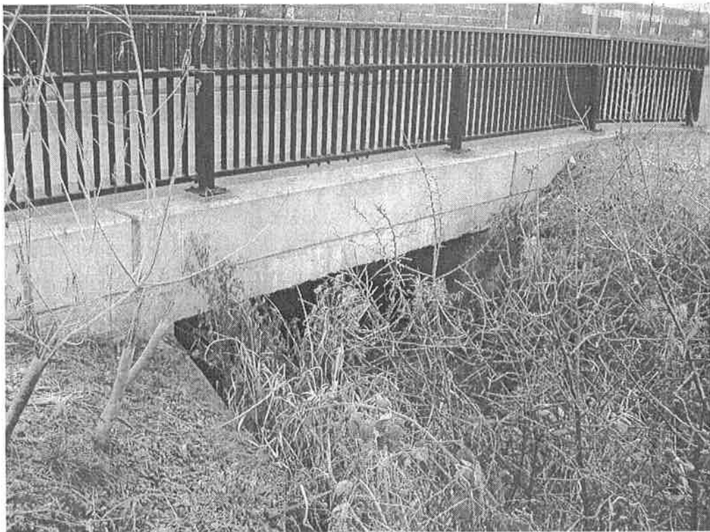
Photo 1 – Skimmingdish Lane Brook – Typical cross-section
