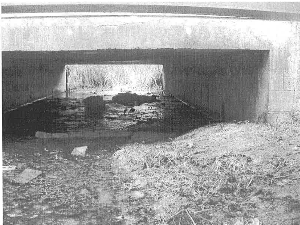
Photo 1 – Skimmingdish Lane Brook – Culvert
