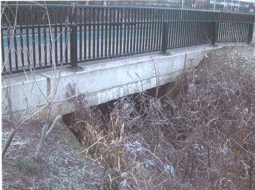
Photograph 1: Looking downstream at Charbridge Lane Bridge
